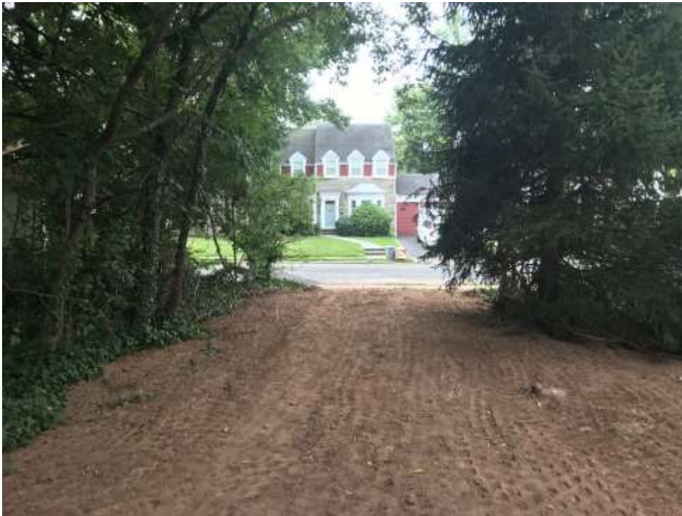
Pathway area prep work underway– Clinton Elementary School
