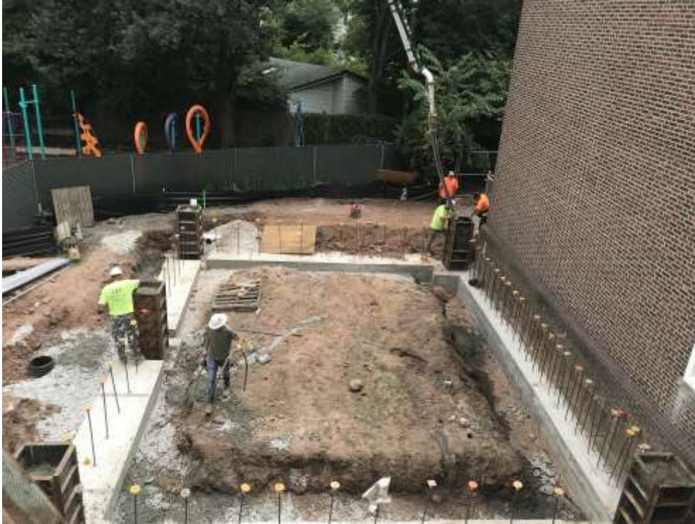
Pouring Piers at Addition C– Clinton Elementary School
