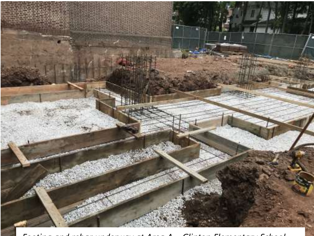
Footing and rebar underway at Area A – Clinton Elementary School
