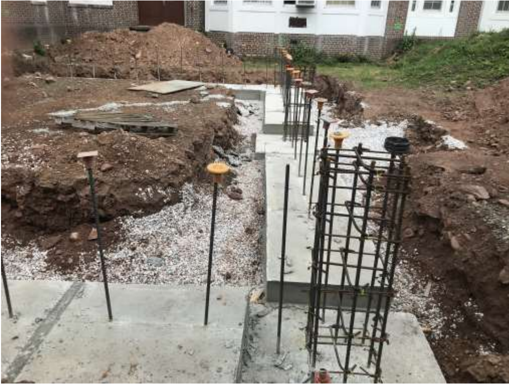
Footing and rebar completed at Area C – Clinton Elementary School
