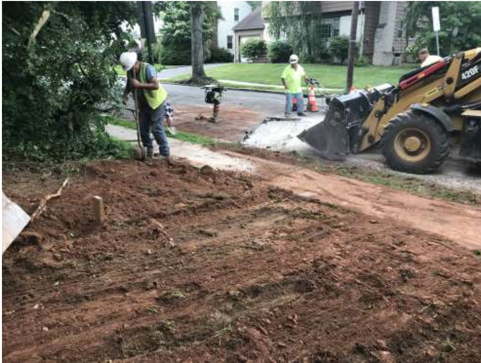
Storm tie-in connection– Clinton Elementary School
