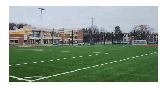
Installation of the artificial turf field has been completed, including the grooming of the in-fill material, game lines and soccer goals. The new flagpole has been installed, and the installation of the chain-link fence and netting posts is nearing completion. MUSCO sports lights have been energized. Fine grading on the north and south sides of the artificial turf field has been delayed due to recent rain and overnight freezing temperatures.
