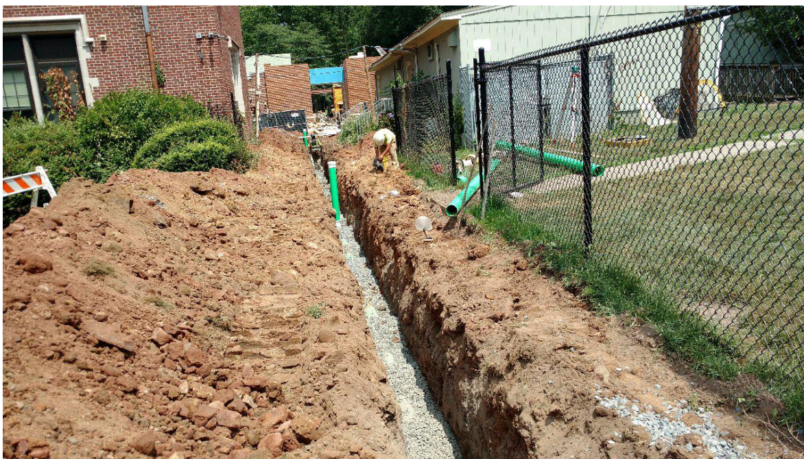
Tuscan School- Sanitary Pipe Installation
