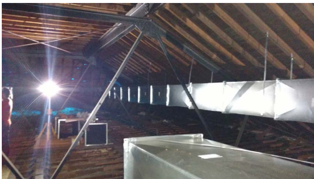
Seth Boyden School- Auditorium Duct Installation at Attic
