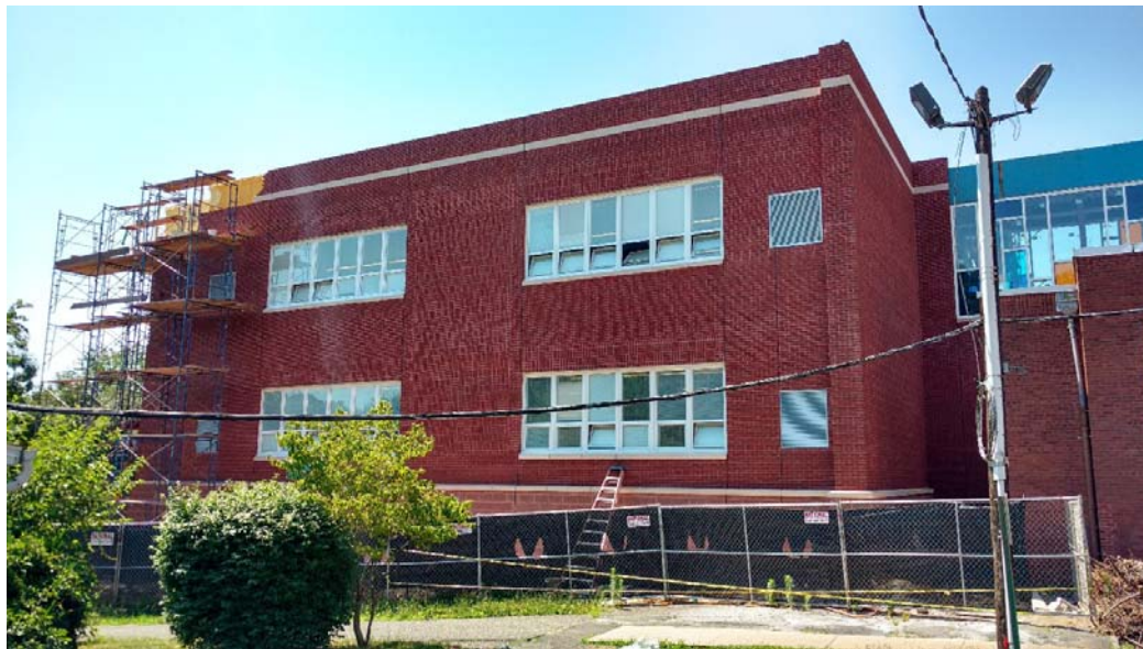
Seth Boyden School- South Building Elevation
