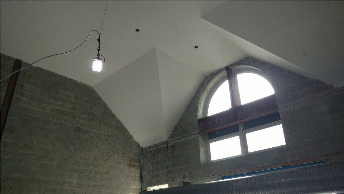
Tuscan School- Painted Classroom Ceiling
