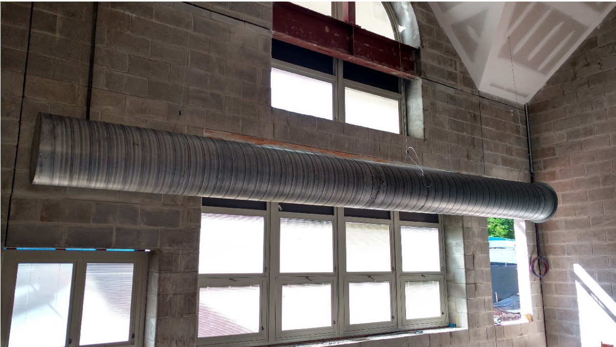
Tuscan School- Rough Elevation of Metal Ductwork at New Classroom
