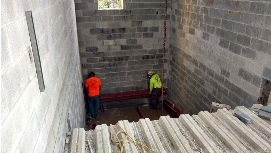
Seth Boyden School- Stair Tower Steel Installation
