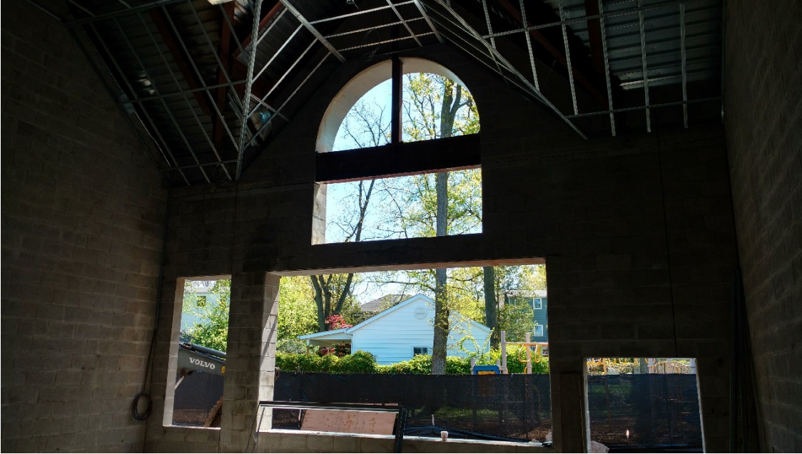
Tuscan School- Classroom Window wall
