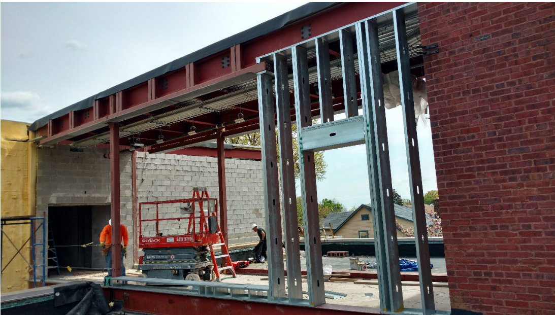
Seth Boyden School - Skywalk Metal Framing
