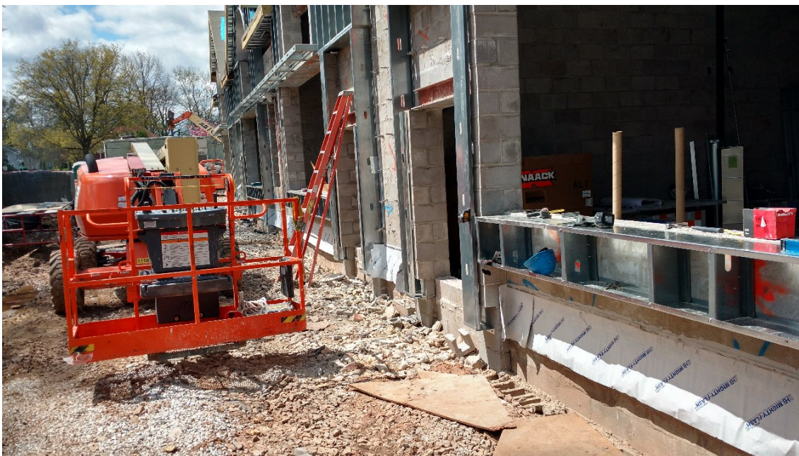
Tuscan School – East Exterior Window Wall Framing
