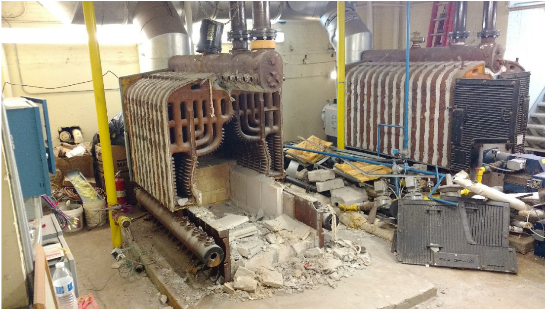
Tuscan School– Existing Boiler Demolition
