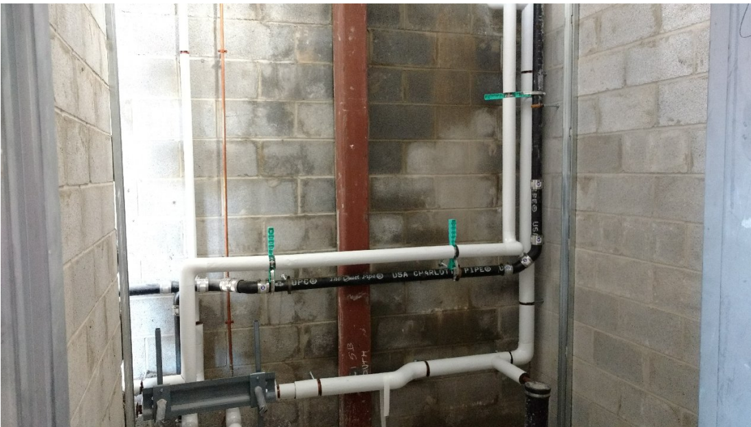
Seth Boyden School - Bathroom Rough plumbing
