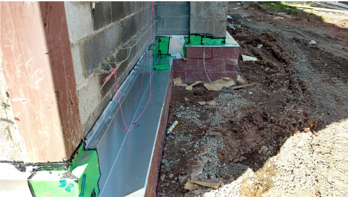
Seth Boyden School - CMU Block flashing
