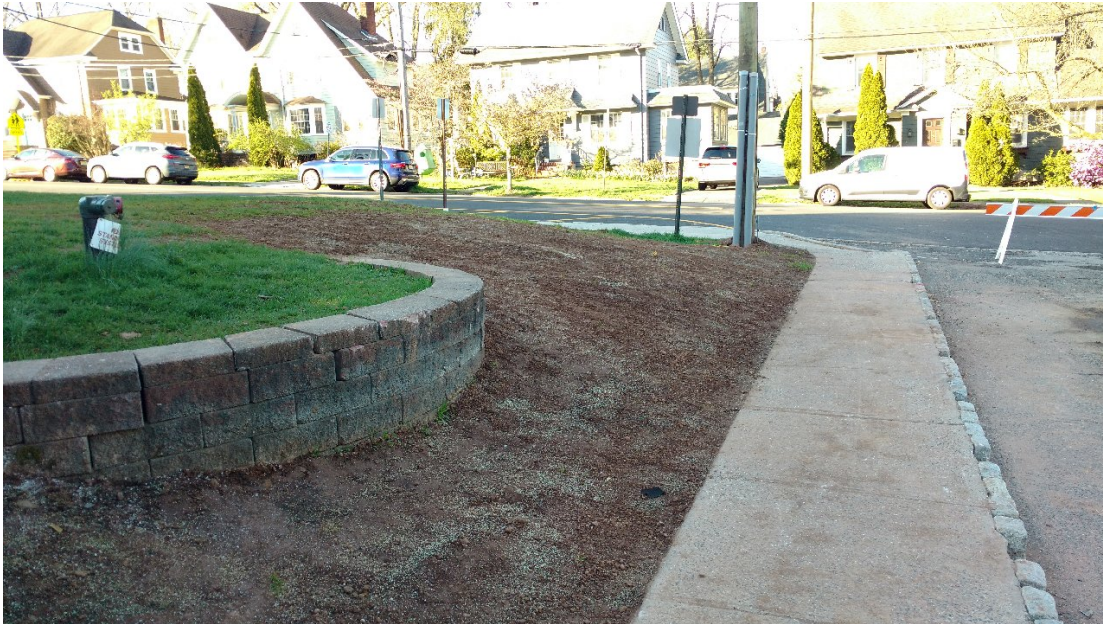
Tuscan School– Primary underground conduit installed and area graded
