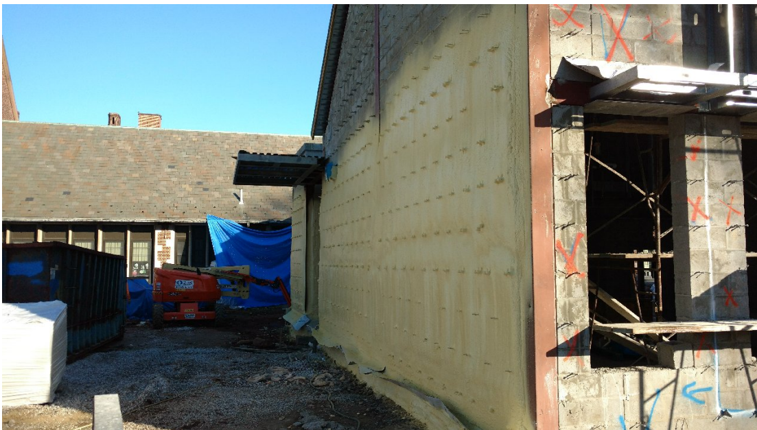
Tuscan School – Exterior Spray Foam Insulation Installed on South Elevation
