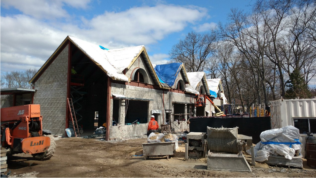
Tuscan School- 90 percent of CMU completed.
