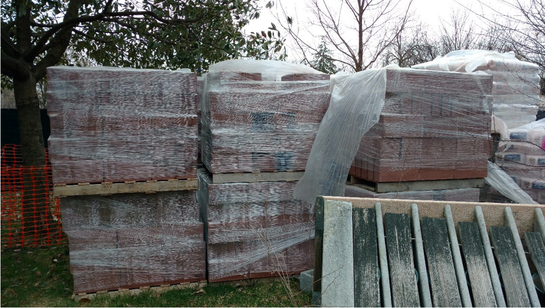
Seth Boyden School- Split-Face CMU on site
