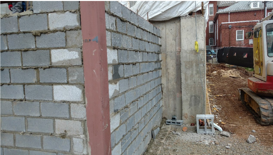
Seth Boyden School - CMU at Lower level Stair Tower
