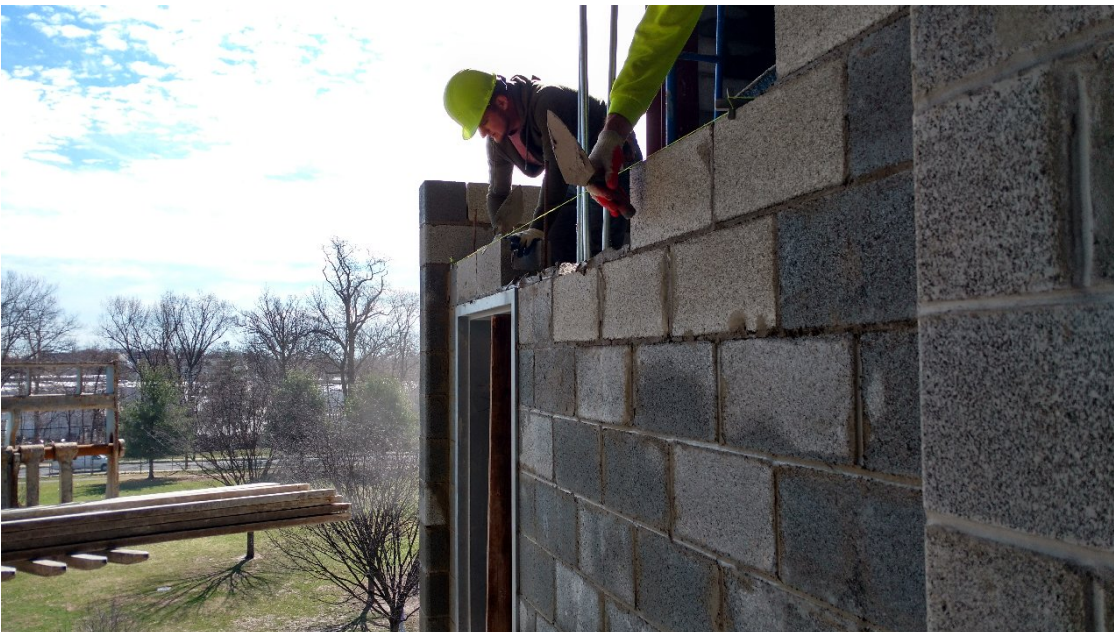
Seth Boyden School - CMU at 2 nd floor Privacy Room
