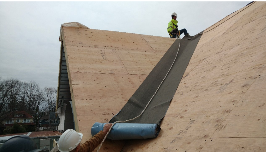
Tuscan School -Ice Shield Installation at Dormer Valley
