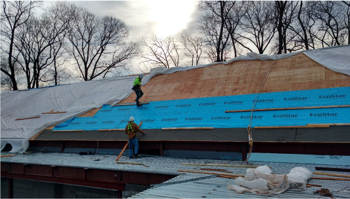
Tuscan School- Sloped Roof Underlayment Installation
