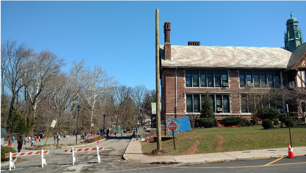
Tuscan School- New site Utility Pole
