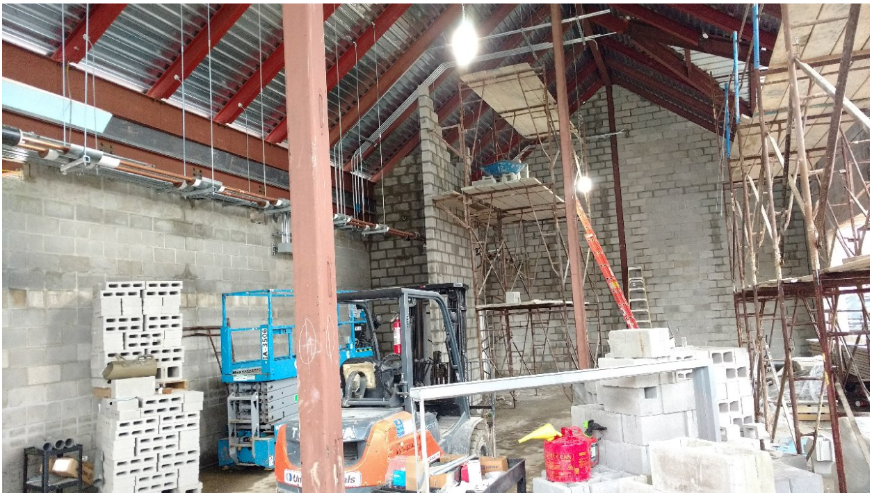
Tuscan School - CMU placement at classroom separation wall
