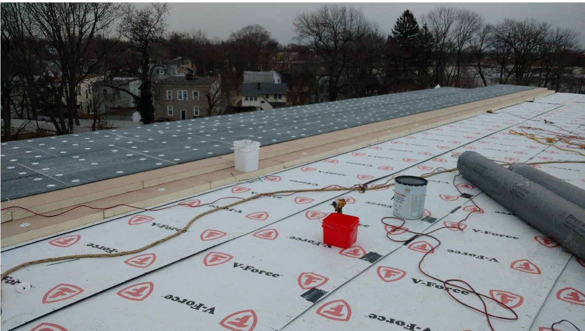
Seth Boyden School - New Addition Roofing
