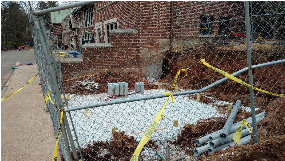
Tuscan School –Exterior Transformer Pad Sub-grade
