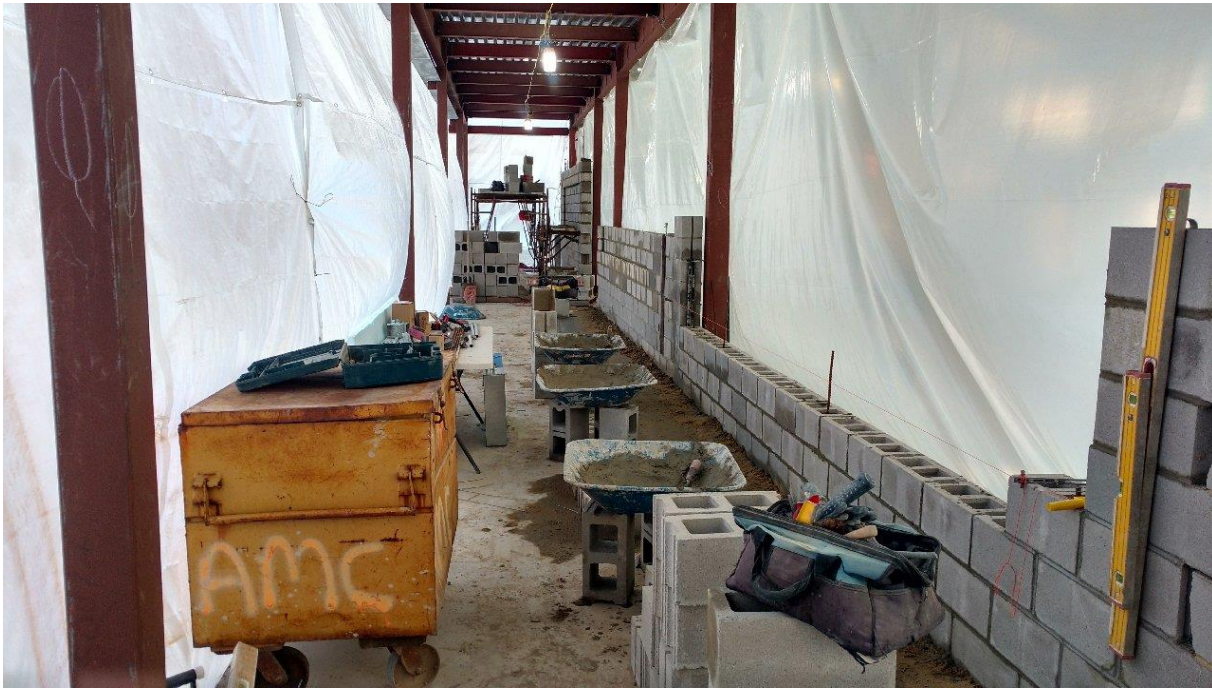
Tuscan School– Interior Corridor CMU Walls
