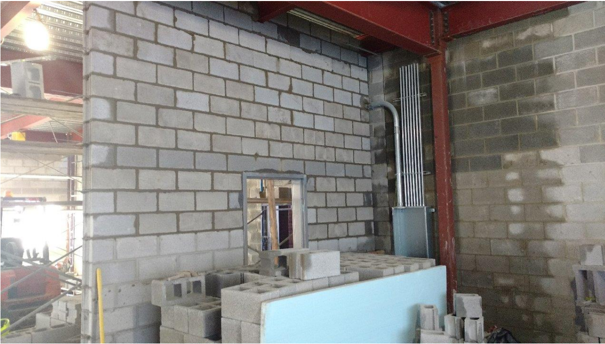
Seth Boyden School- First Floor Corridor Wall
