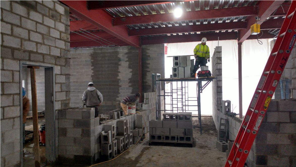
Seth Boyden School - First Floor corridor Walls
