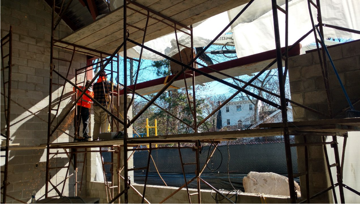
Tuscan School- Window Lintel Steel
