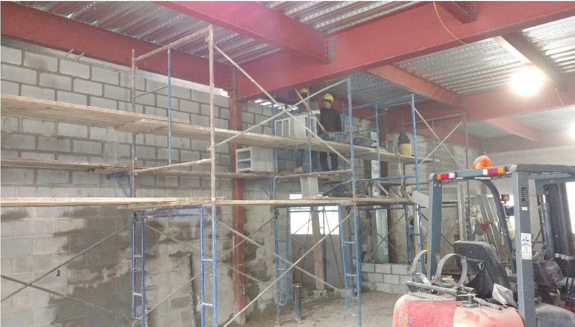
Seth Boyden - Fire wall constructed to the first floor ceiling height
