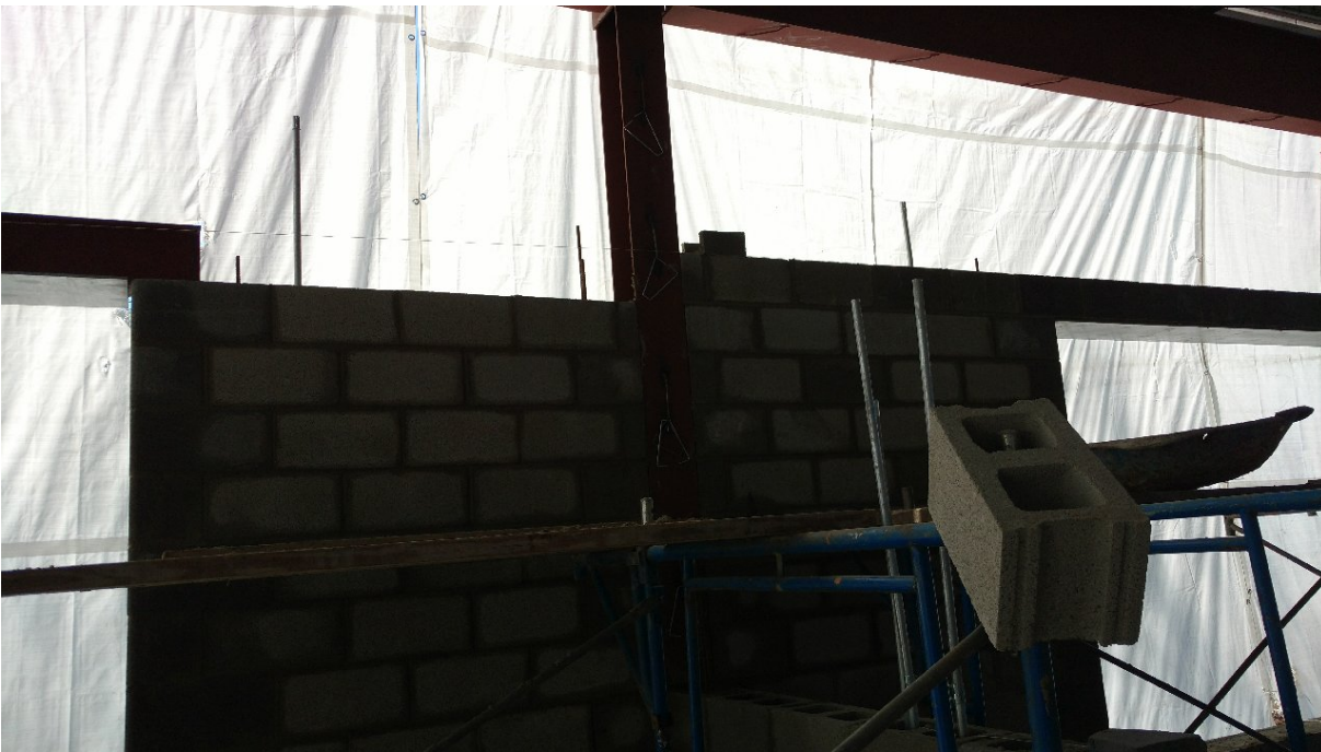
Seth Boyden- Second Floor CMU Exterior Wall
