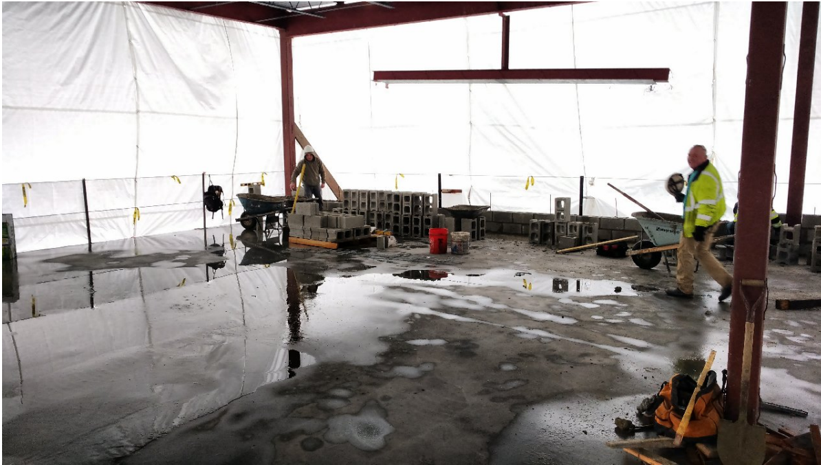
Seth Boyden- Second floor Exterior wall CMU placement
