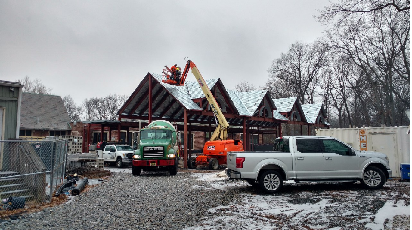
Tuscan School - Metal Decking Installation
