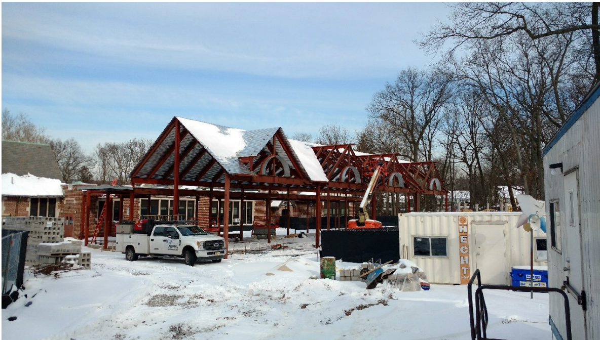
Tuscan School - Structural steel installation
