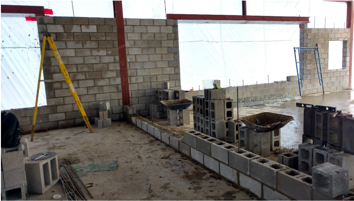
Seth Boyden School - CMU walls
