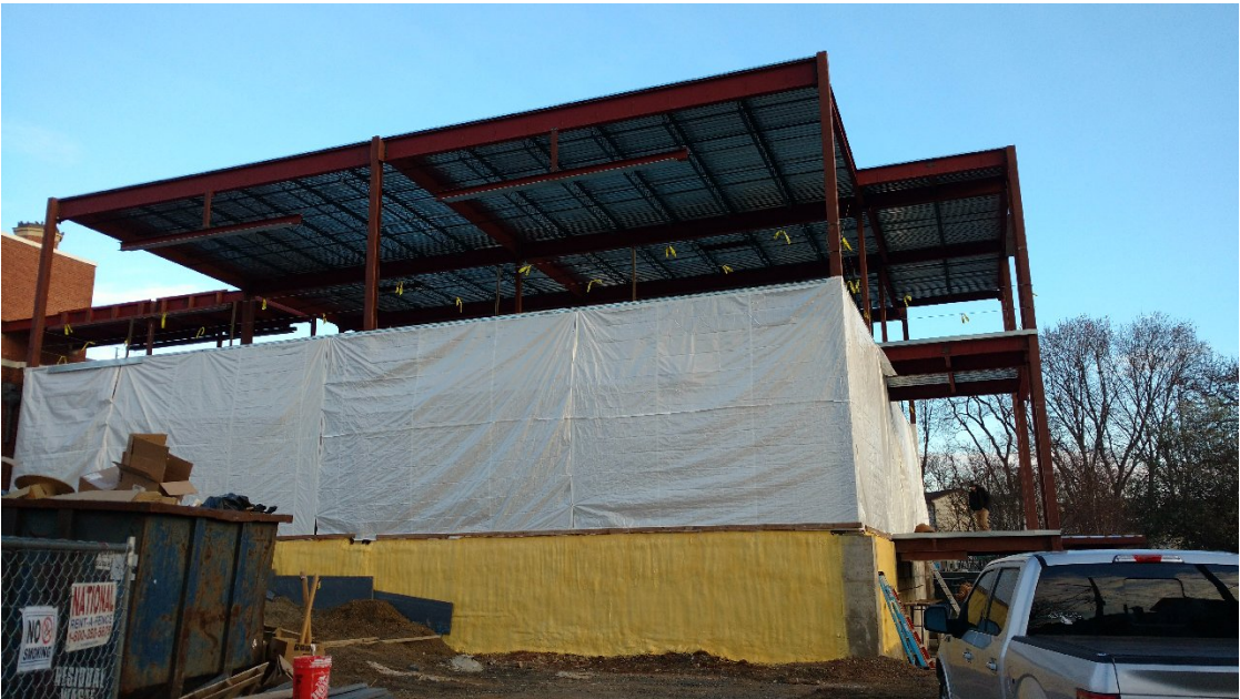
Seth Boyden - Structural Steel/First floor Temp enclosure
