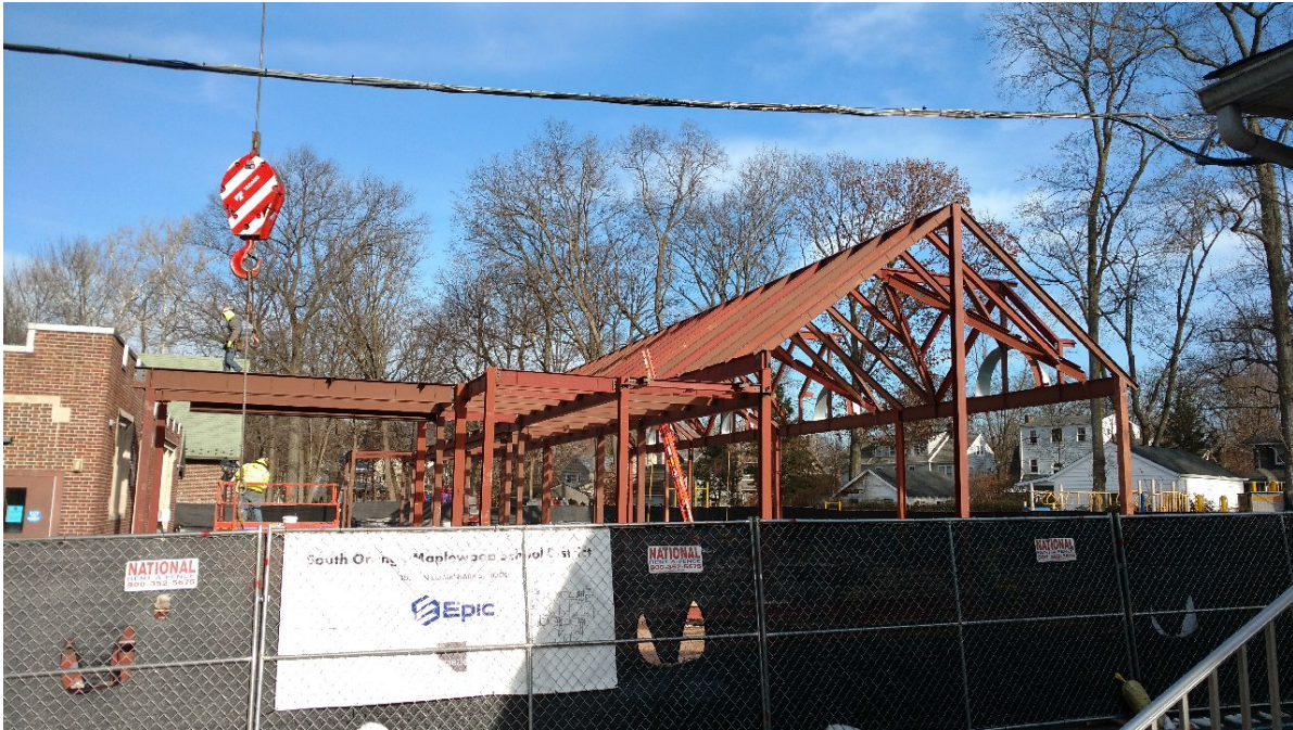
Tuscan School - Structural Steel Installation
