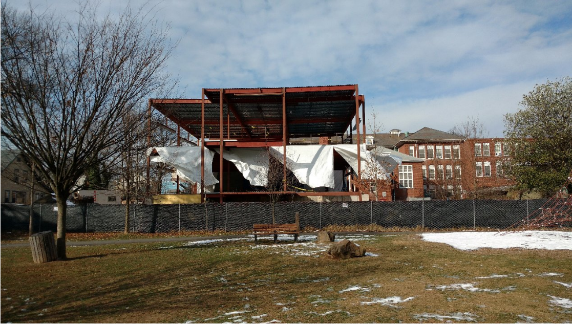
Seth Boyden- Structural Steel/First floor Temp enclosure
