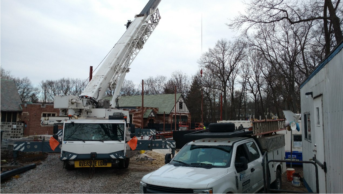
Tuscan School - Structural Steel Installation
