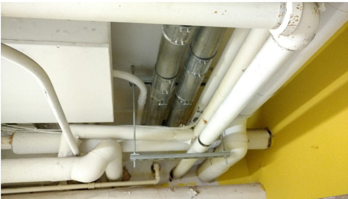
Tuscan School - New Electrical Feeder conduit to Existing Switchgear
