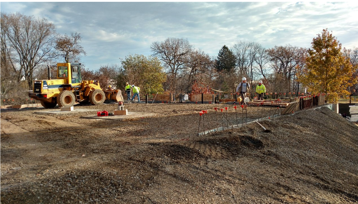
Seth Boyden - 3/4 inch drainage materials being placed
