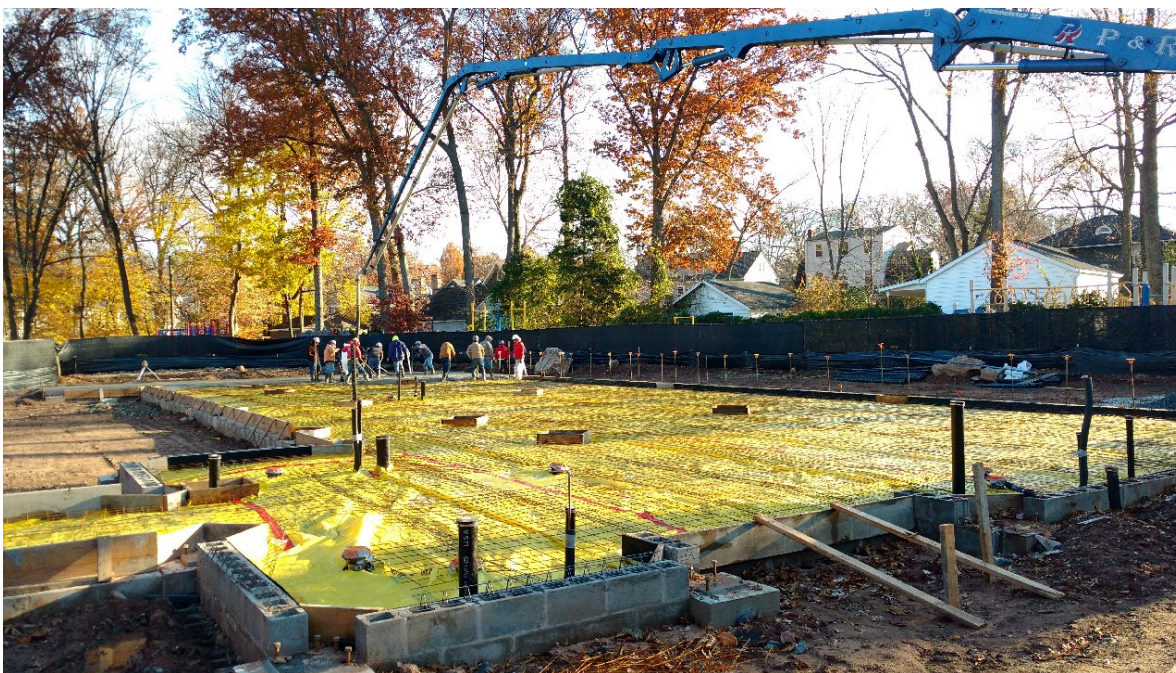
Tuscan School - Concrete Slab on Grade Placement
