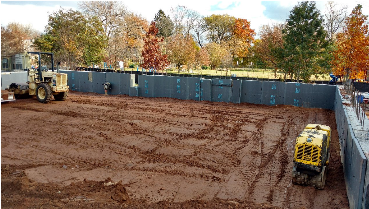
Seth Boyden- Foundation Wall Soil Backfilling
