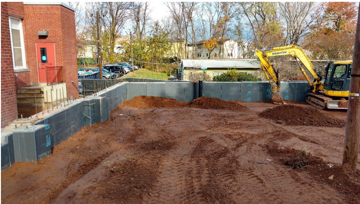
Seth Boyden - Foundation Wall Soil Backfilling
