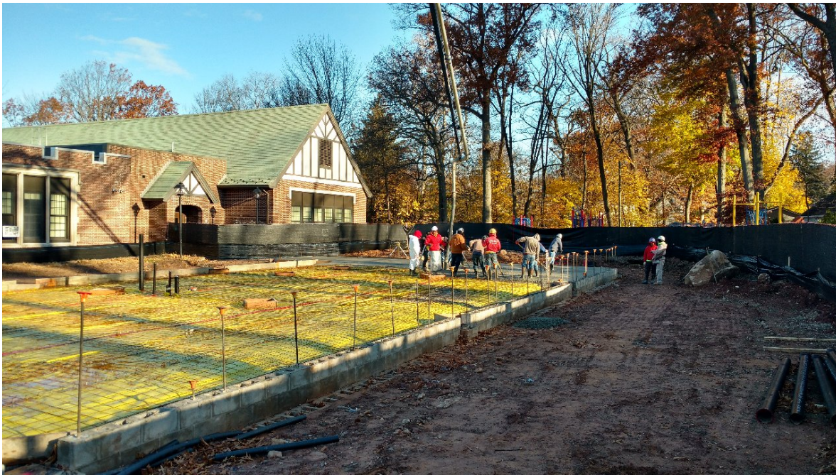
Tuscan School - Concrete Slab on Grade Placement
