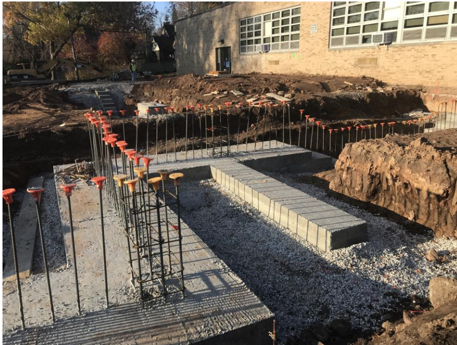
Poured footings - Jefferson Elementary School
