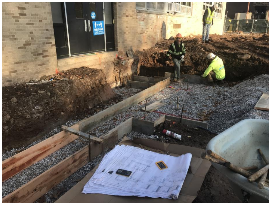
Preparing another footing section for rebar and concrete Jefferson Elementary School
