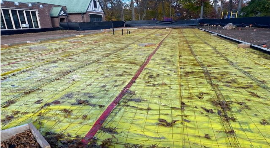
Installing wire mess/rebar– Tuscan Elementary School
