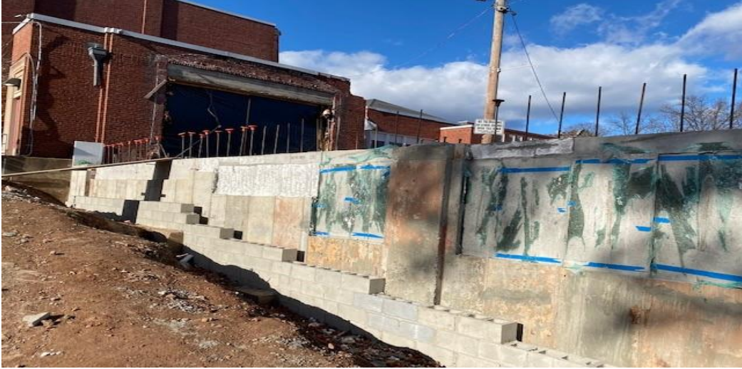
Installing CMU– Seth Boyden Elementary School
