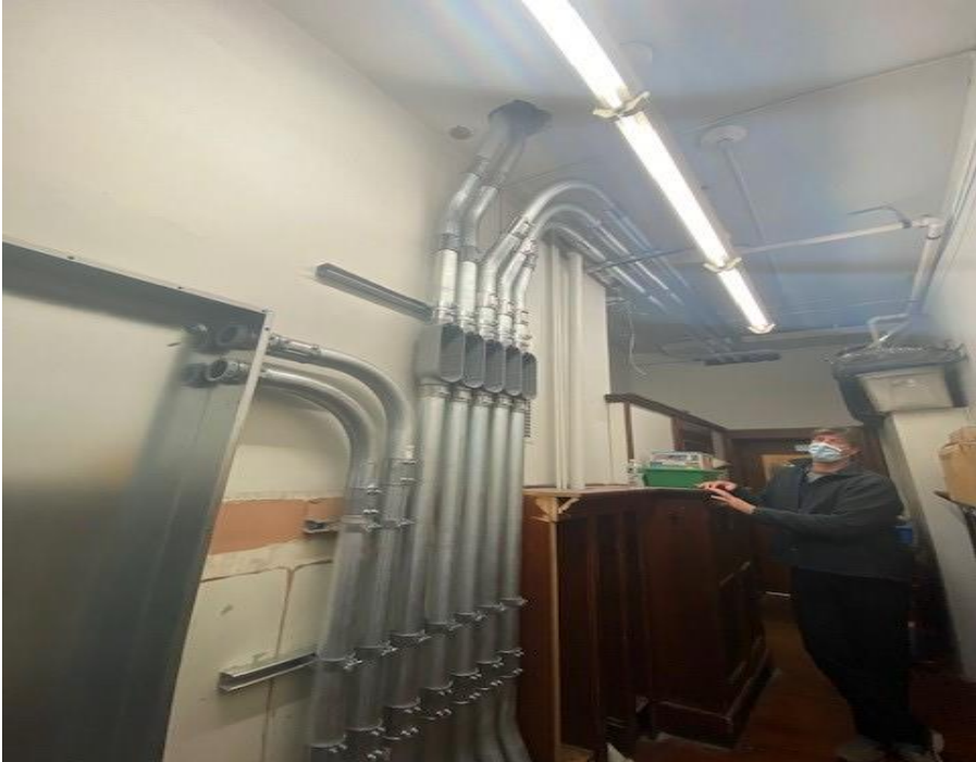
Running conduits in the school– Seth Boyden Elementary School
