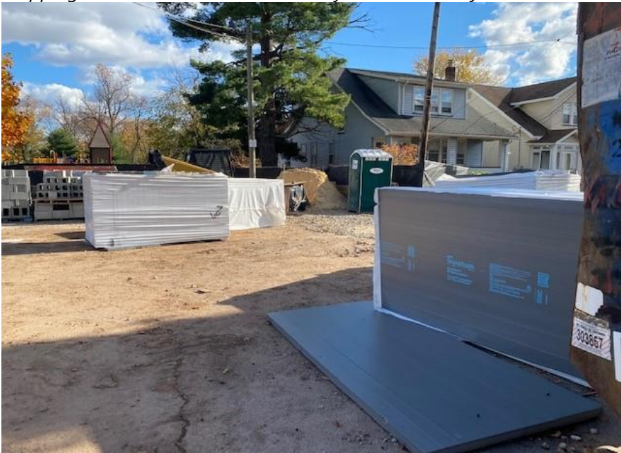
Prepping to install insulation– Seth Boyden Elementary School
