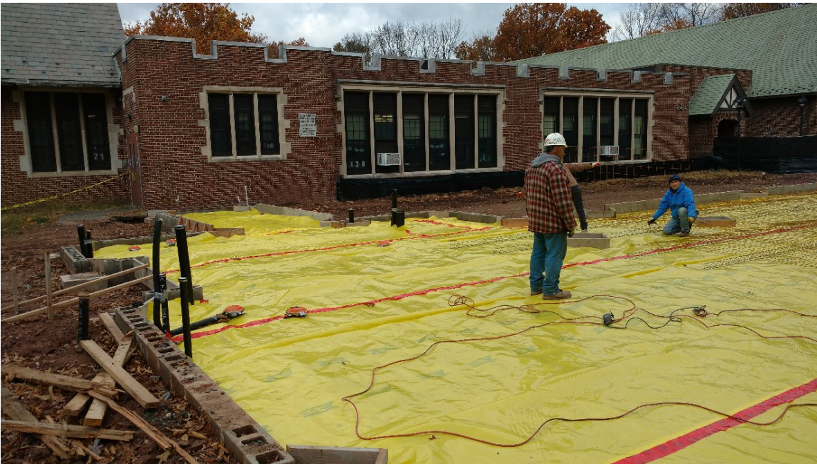
Tuscan School - Vapor barrier/wire mesh
