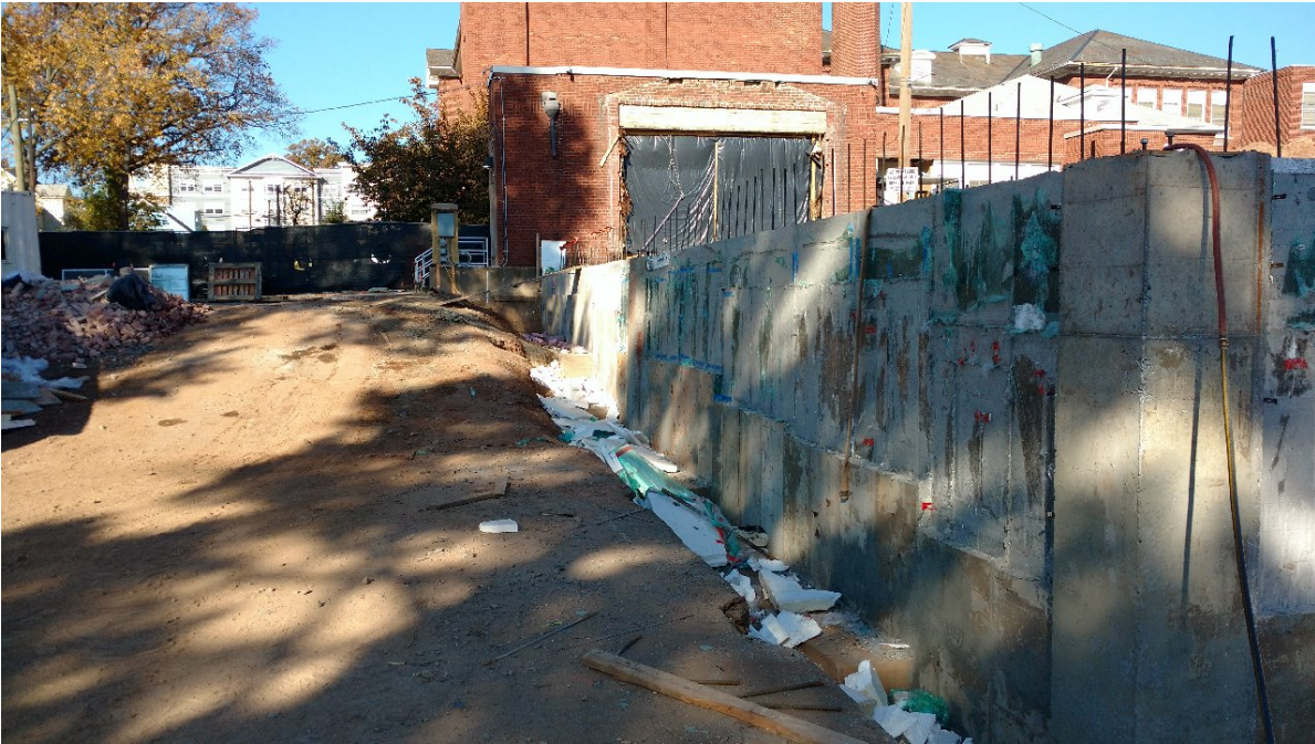
Seth Boyden- New Concrete Foundation Wall
