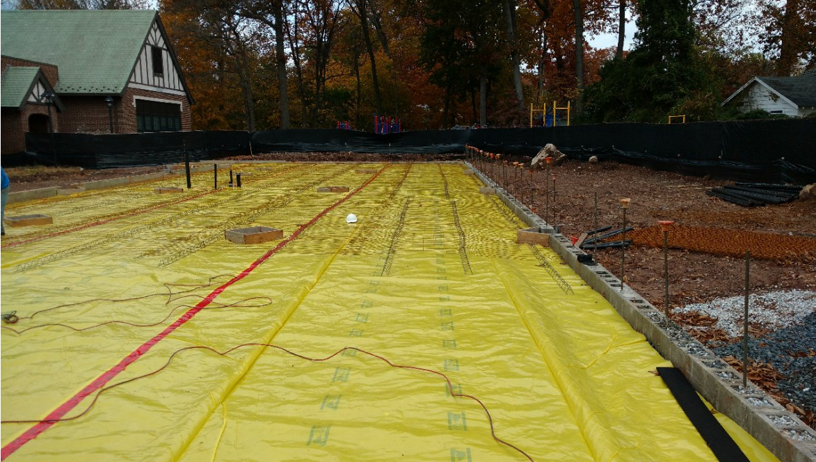
Tuscan School - Vapor barrier/wire mesh
