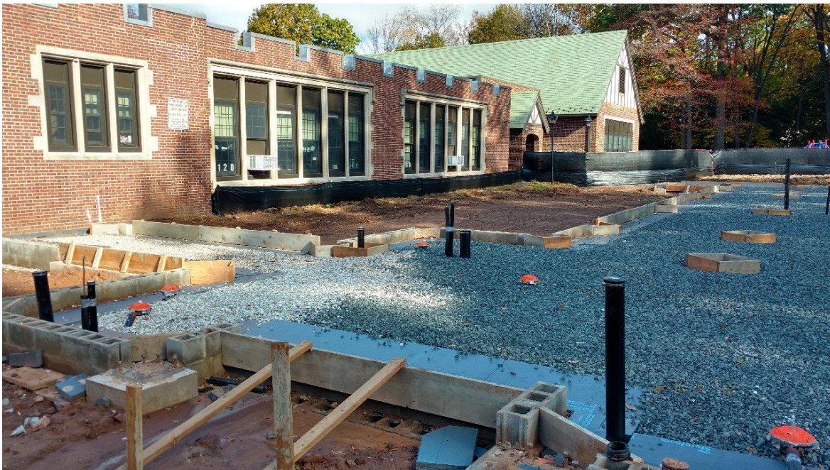
Tuscan School - Slab on Grade
