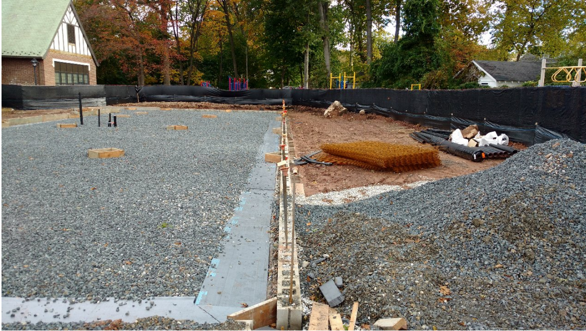
Tuscan School - Slab on Grade
