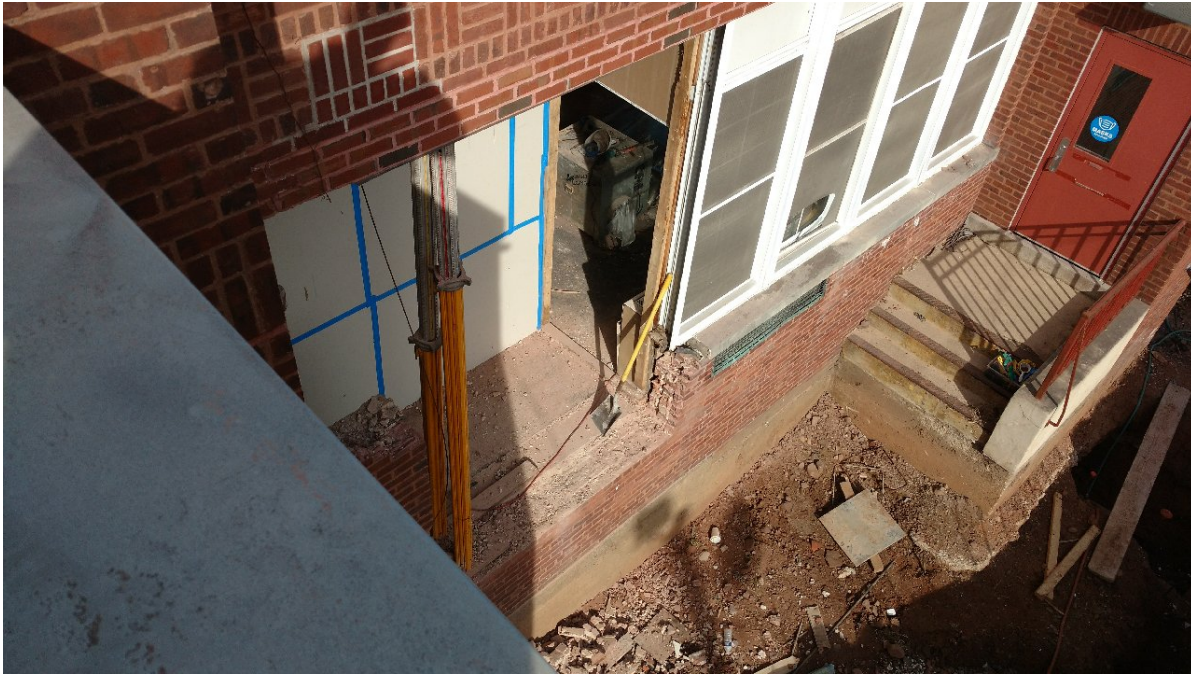
Seth Boyden- Demo existing wall
