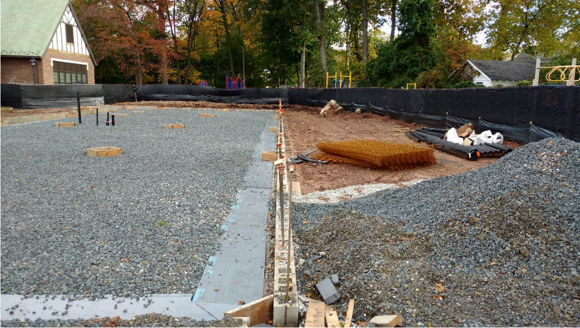
Tuscan School - Slab on Grade
