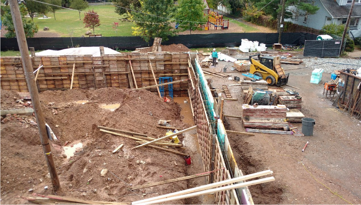
Seth Boyden- Foundation Wall Forms
