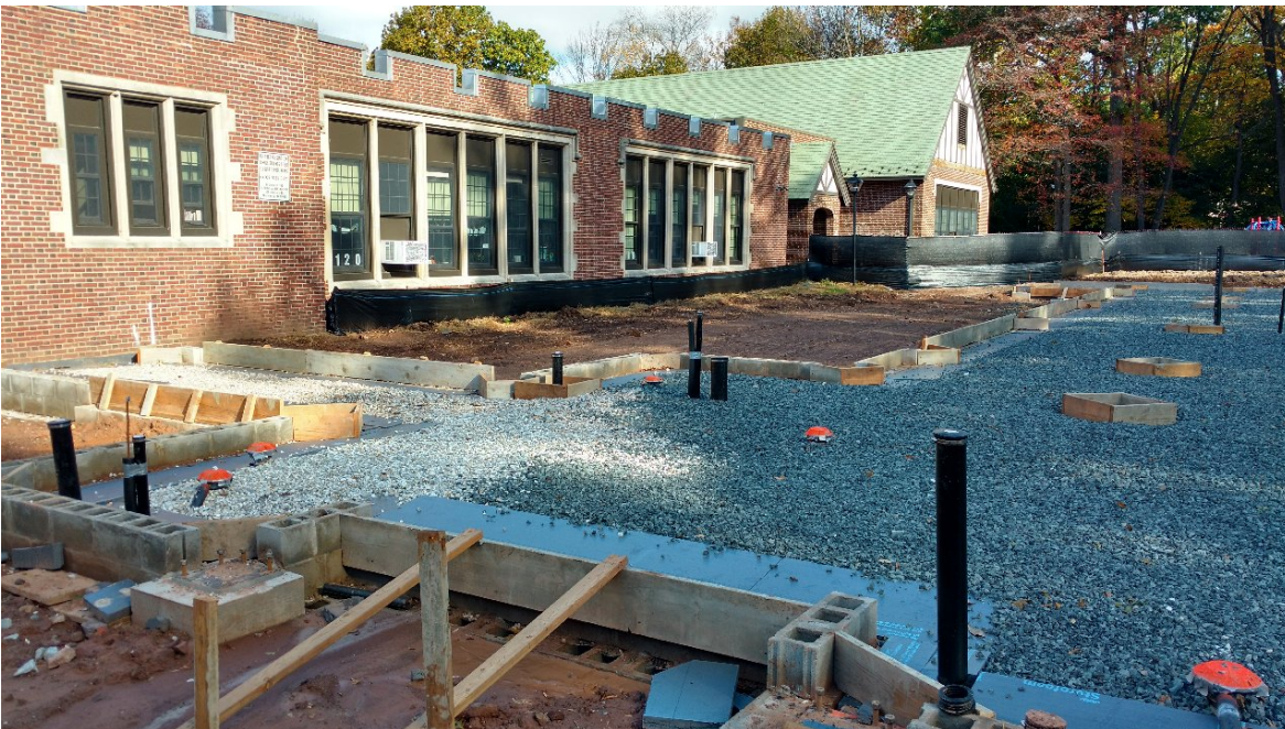
Tuscan School - Slab on Grade
