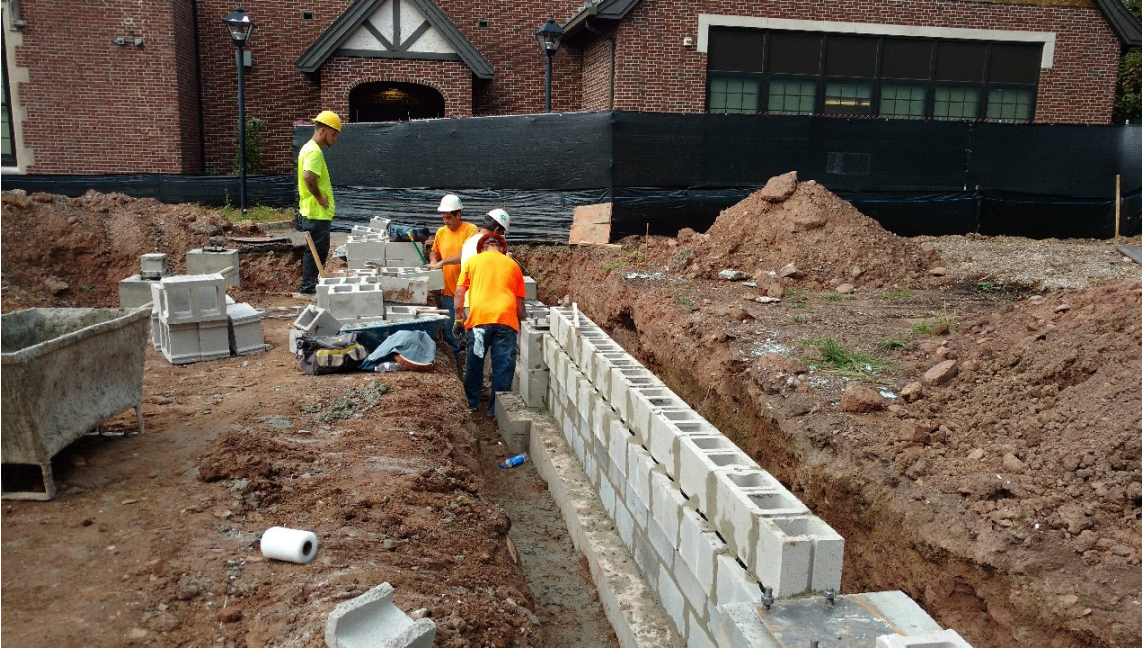
Tuscan School - Concrete Masonry Units (CMU) being placed
