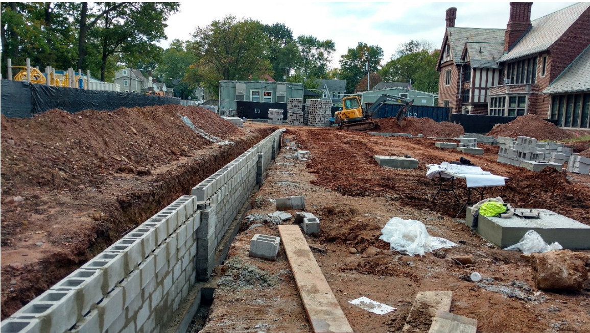
Tuscan School - CMU Foundation wall
