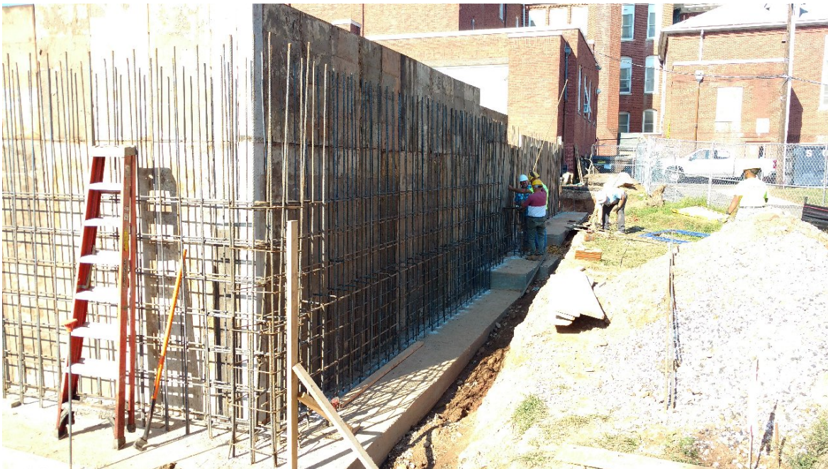
Seth Boyden School - Reinforcing steel at foundation wall forms
