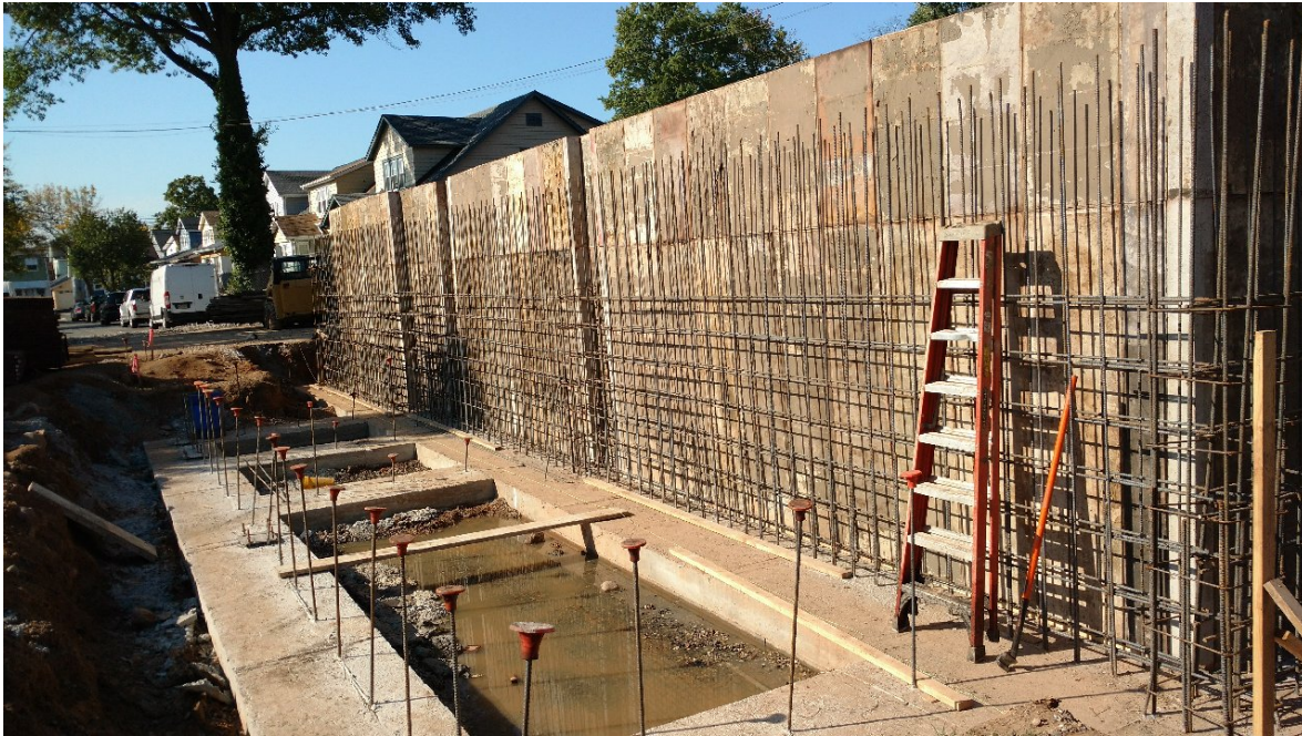
Seth Boyden- Foundation Wall Forms
