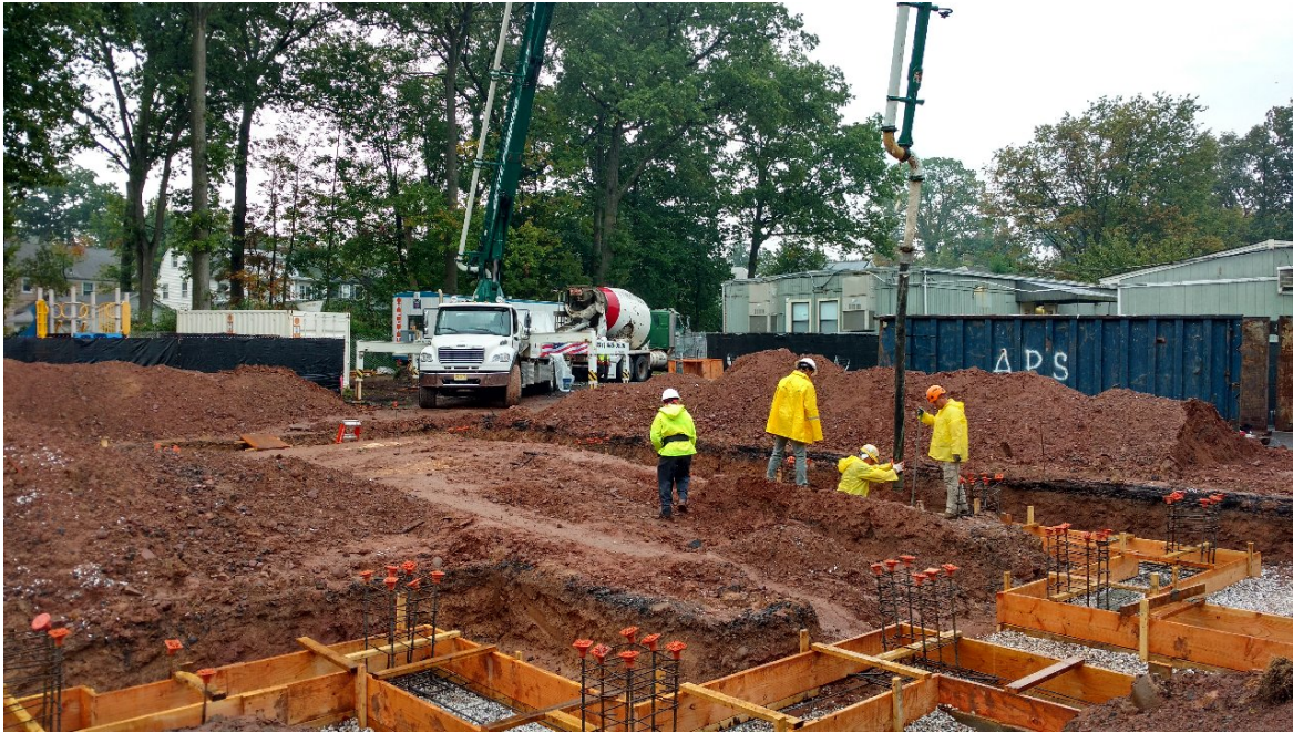
Tuscan School - Concrete footing placement
