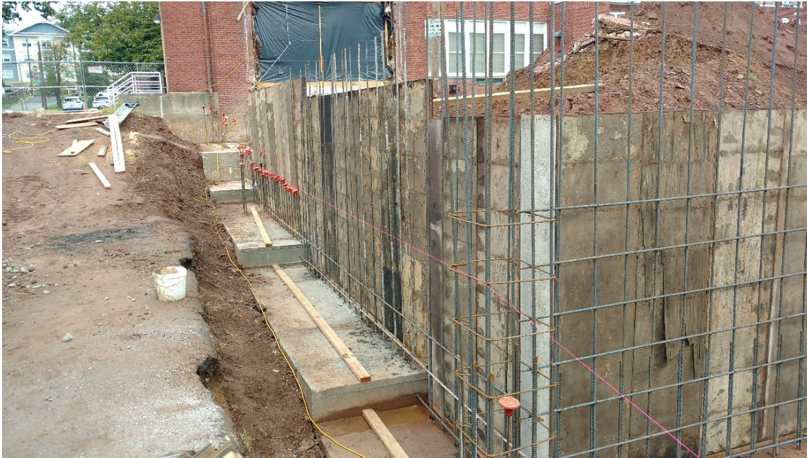
Seth Boyden- Foundation Wall Forms
