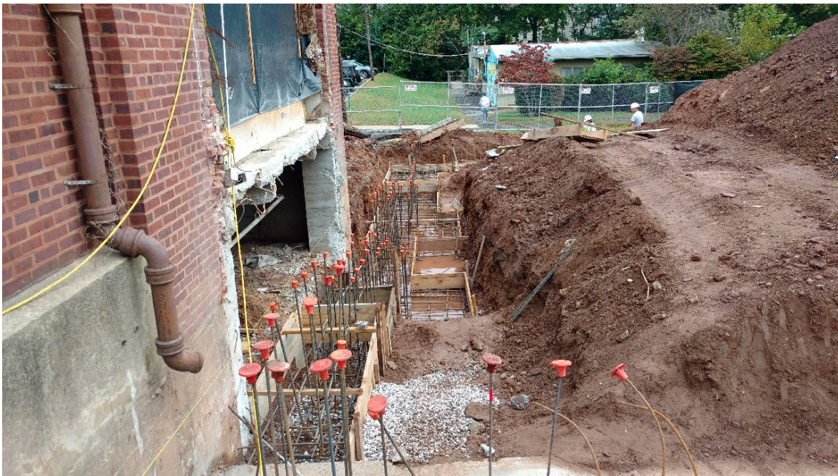
Seth Boyden School - Reinforcing steel at Step footing (demolished Bow window)
