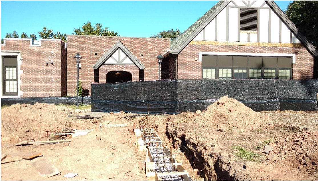
Tuscan School - Footing form placement/ Silt fence/Privacy screen
