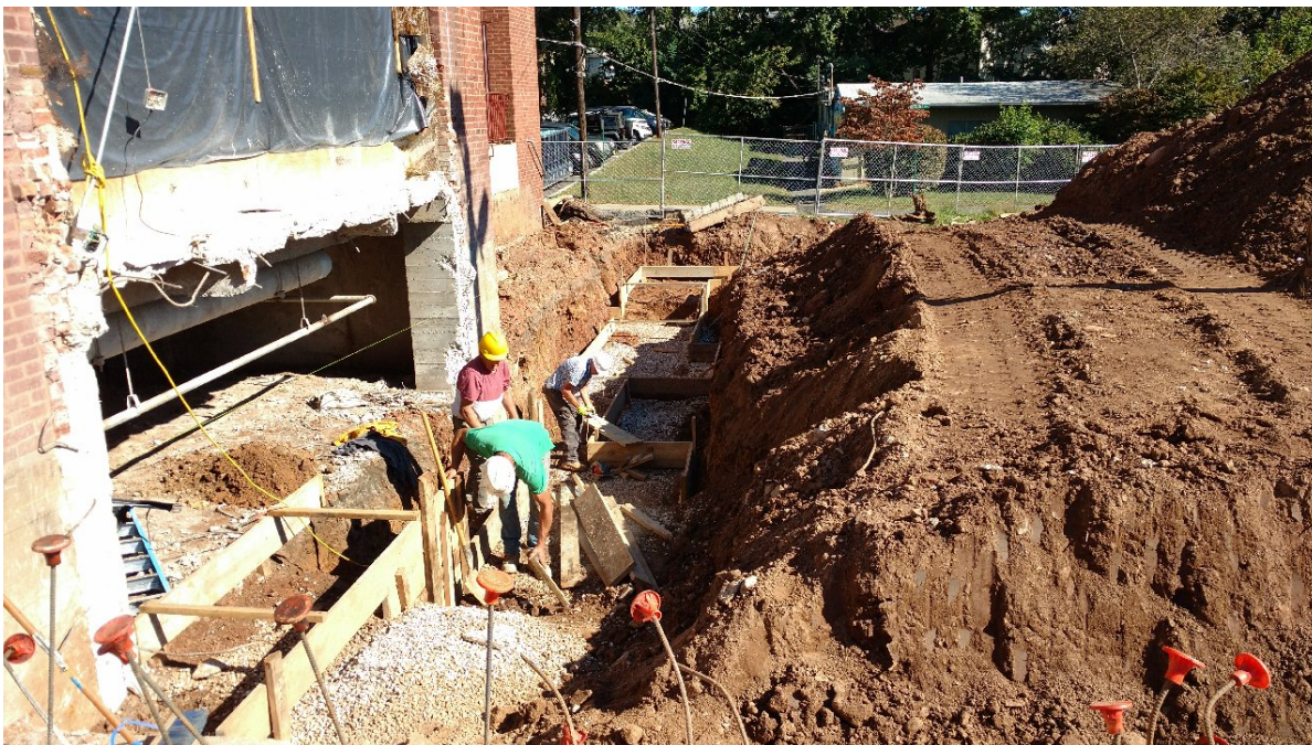
Seth Boyden School -Step footing at demolished Bow window
