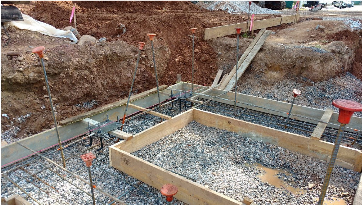
Seth Boyden- Exterior Stair footing
