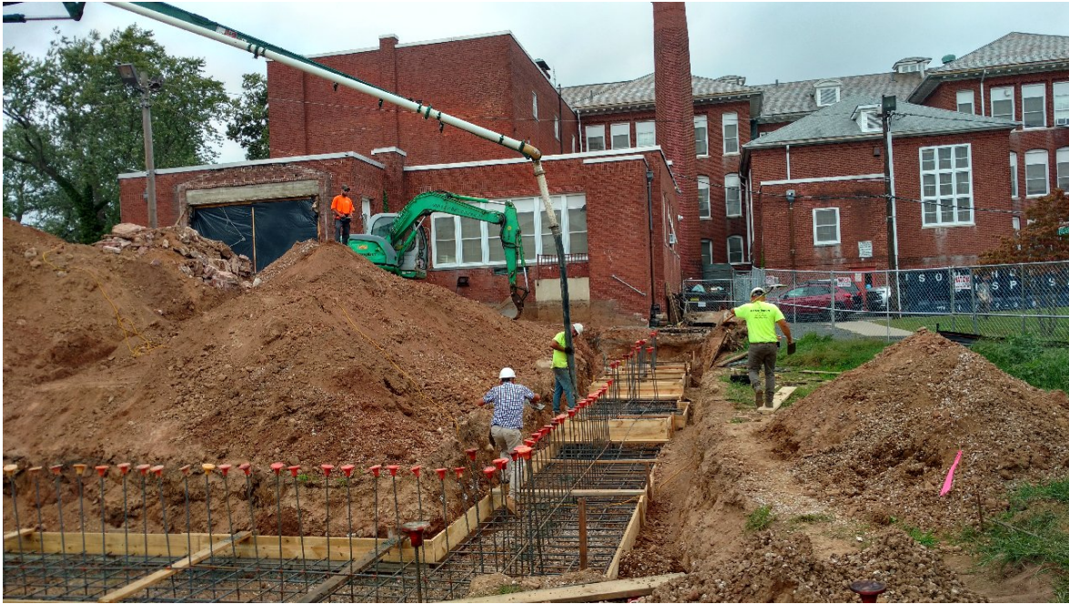
Seth Boyden- footing Concrete Placement
