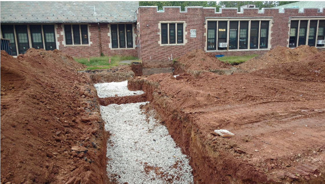
Tuscan School - Footing form placement
