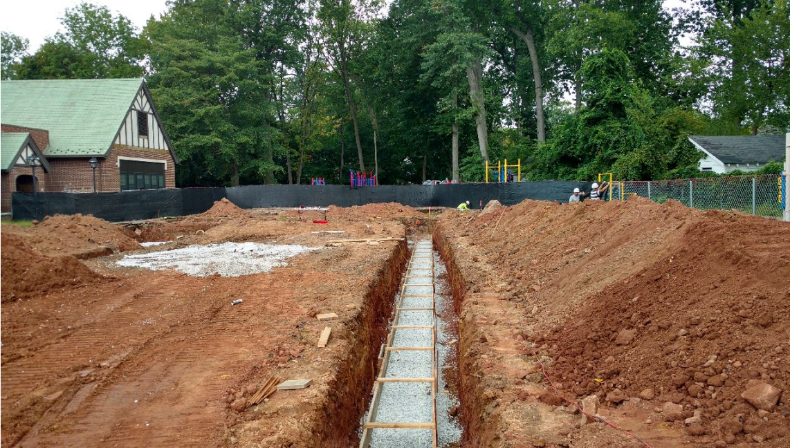
Tuscan School - Footing form placement
