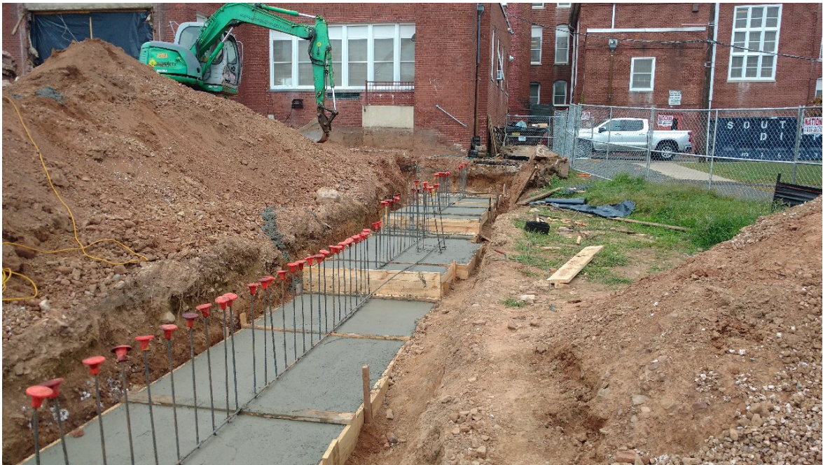
Seth Boyden School - Concrete Placement
