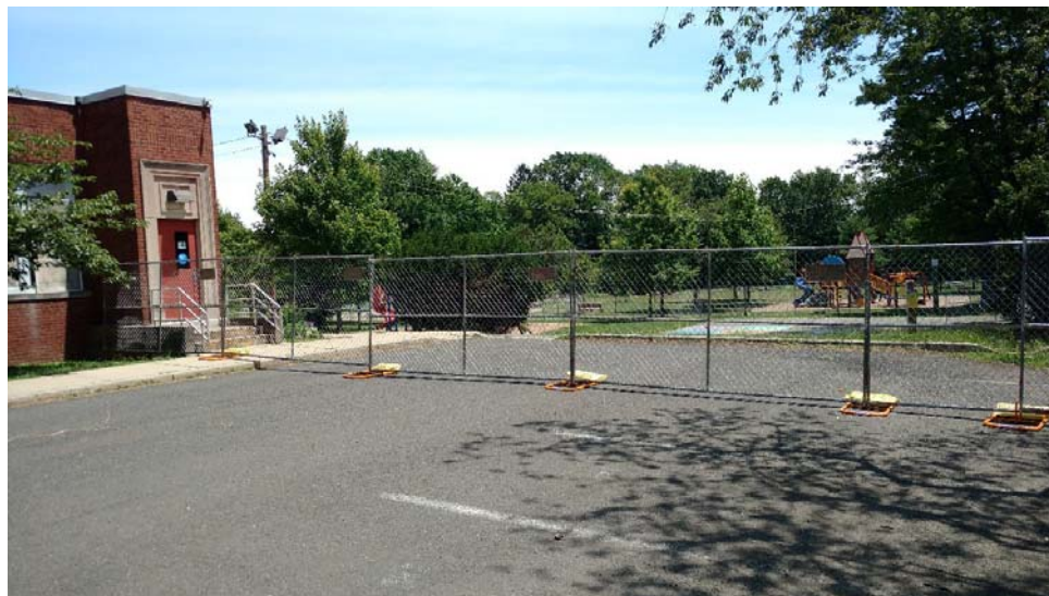
Seth Boyden School Temporary Construction Fence
