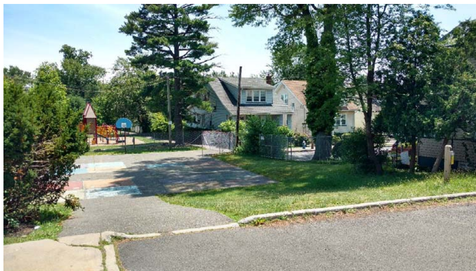
Seth Boyden School Temporary Construction Fence/Gate
