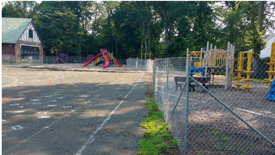
Tuscan School Temporary Construction Fence
