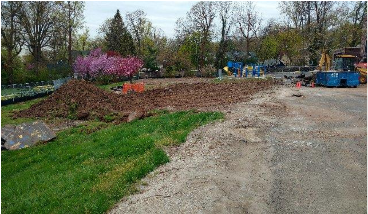
Strip topsoil
