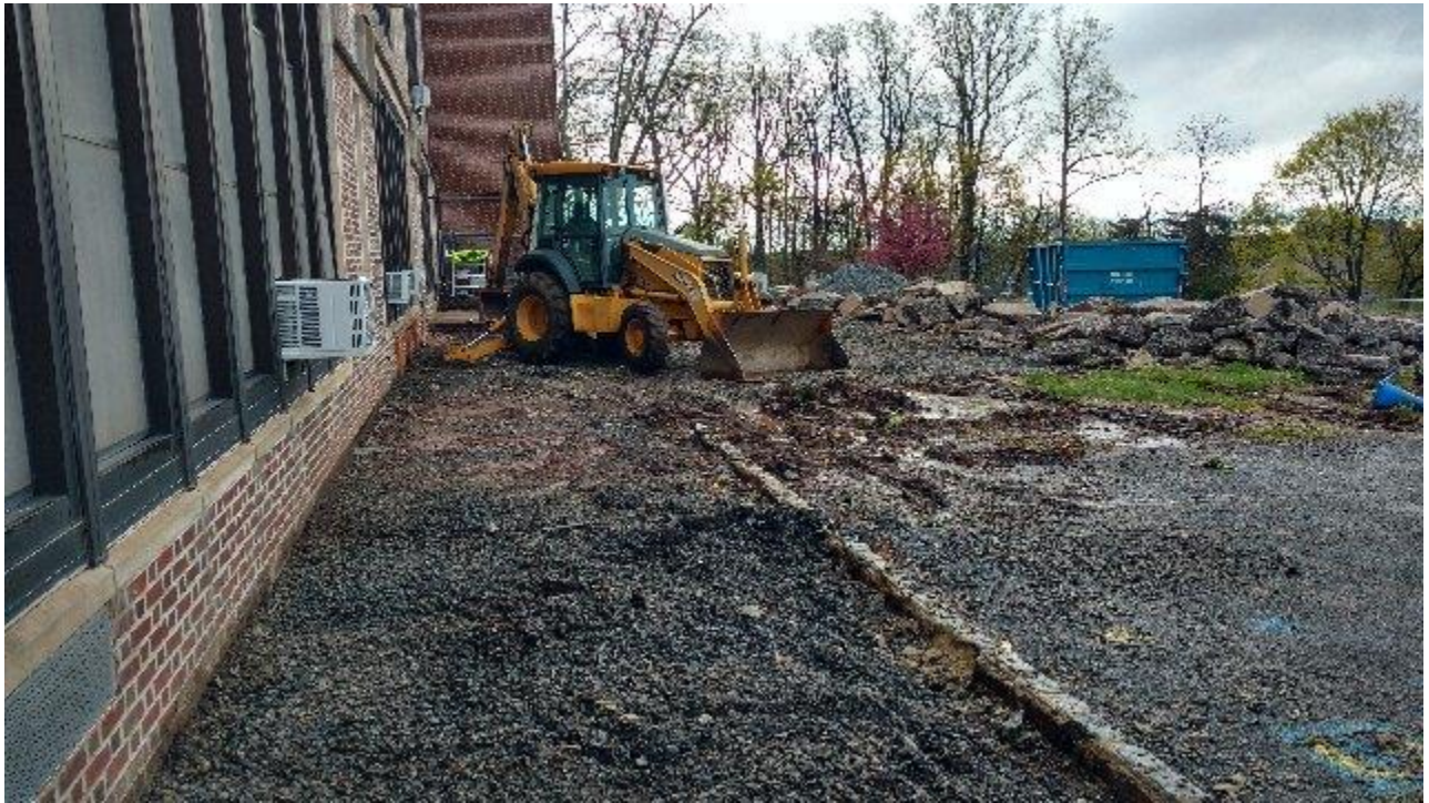
Sidewalk demo rear of elementary
