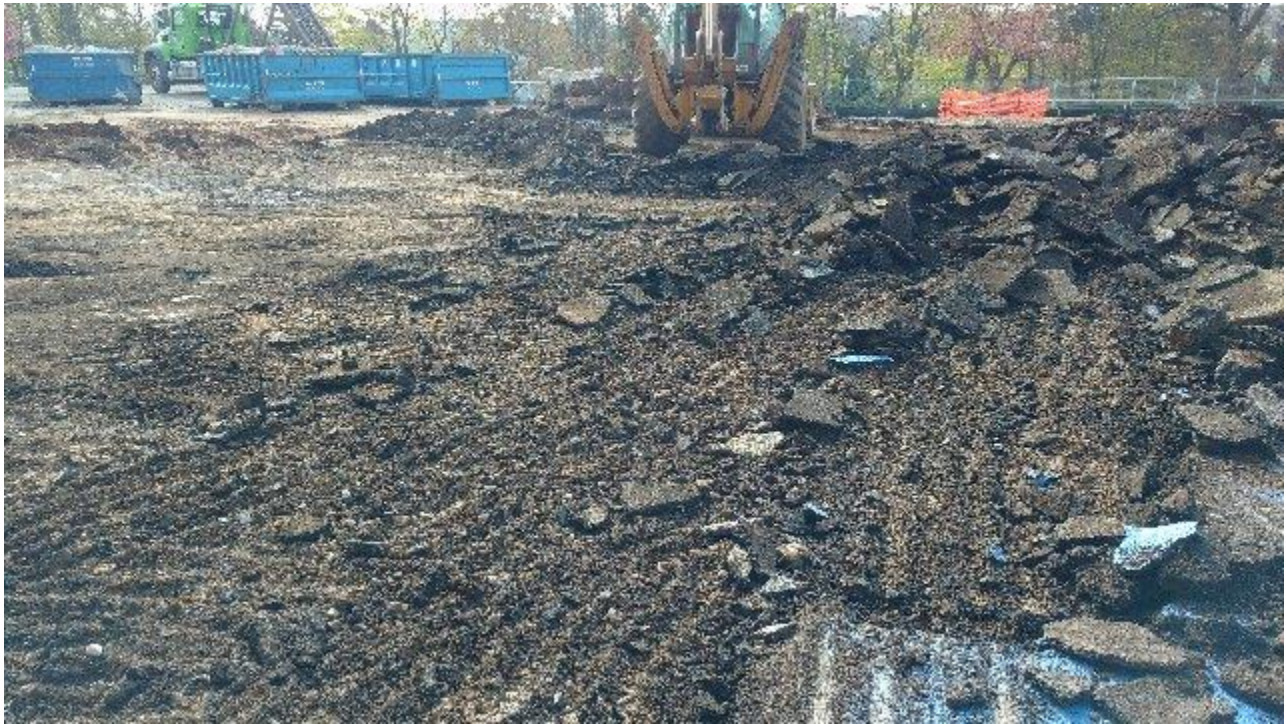
Removal of existing asphalt pavement
