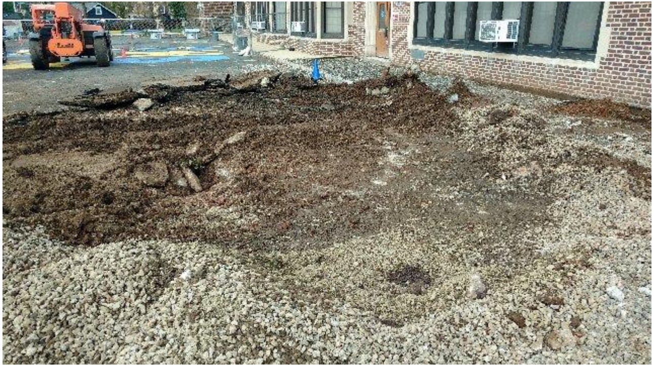
Encountered concrete slab under asphalt
