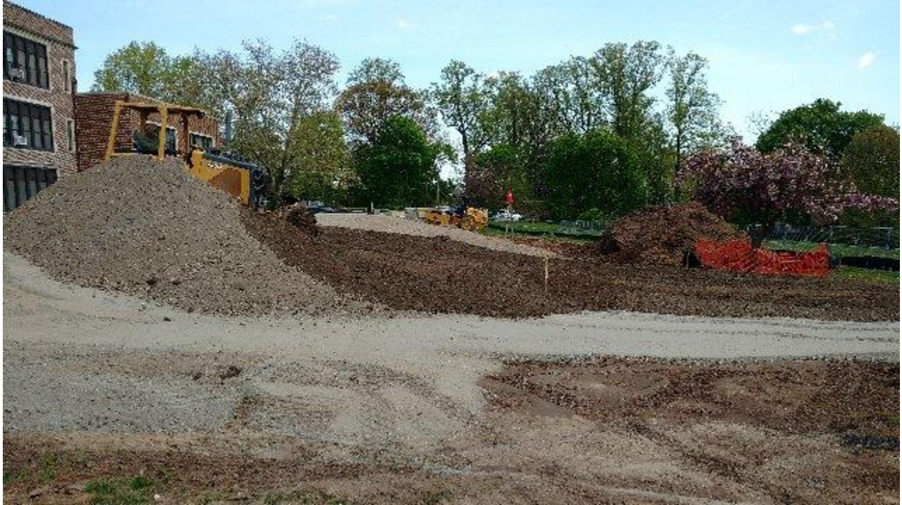
Grading DGA for proposed road at SME
