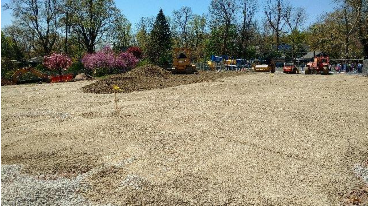
Grading DGA for proposed addition pad at SME
