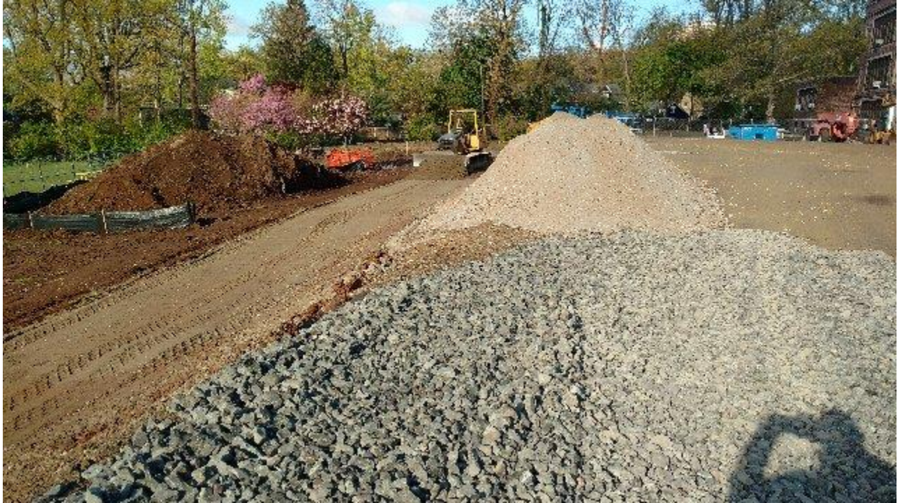
Grading DGA for proposed road at SME
