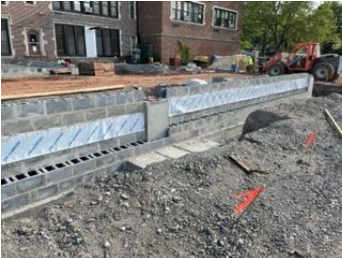
Foundation block at SME
