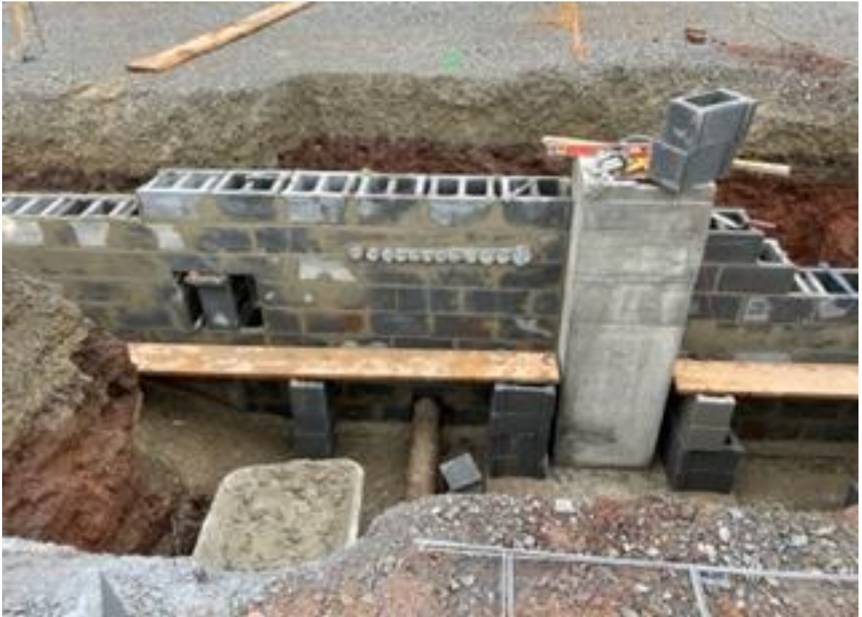
Foundation block walls/ Electric sleeves at SME
