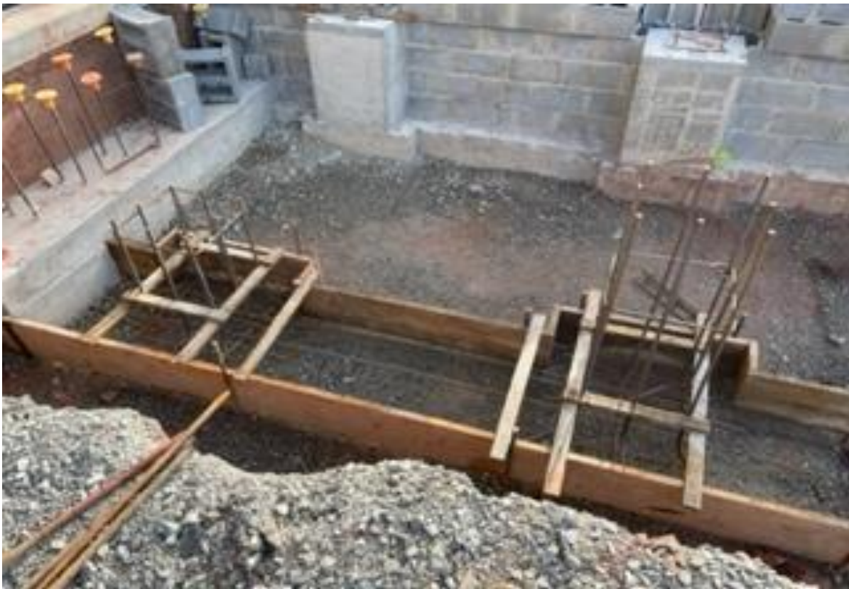
Footing forms, rebar, piers and foundation block at SME
