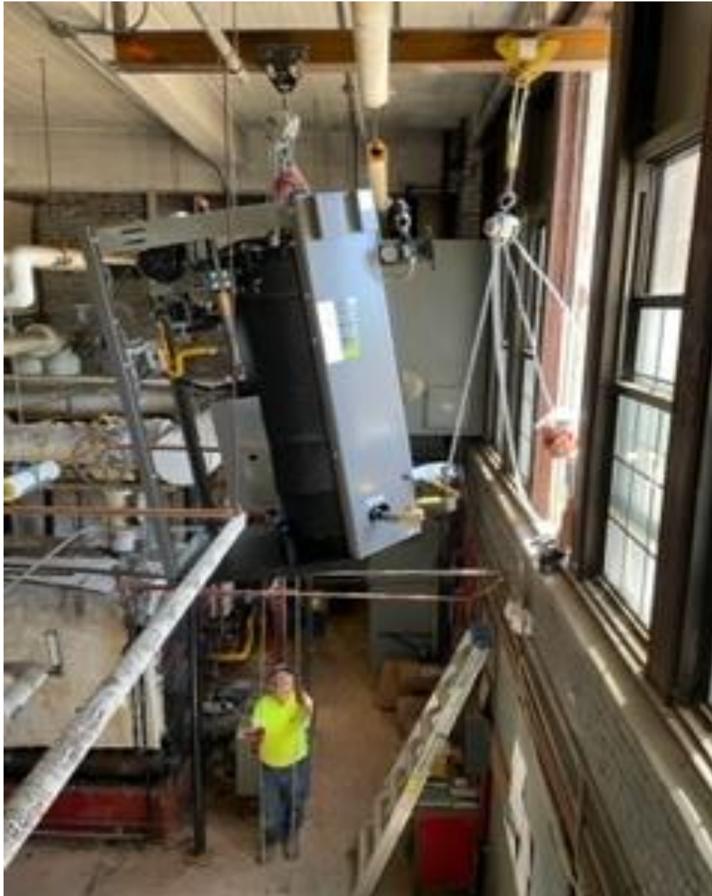
Hoisting in new boilers to basement at SME
