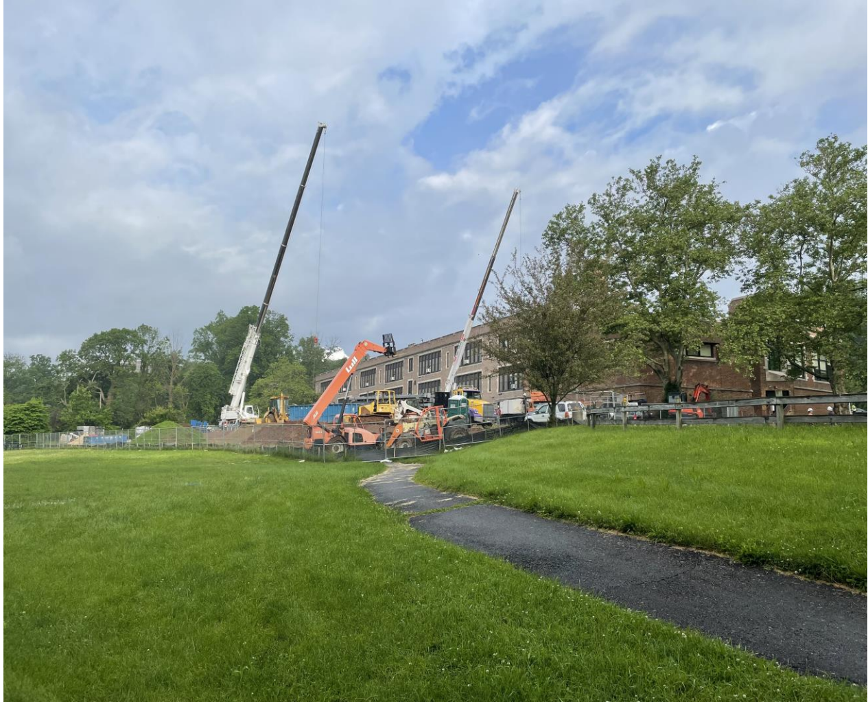
Cranes for steel and for roofing
