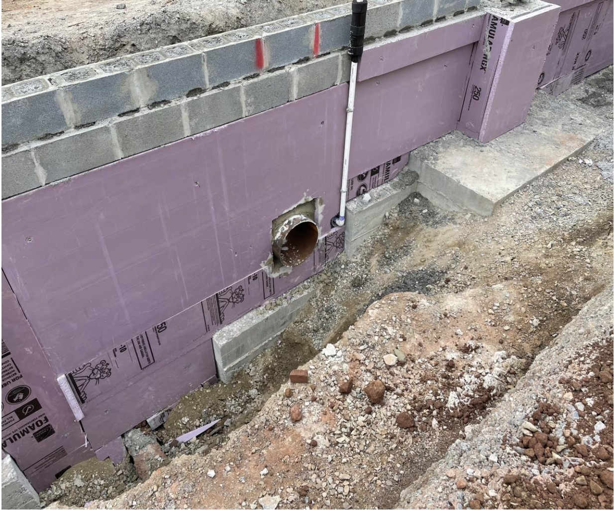
Foundation block and insulation at SME
