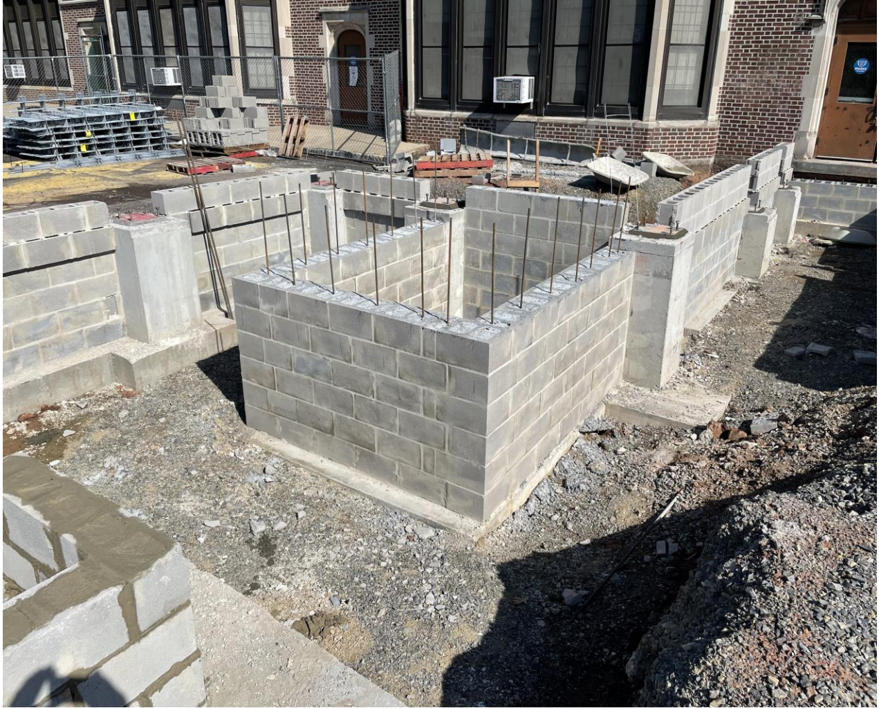
Elevator pit at SME
