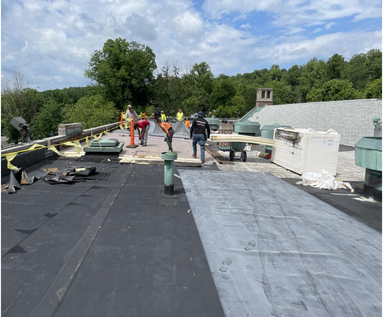
Demo existing roof & Install new insulation and EPDM at SME
