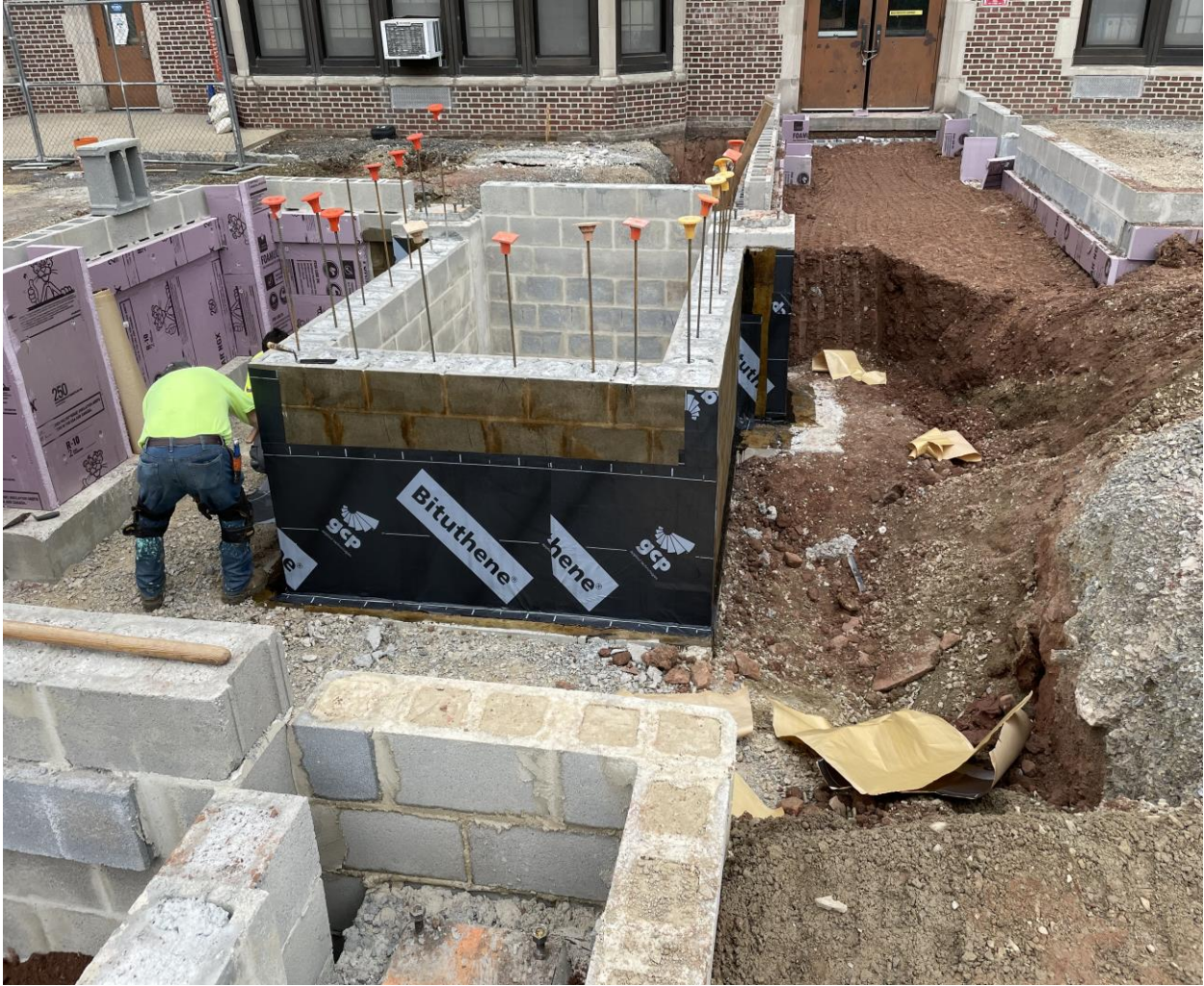
Waterproofing elevator pit at SME
