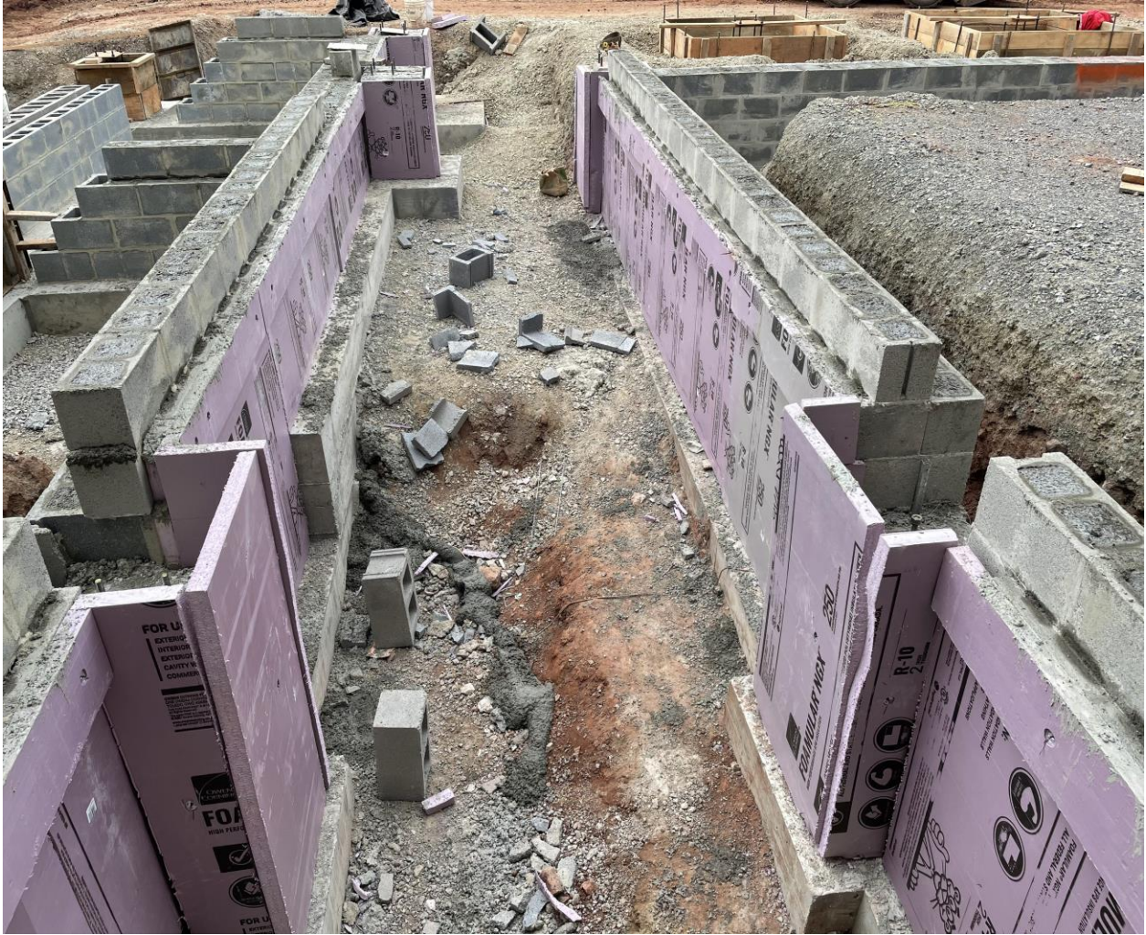
Foundation block and insulation at SME
