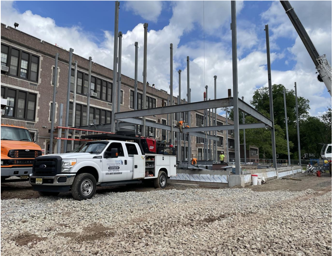
Steel erection at SME
