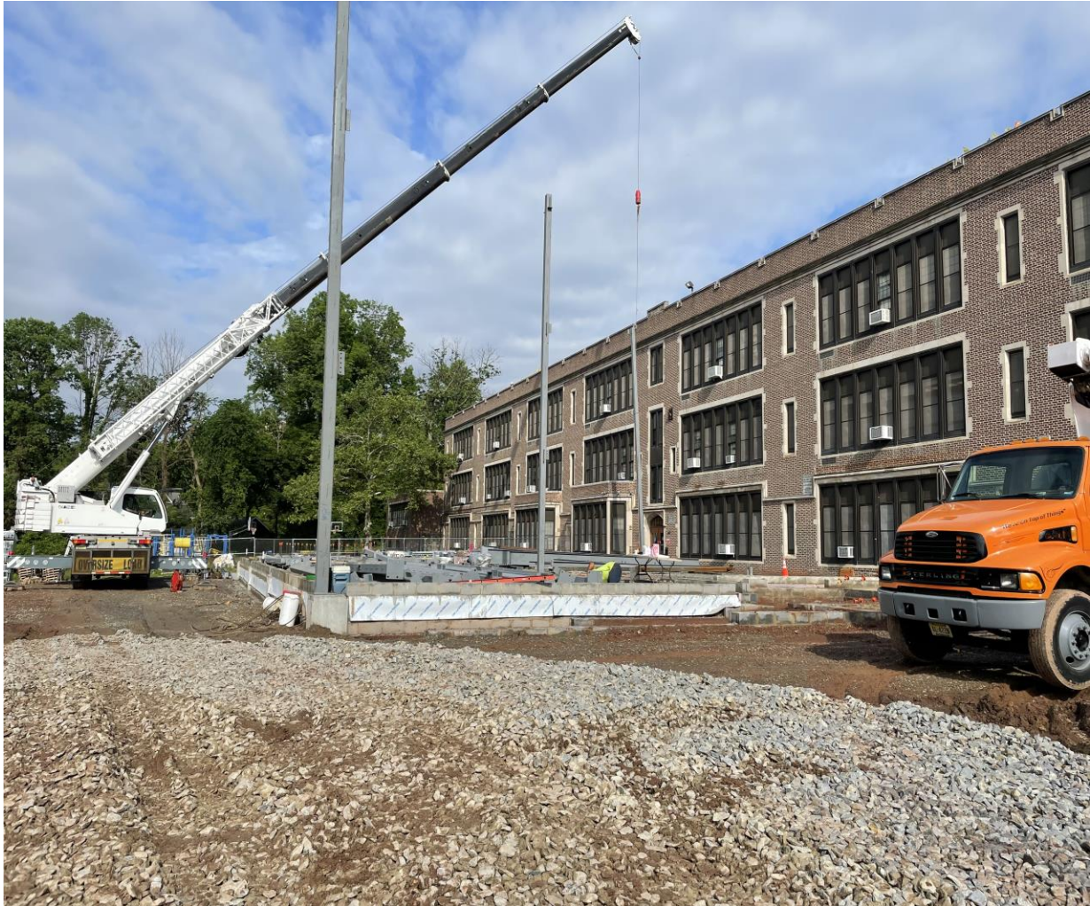
Steel erection at SME
