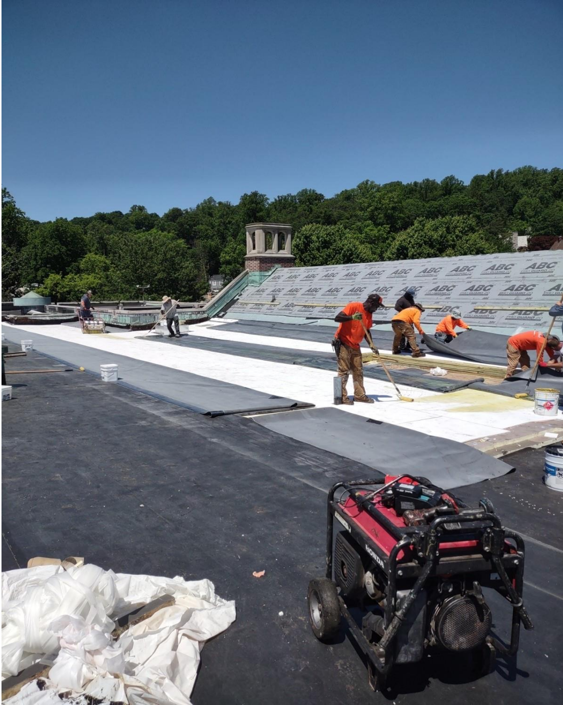
Roof replacement at SME
