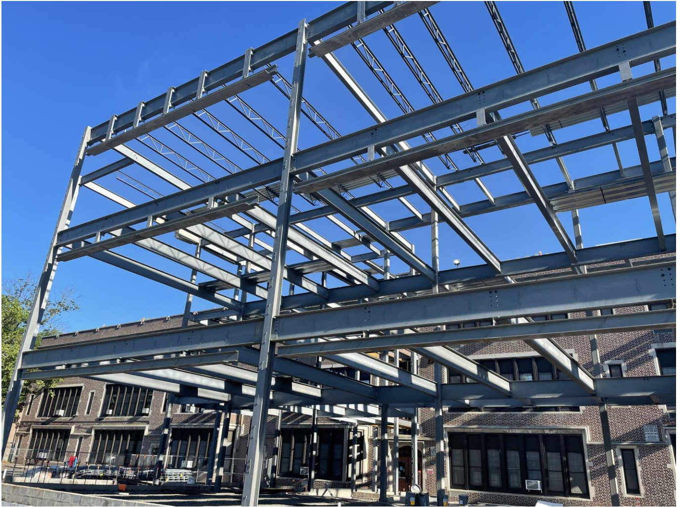
Steel erection at SME
