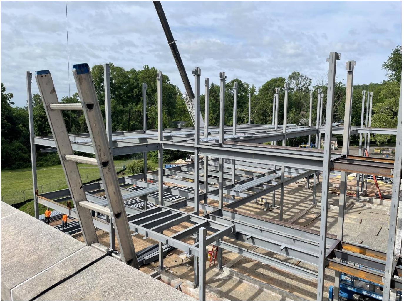
Steel erection at SME
