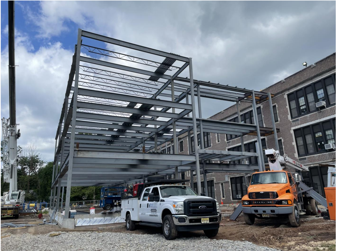
Steel erection at SME
