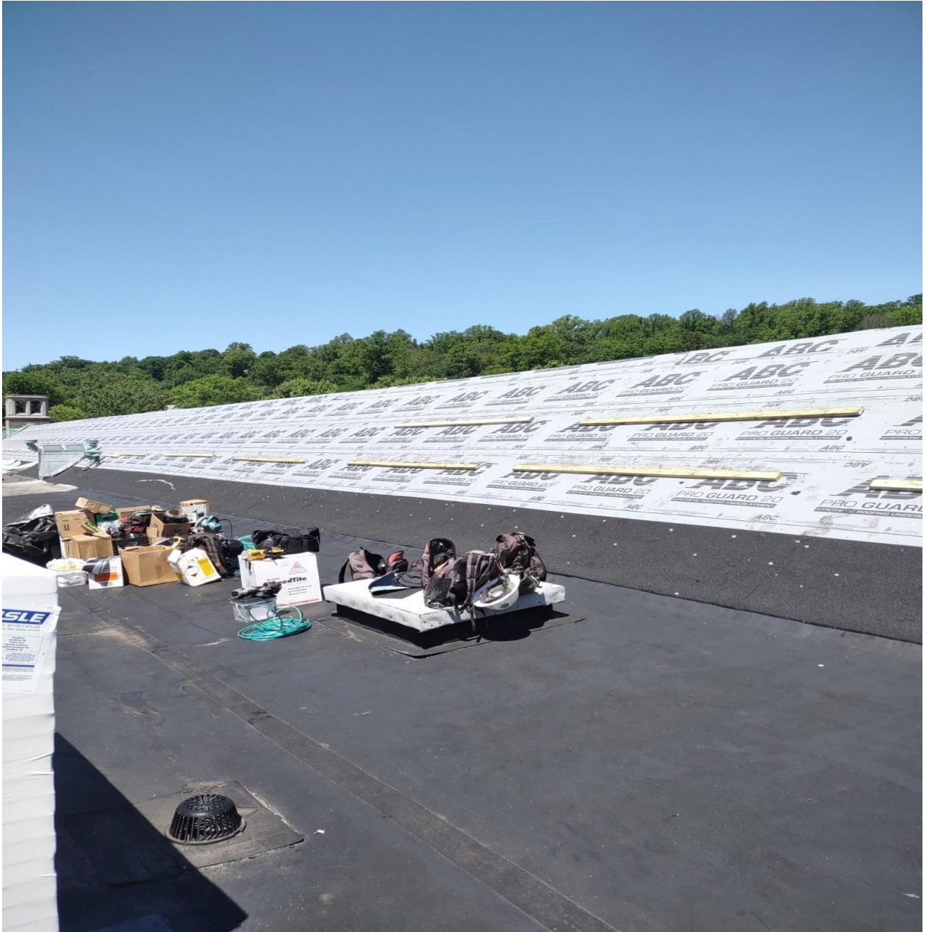
Roof replacement at SME
