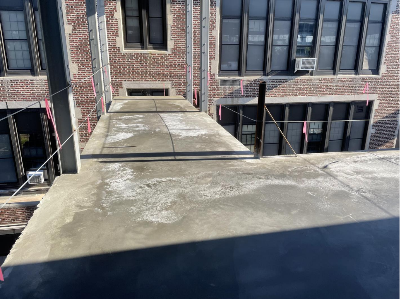
Second floor slab poured at SME
