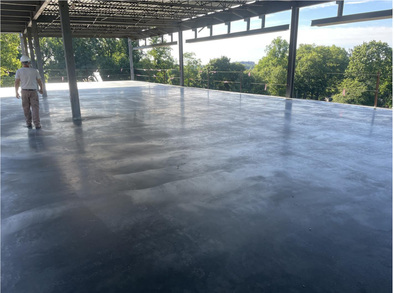
Second floor slab poured at SME
