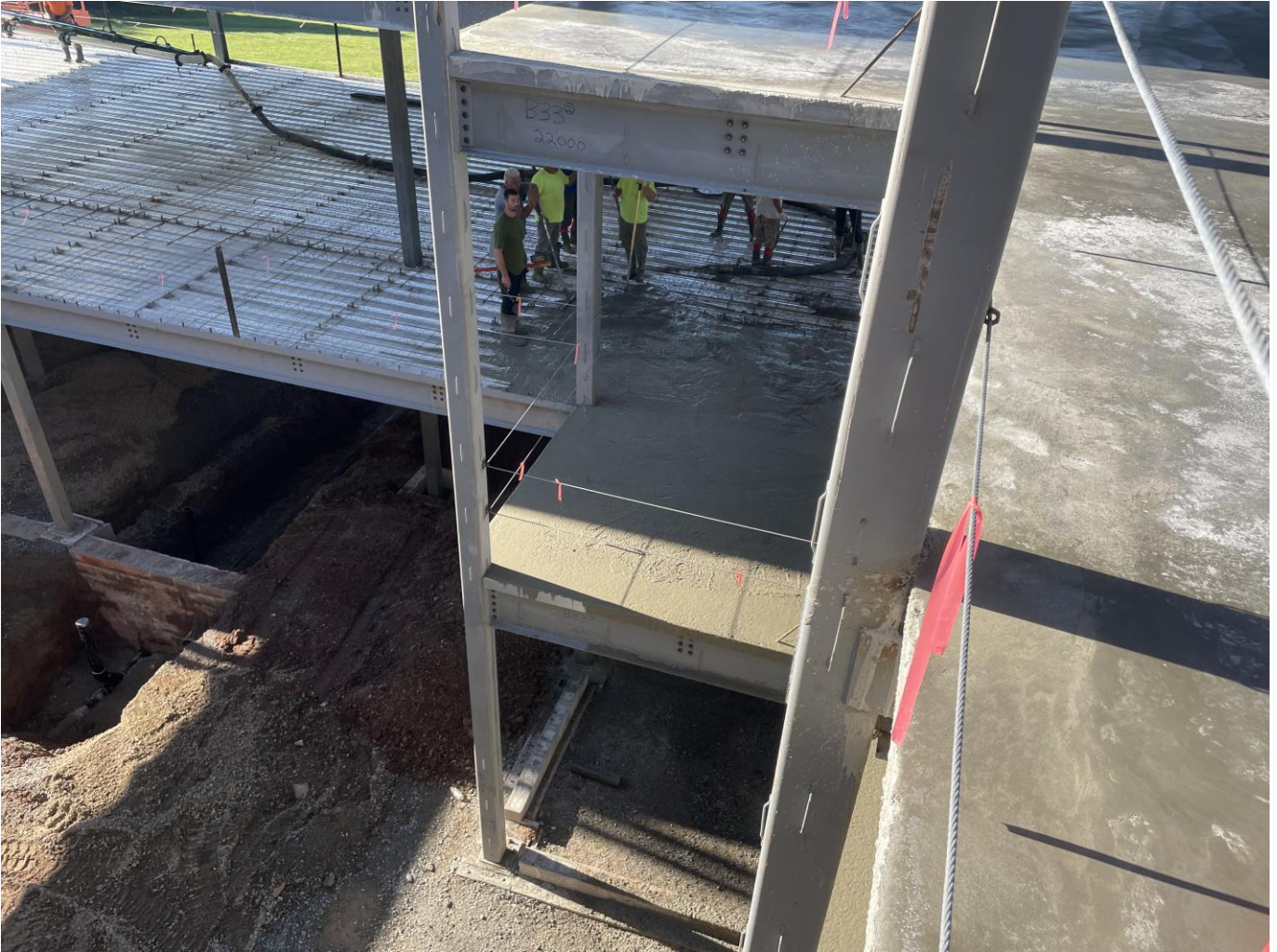
First floor slab poured at SME
