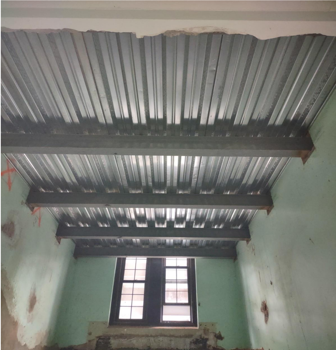
Beams and decking for proposed corridors into new addition at SME
