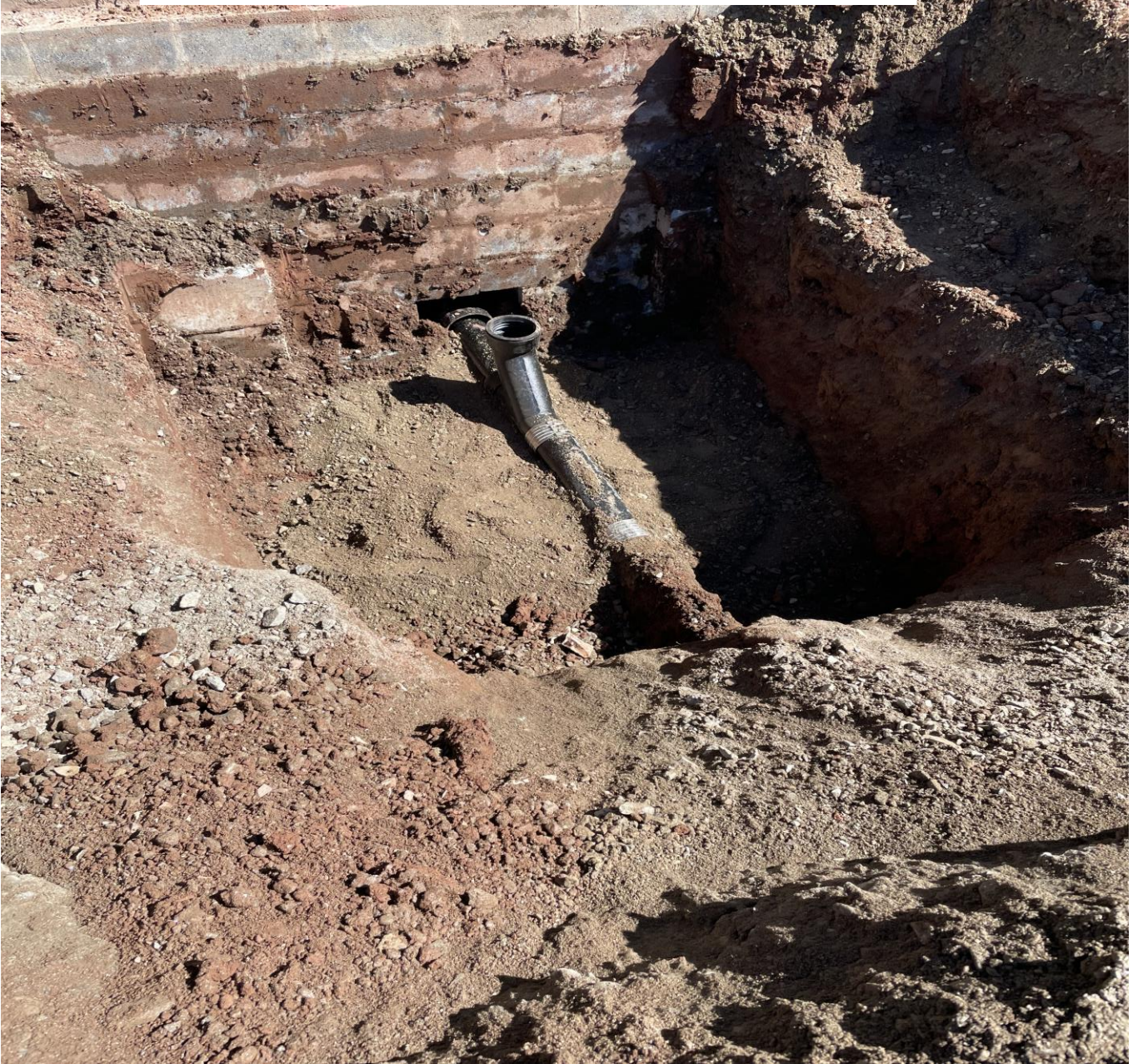
Sanitary sewer replacement at SME
