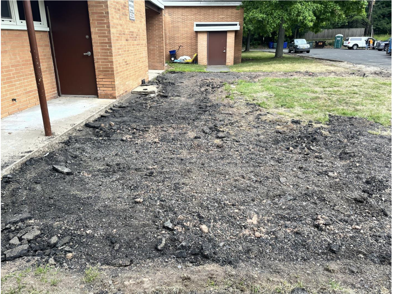
Demo of existing sidewalks at SMA
