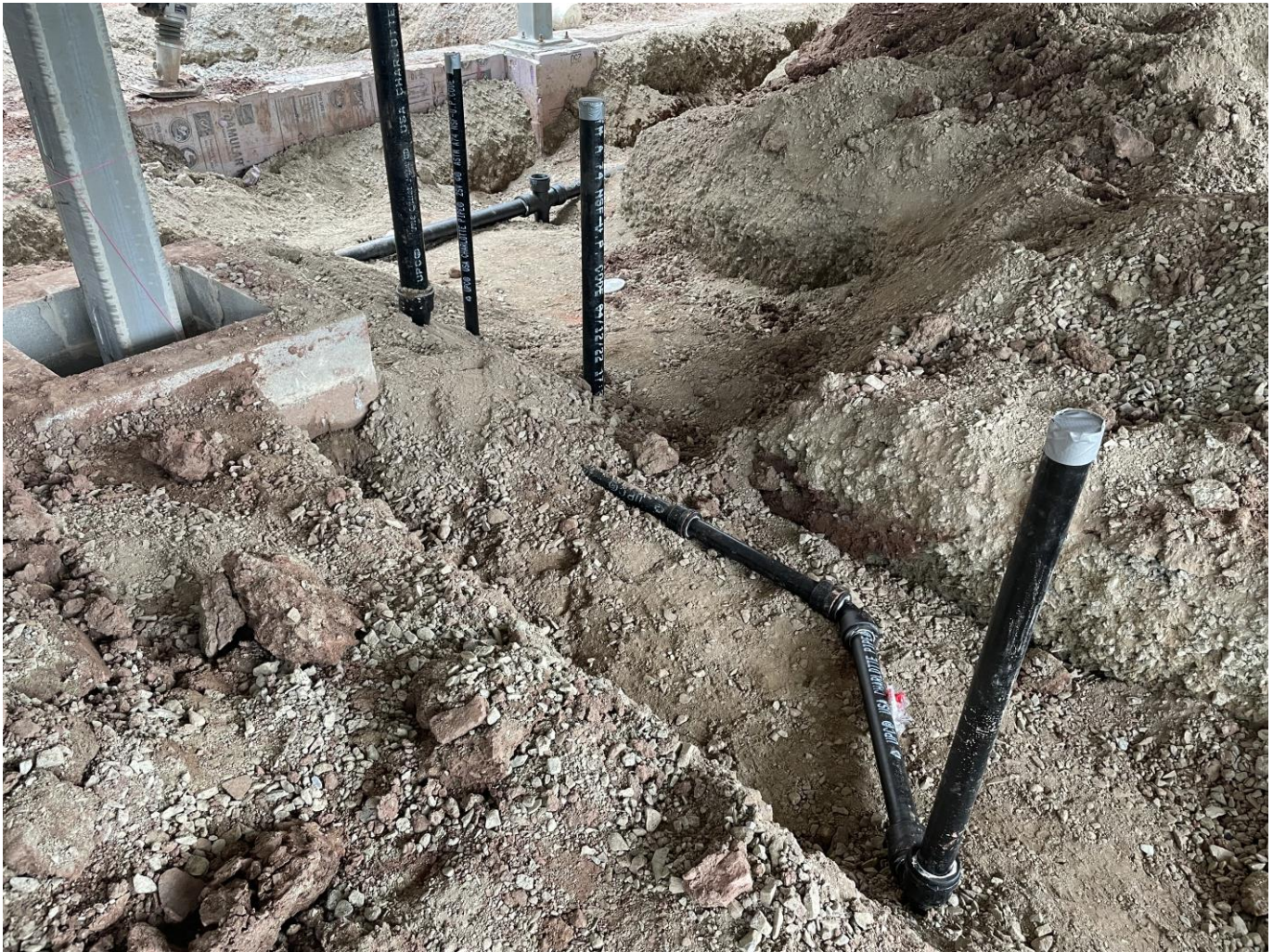
Sanitary underground at SME
