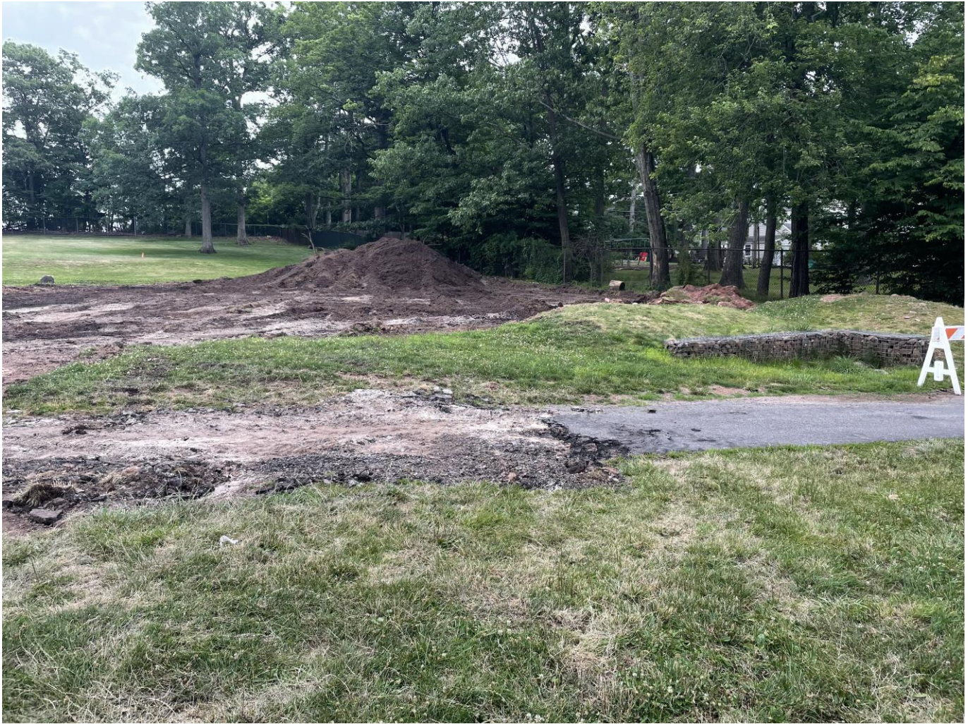
Demo of existing sidewalks and playground equipment at SMA
