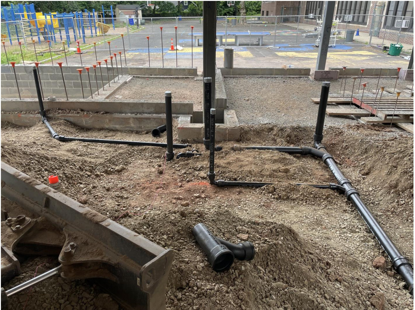
Sanitary underground at SME
