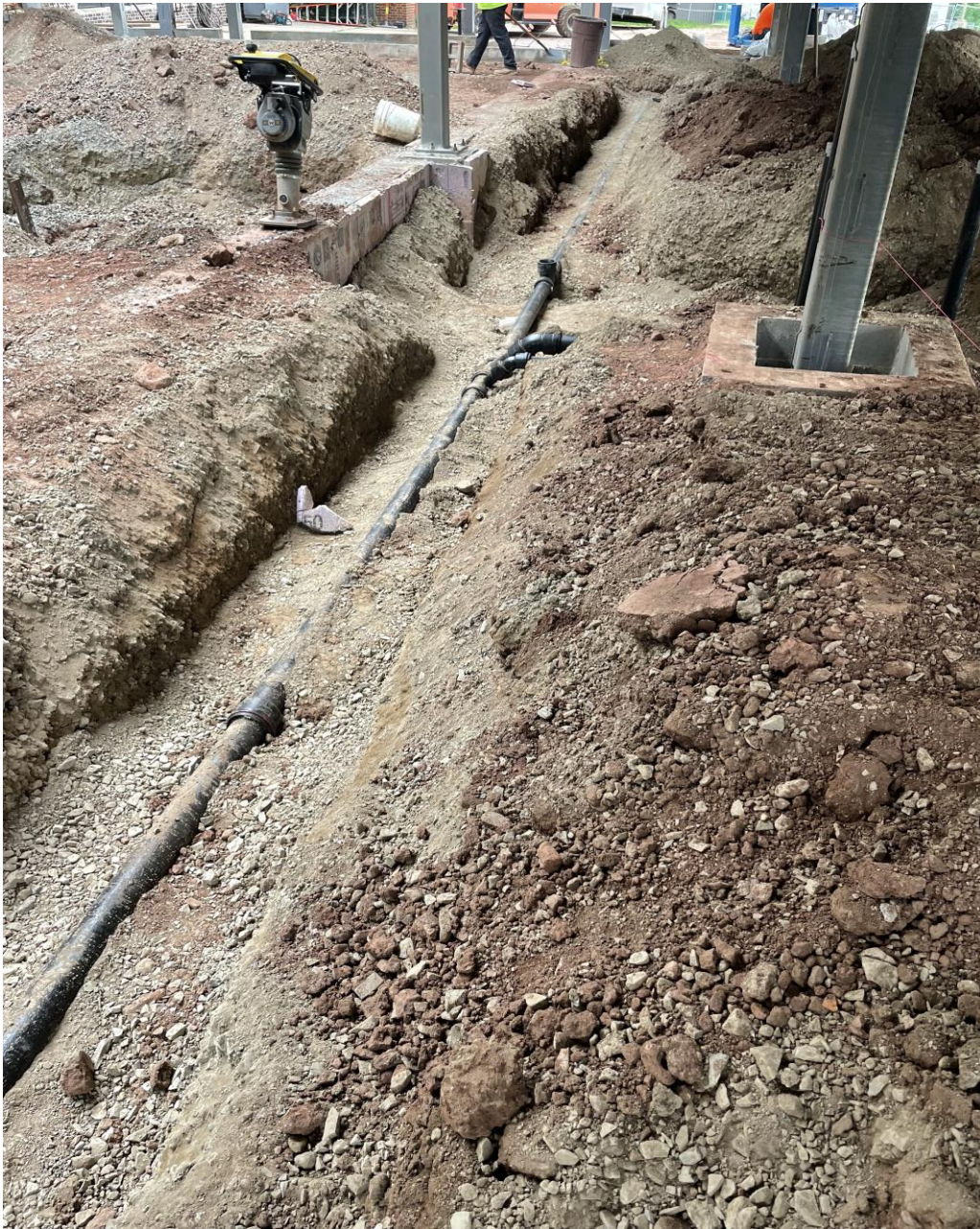
Sanitary underground at SME
