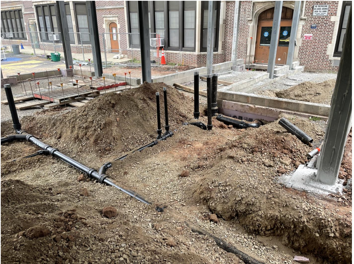
Sanitary underground at SME
