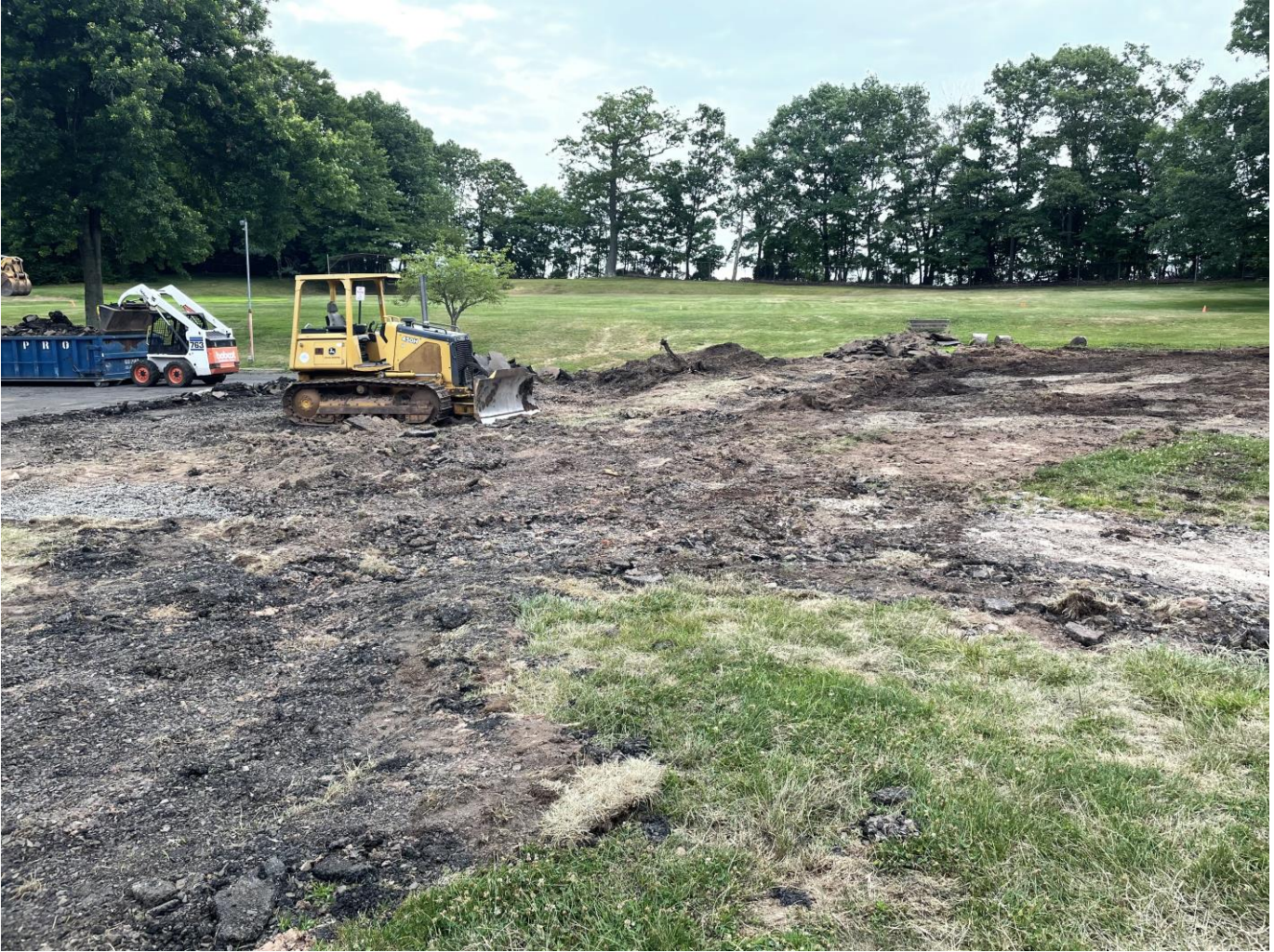
Demo of existing asphalt parking lot and curb at SMA
