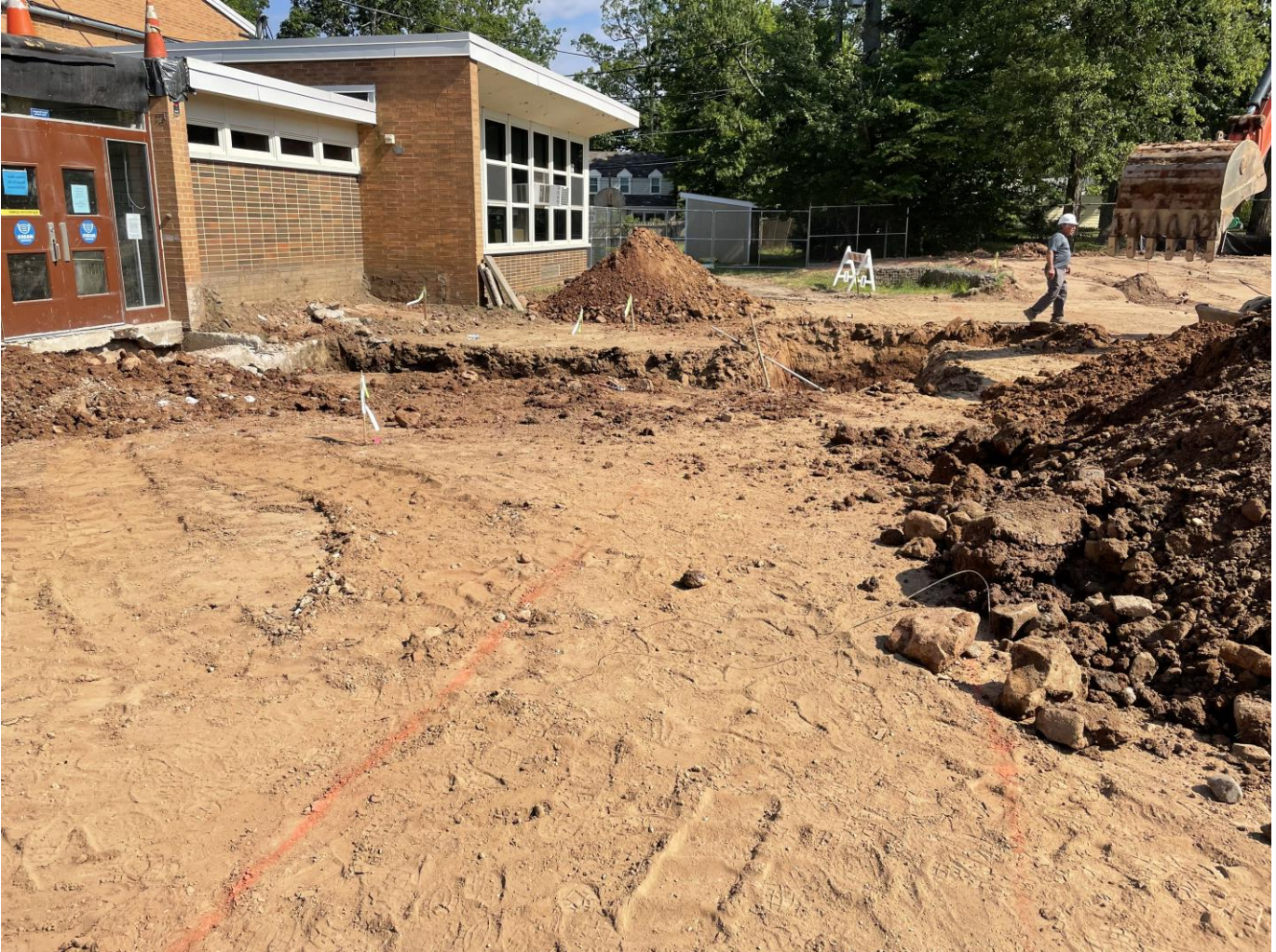
Begin excavation of footings at SMA
