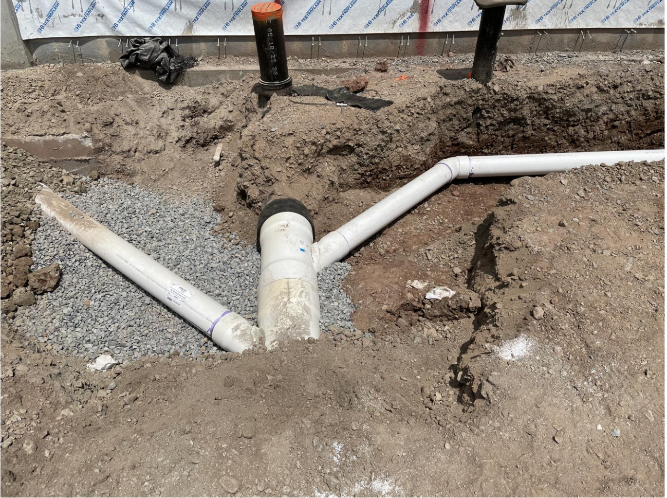
Underground drainage at SME
