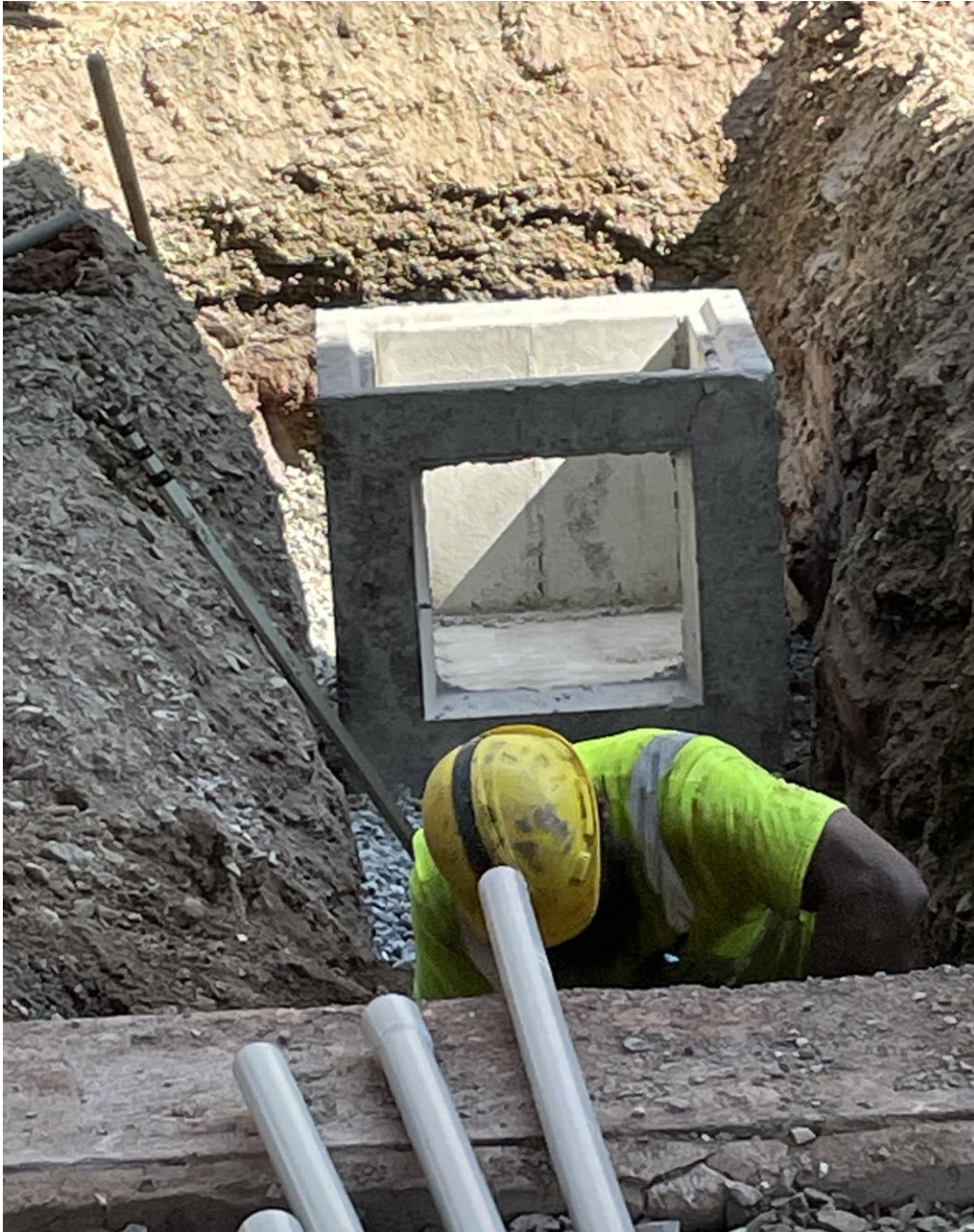
Drainage inlet in proposed courtyard at SME
