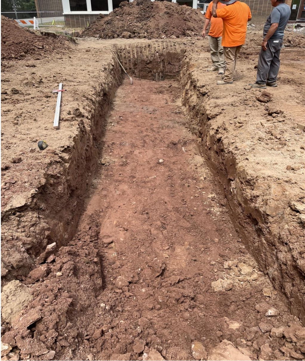
Excavation of footings at SMA for proposed addition at SMA
