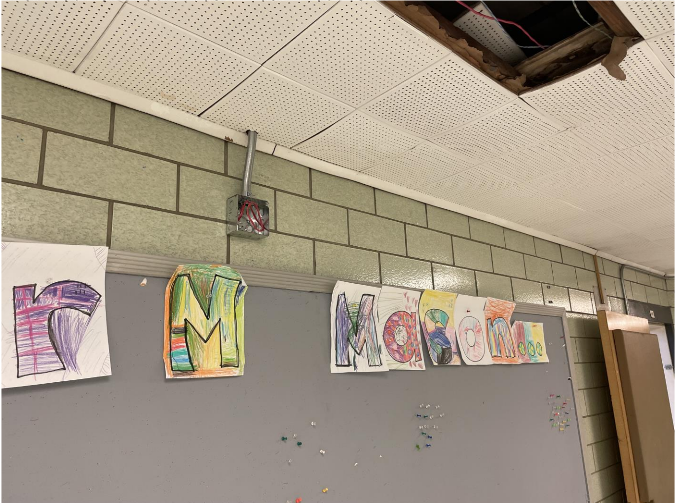
Fire Alarm rough in at SMA
