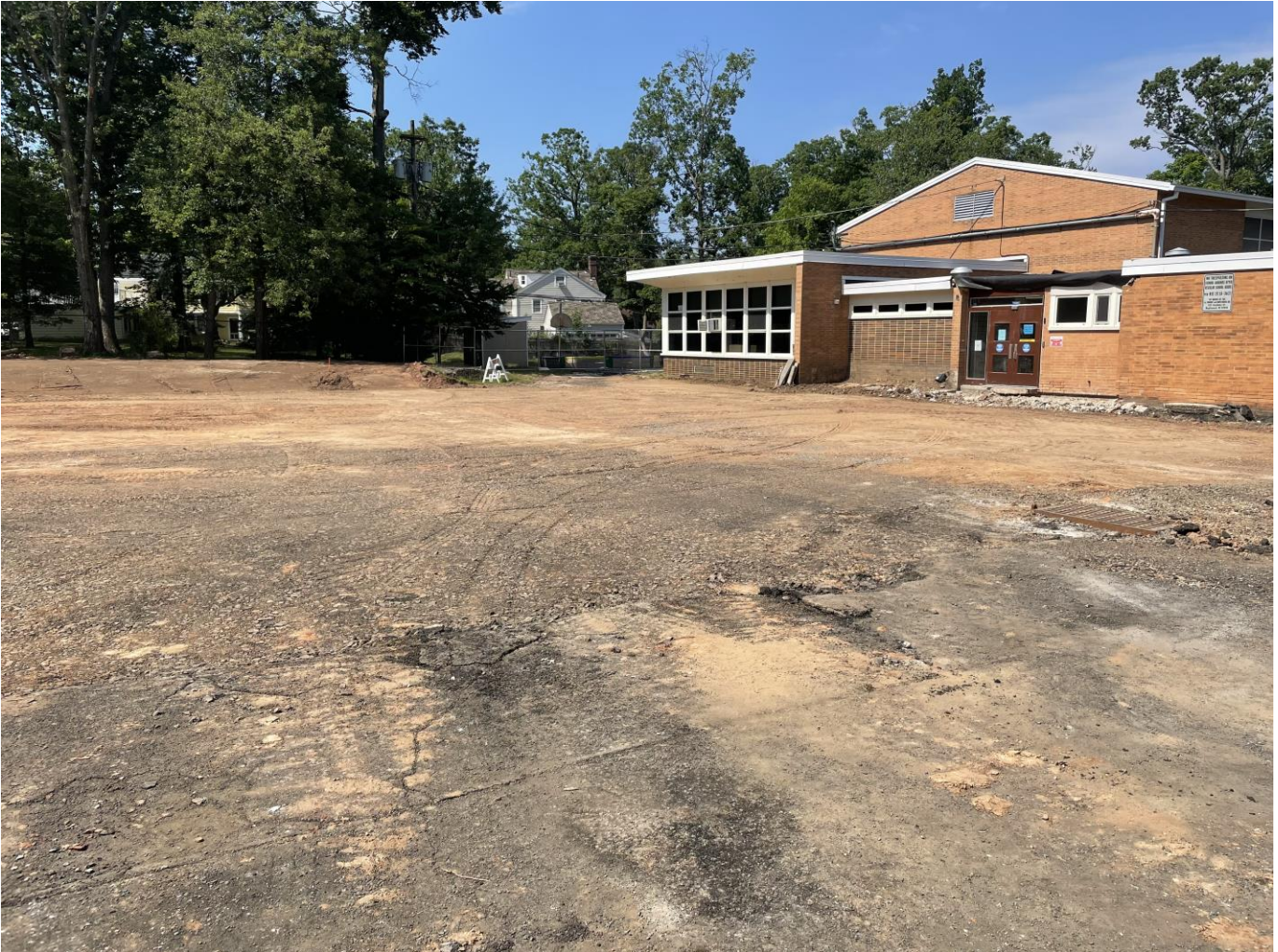
Graded addition pad at SMA
