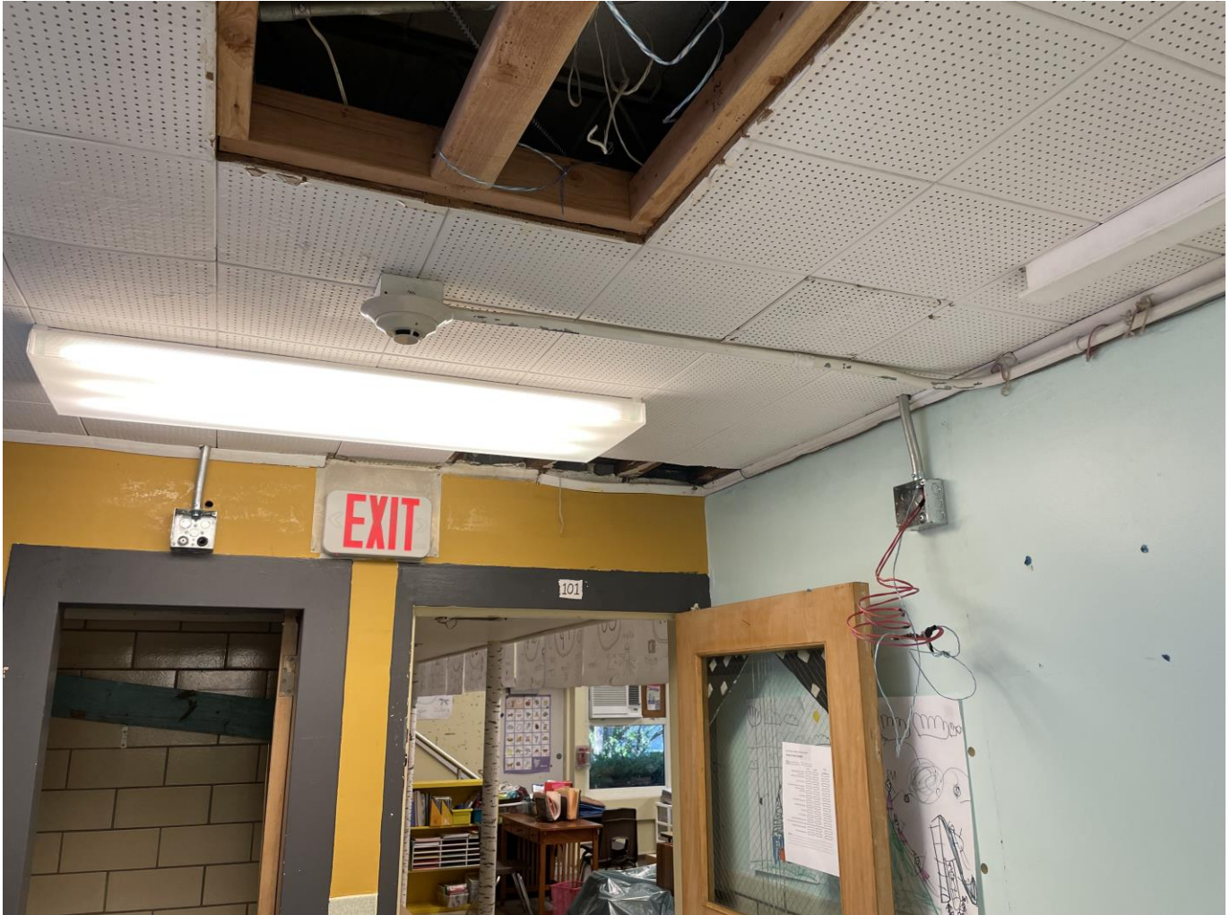
Fire Alarm rough in at SMA
