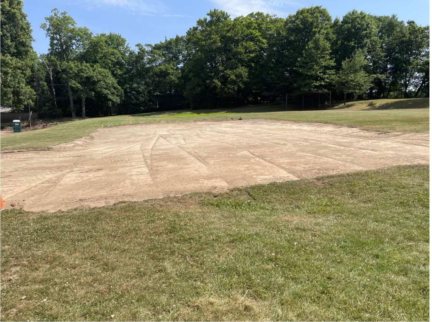
Rough graded playground area at SMA
