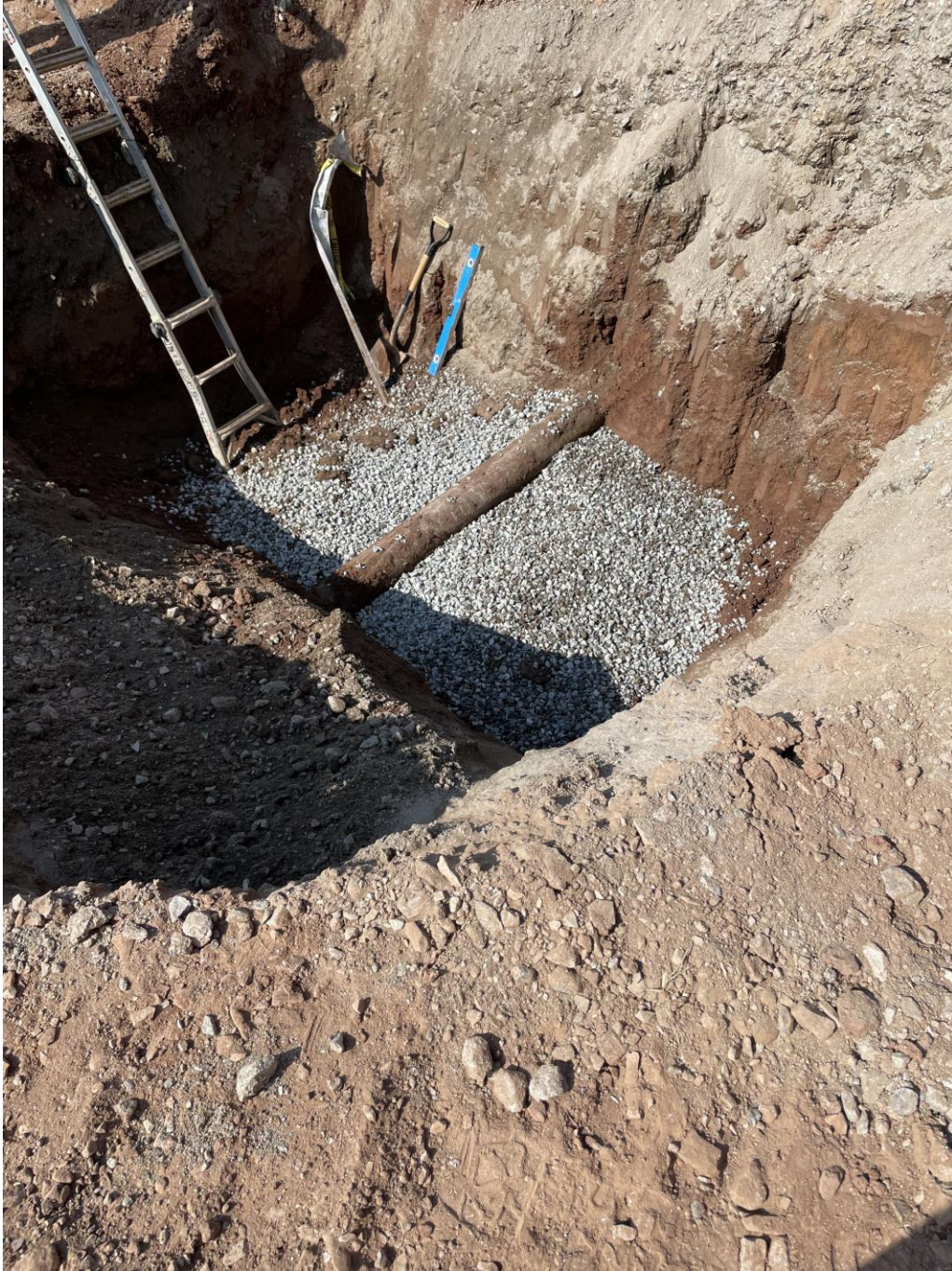
Excavate and install doghouse drainage inlet at SME
