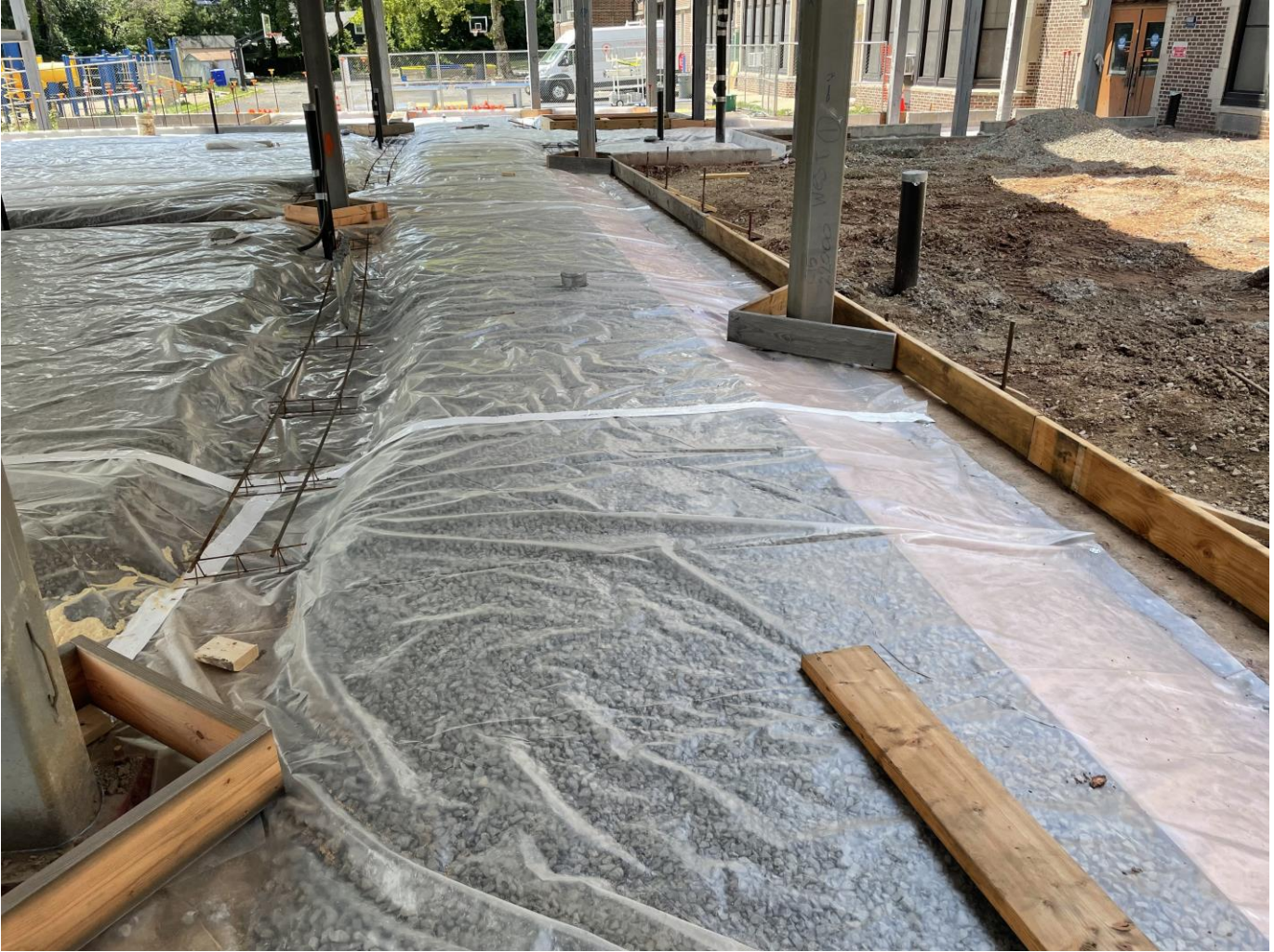
Vapor barrier and rebar for SOG at SME
