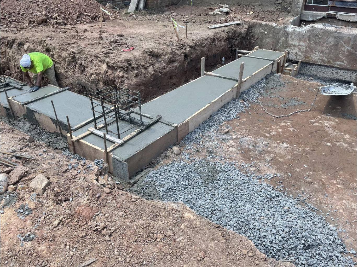
Concrete footings at SMA
