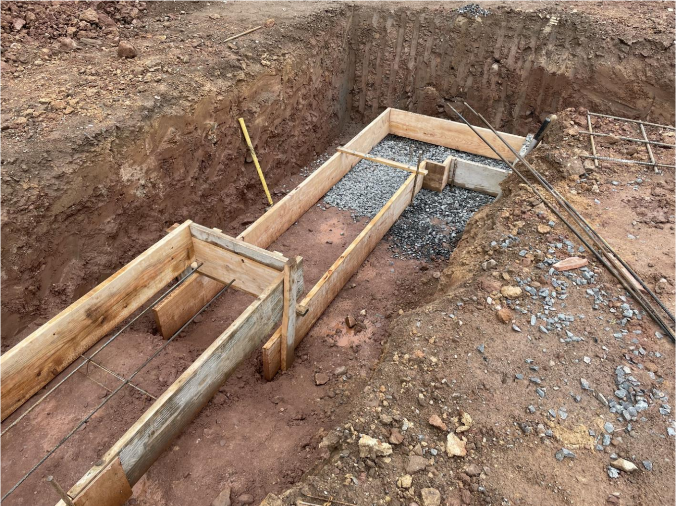
Form footings at SMA
