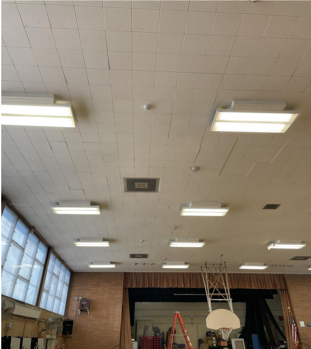
Installation of new Fire Alarm devices at SMA
