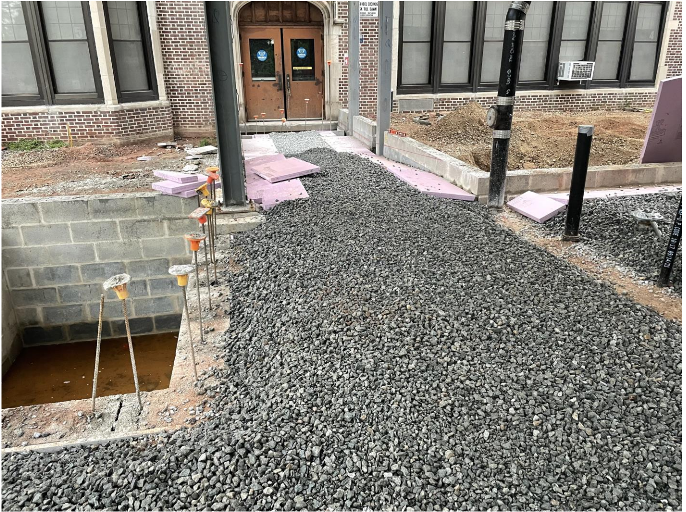
Stone sub base for SOG at SME
