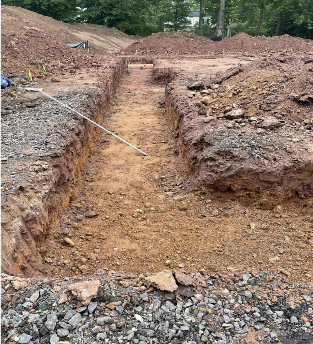
Excavate for proposed addition footings at SMA
