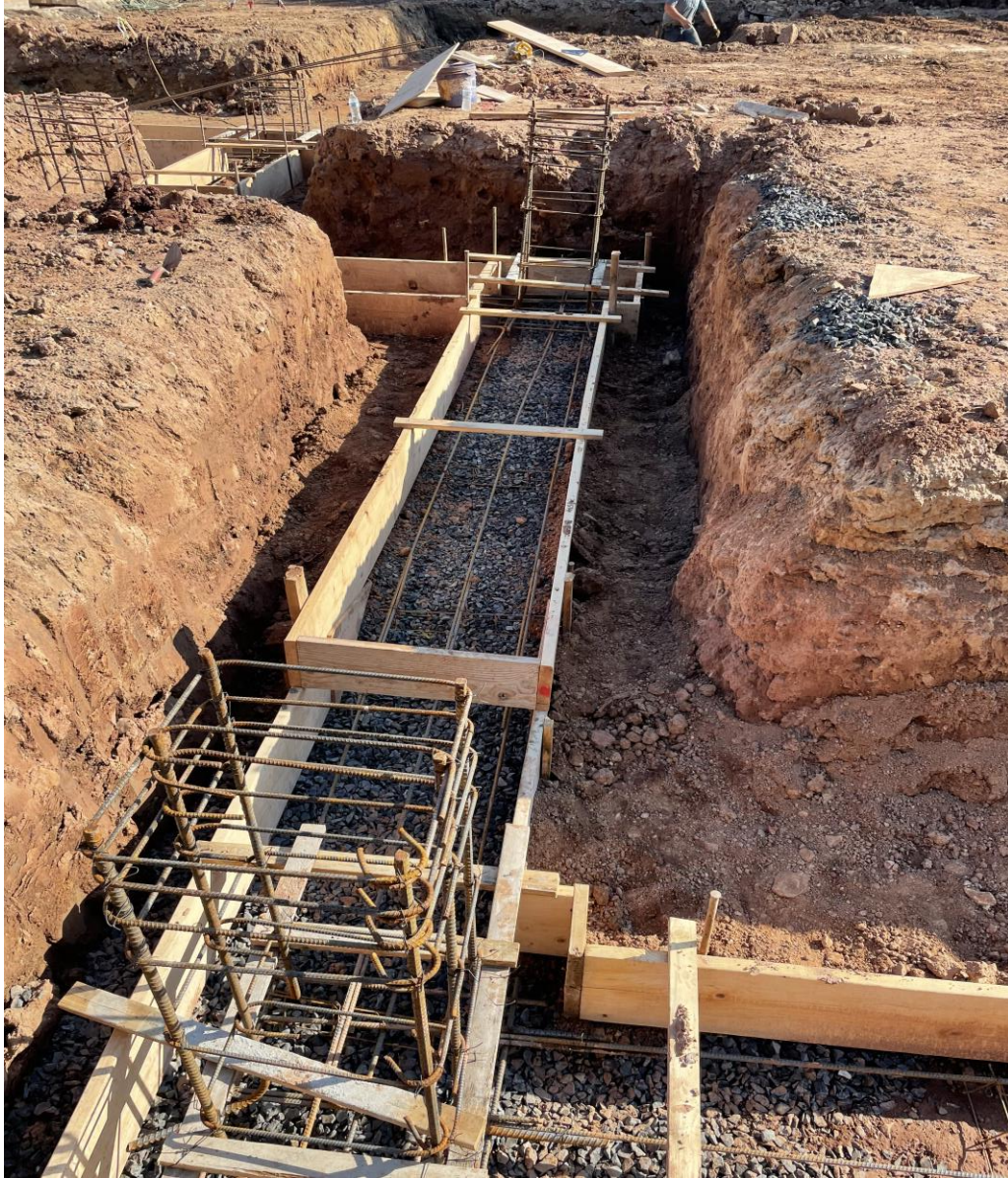
Footing forms, rebar/ Pier rebar at SMA
