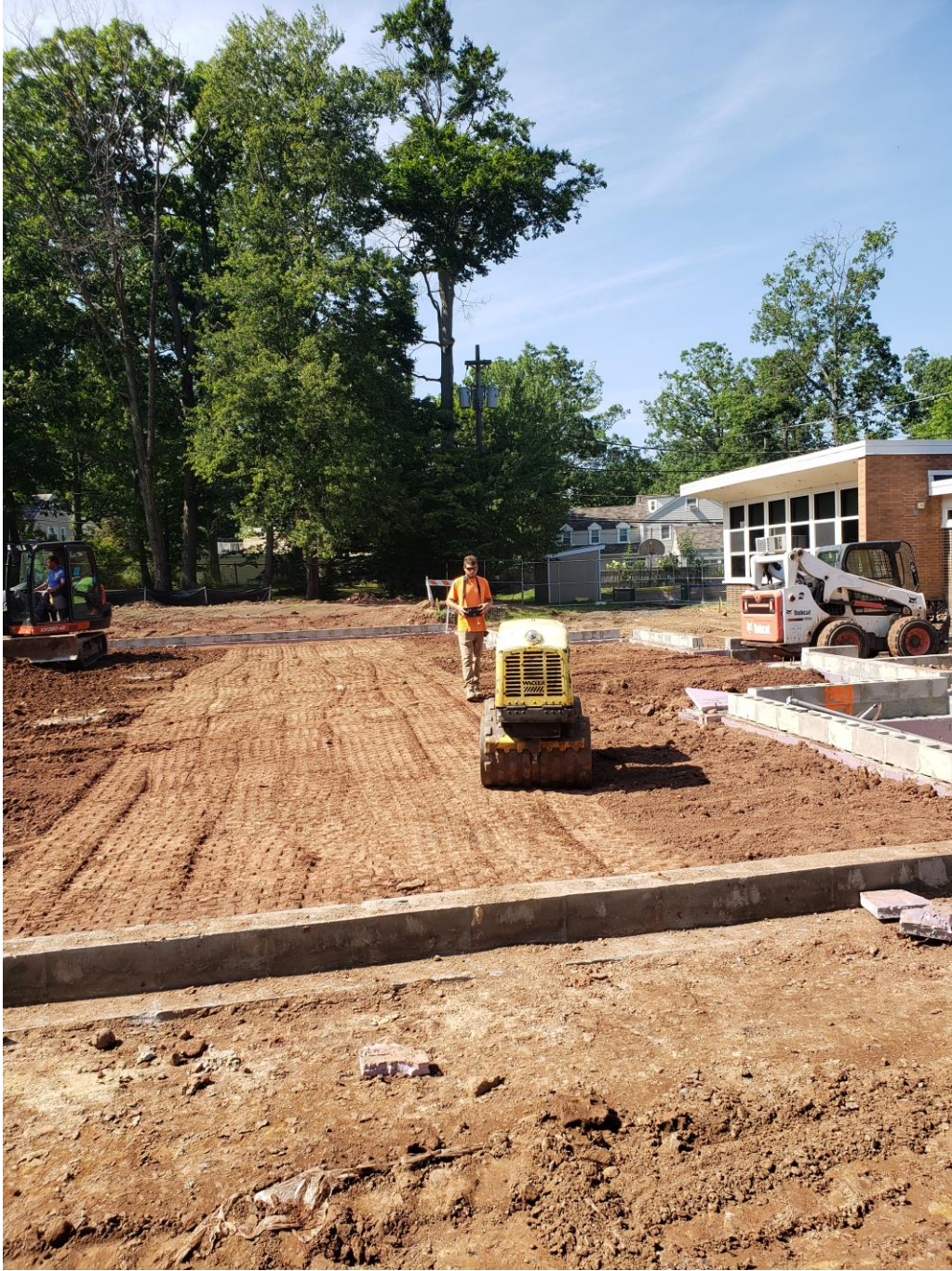
Foundation Backfill SMA
