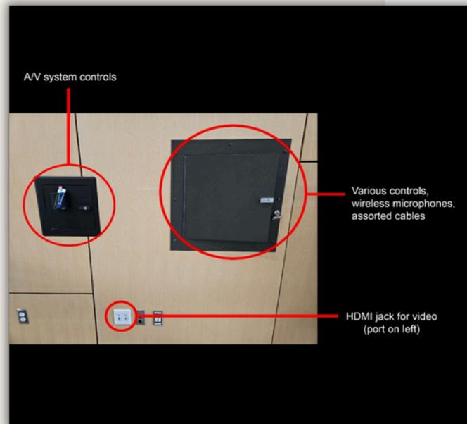
The A/V control panel is used to turn on/off the system, turn the projector on/off, control the overall volume of the system, and control the volume of individual wireless microphones. You generally only need to worry about the items mentioned below in the image. There are other controls that you should not need to use. Normally, the system is left ON, but you may need to turn it on. If so, tap the AV Plate button and this will turn the system on.
