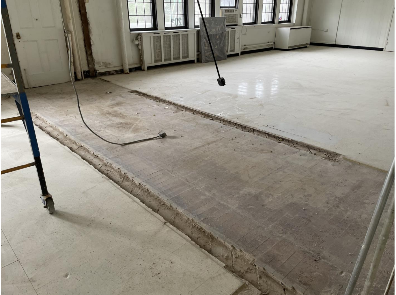
Interior wall demo at SME
