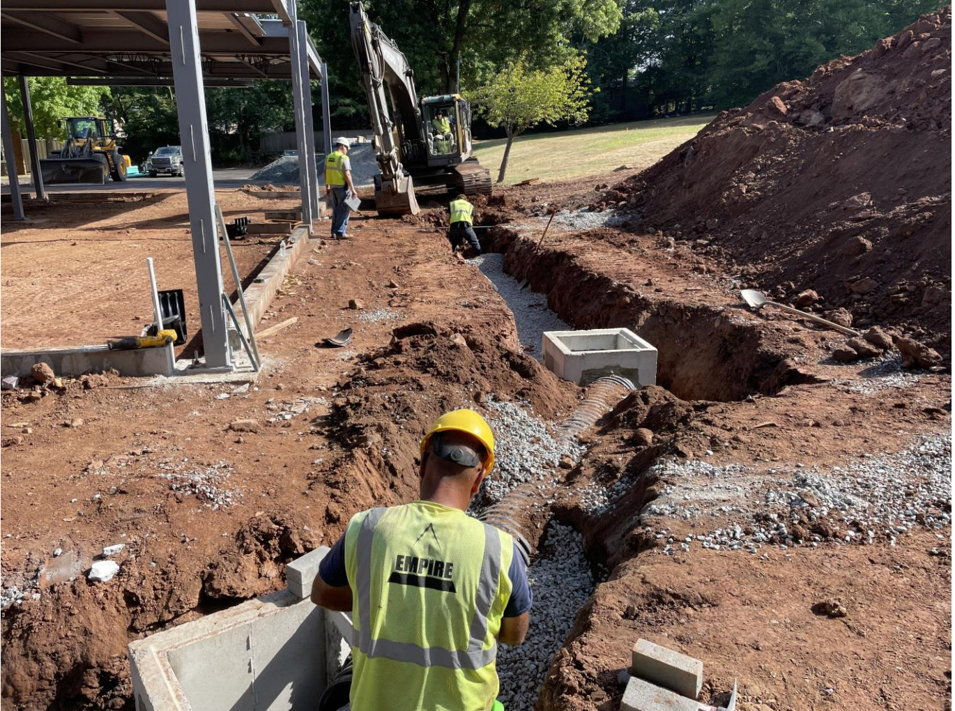
Exterior drainage at SMA
