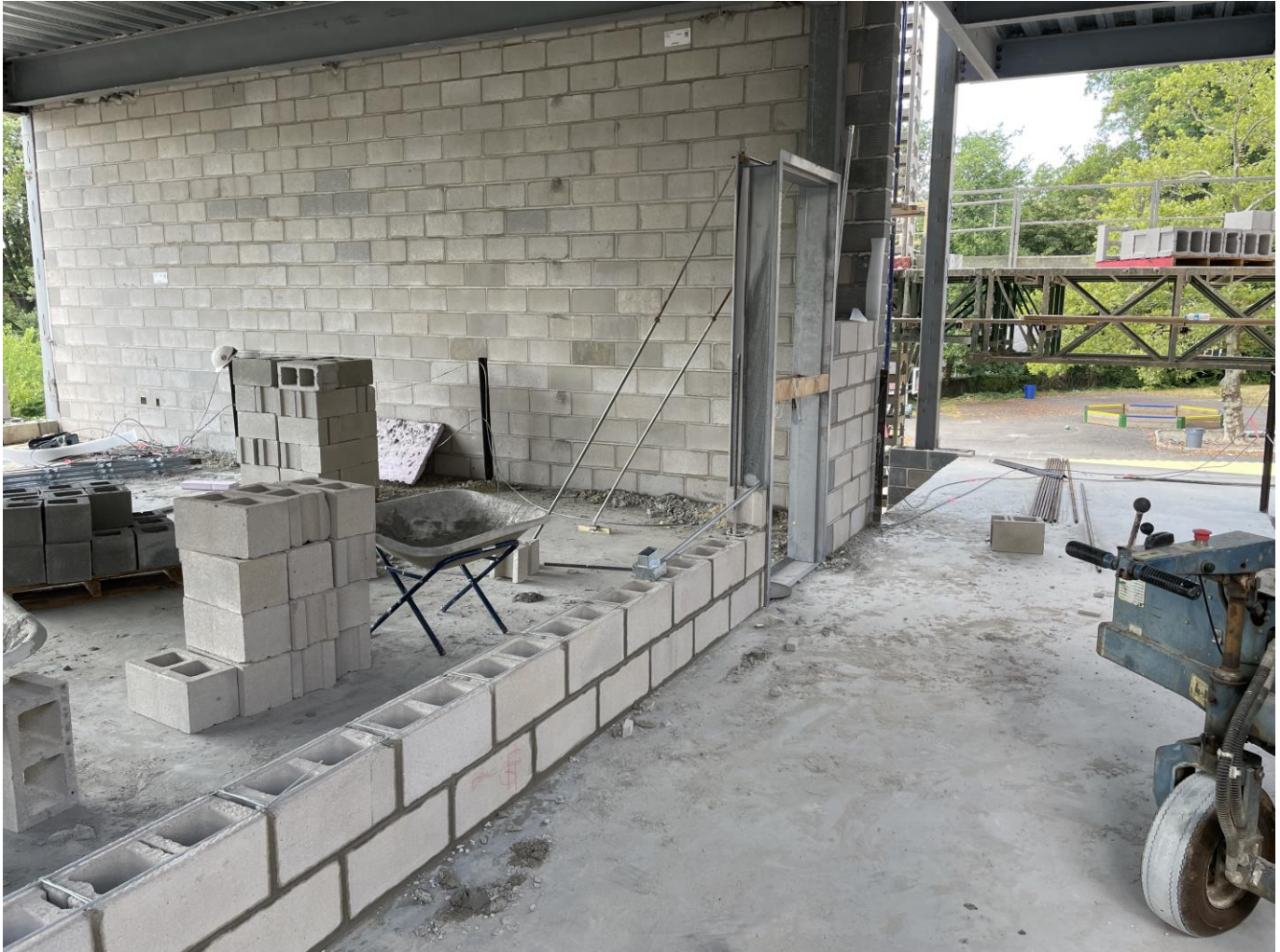
Set Door Bucks & interior block work at SME
