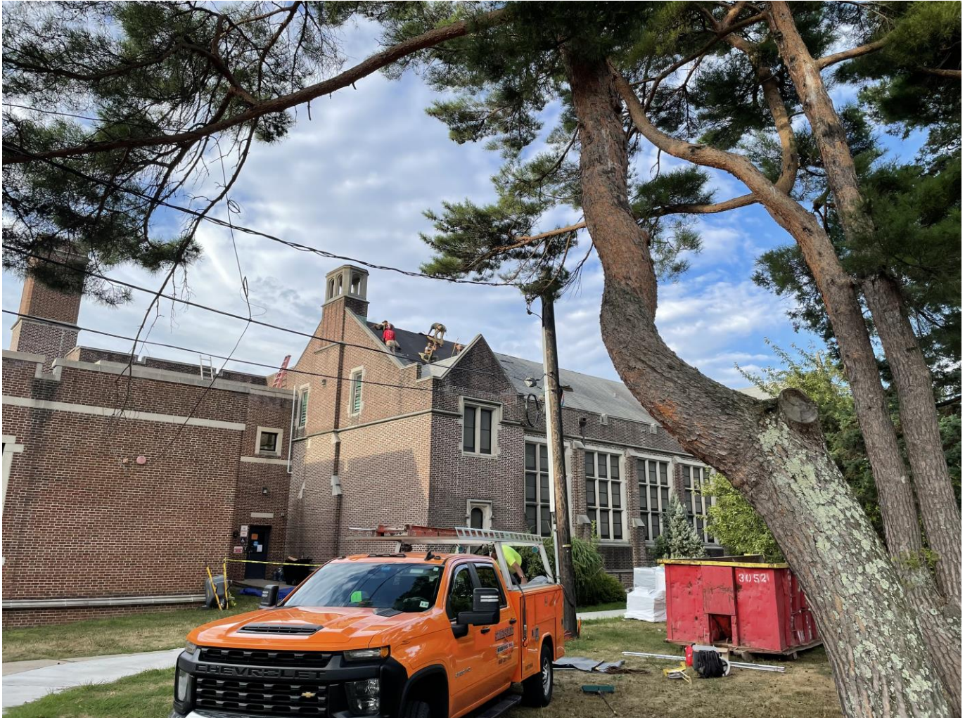
Roof demo and re-roof at SME
