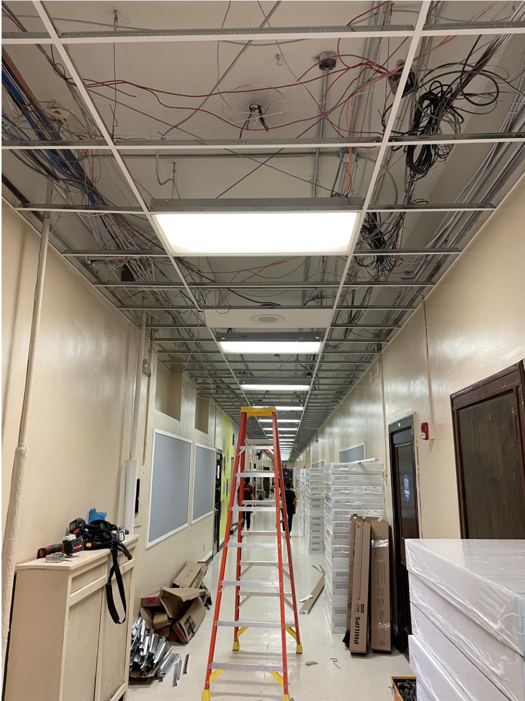
Continue ceiling grid in corridors at SME
