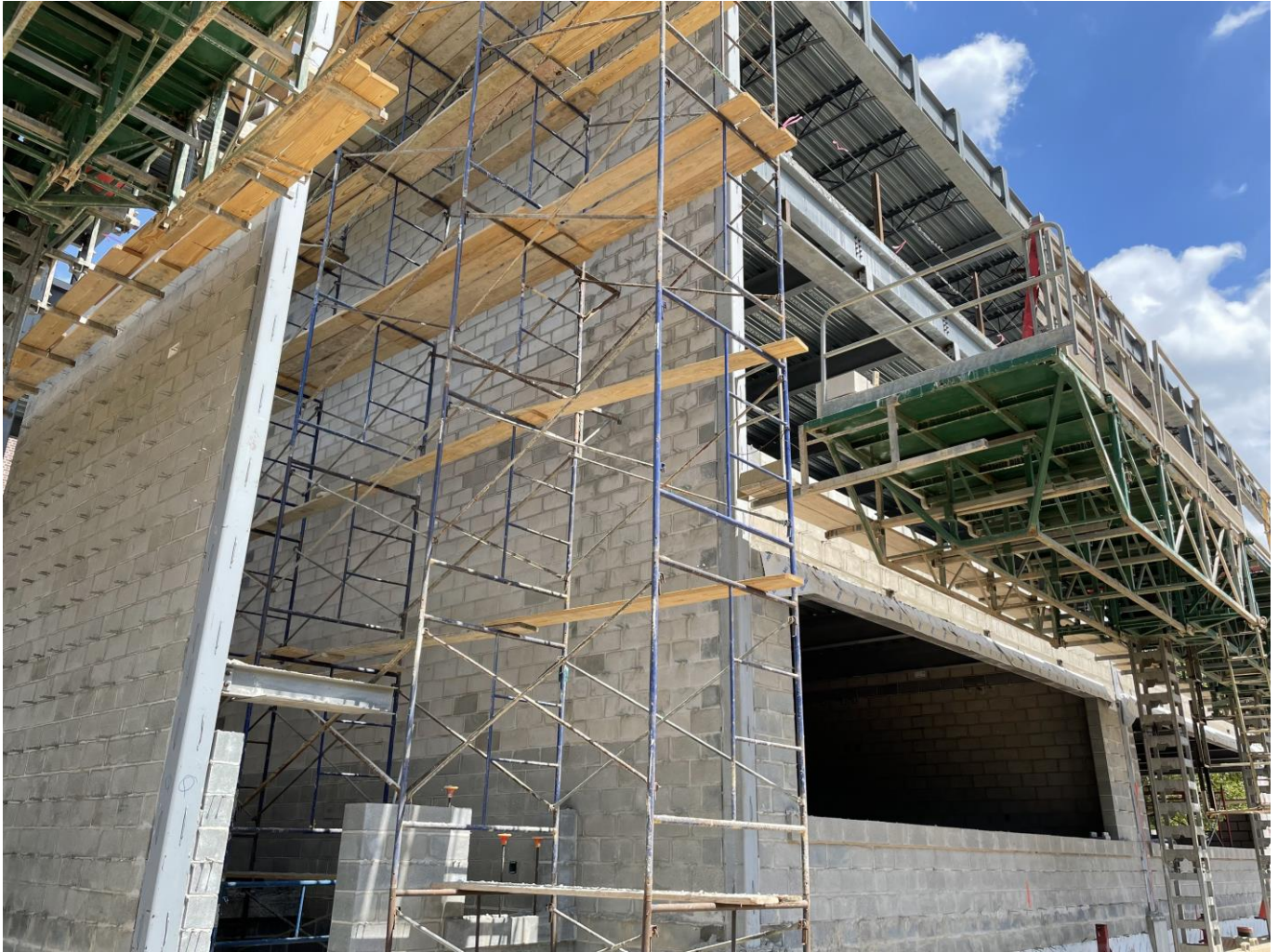
Exterior blockwork SME
