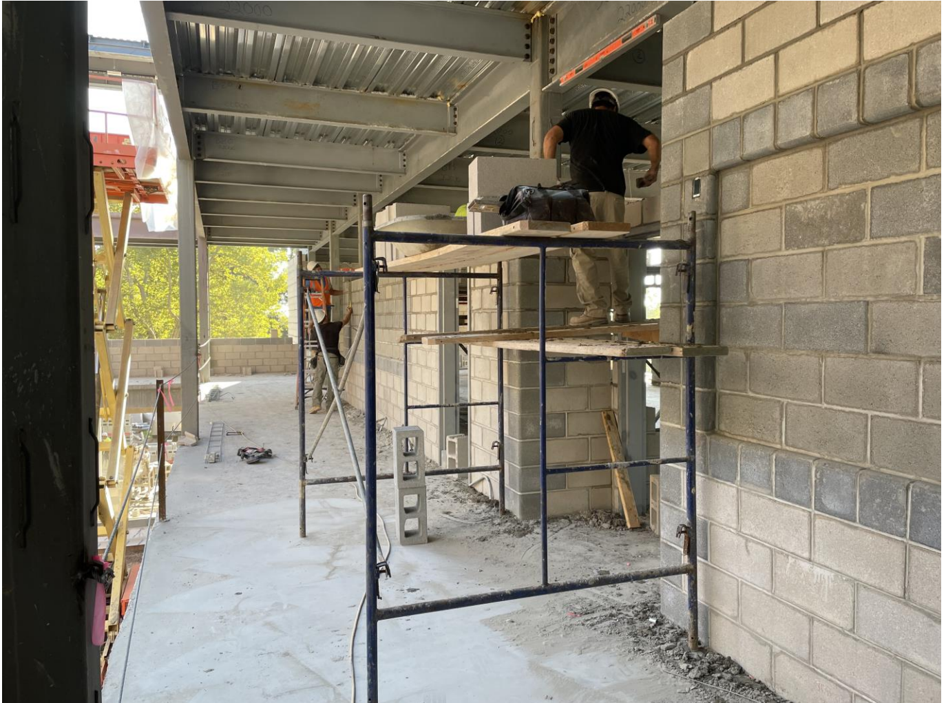
Interior block work at SME
