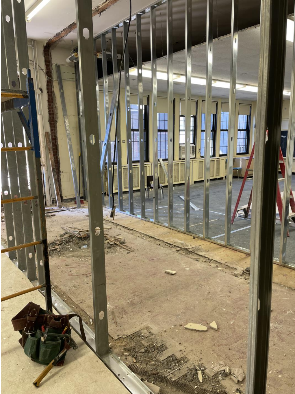
Interior wall construction for proposed connecting corridor at SME
