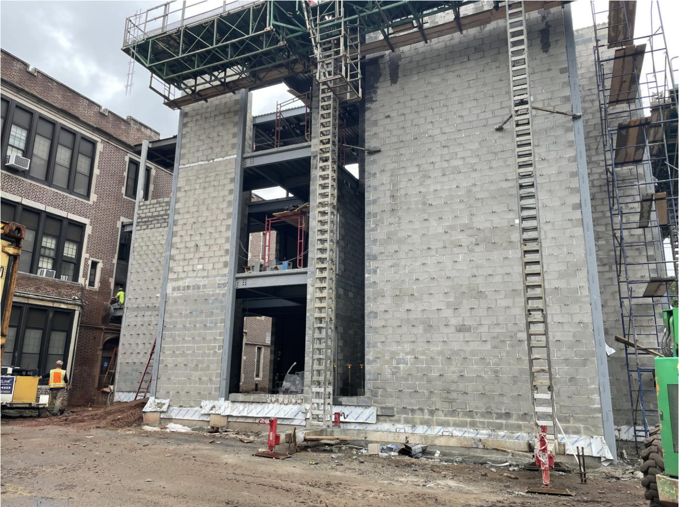
Exterior block work at SME
