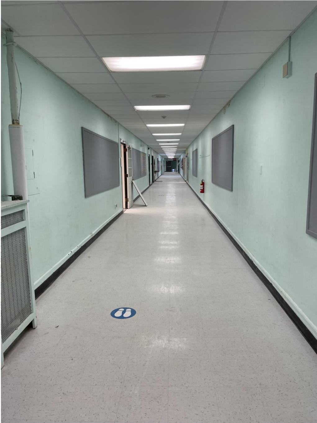
Installed ceiling tiles in corridors at SME
