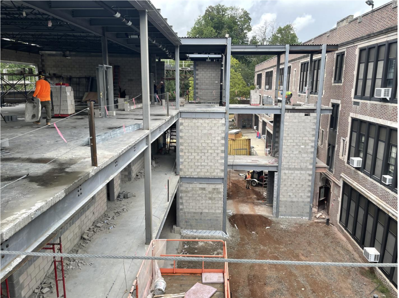
Interior/exterior block work at SME
