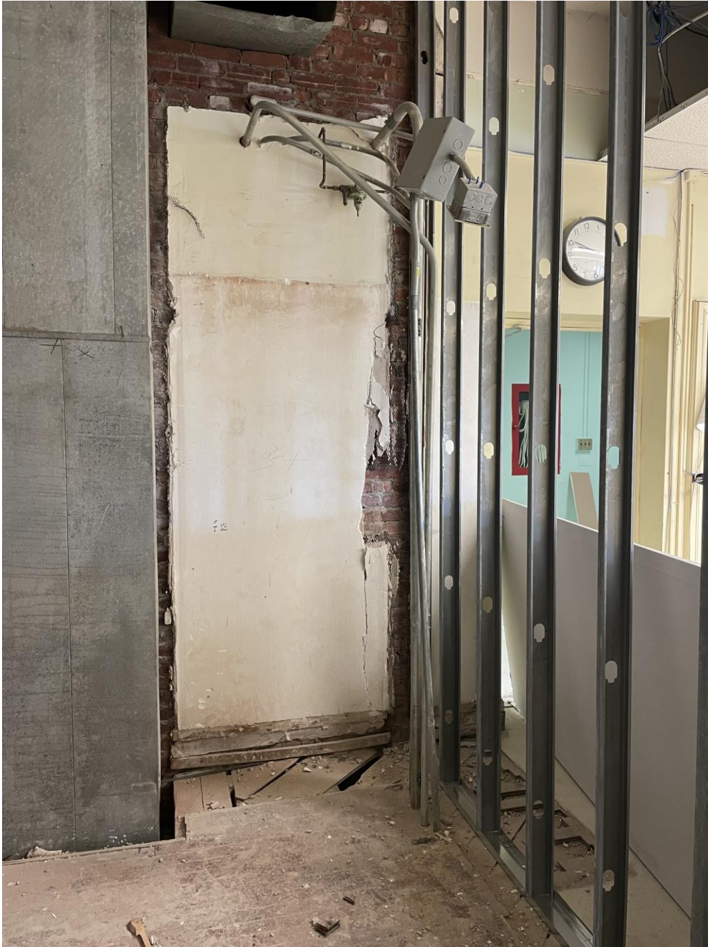
Framing for new corridor walls at SME
