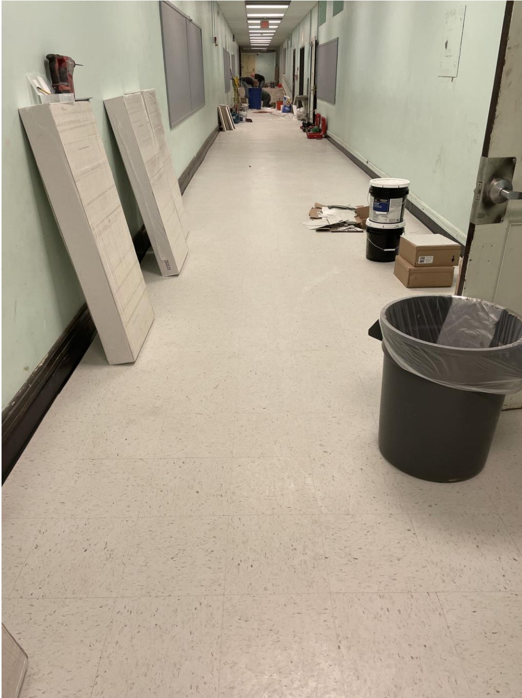
Ground floor corridor floor tile at SME
