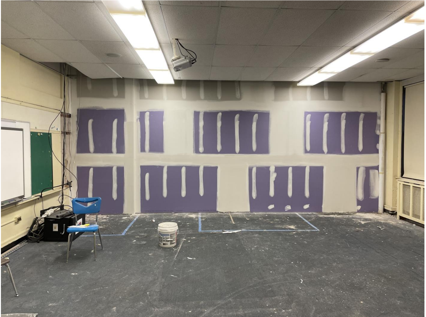
New corridor partition walls at SME
