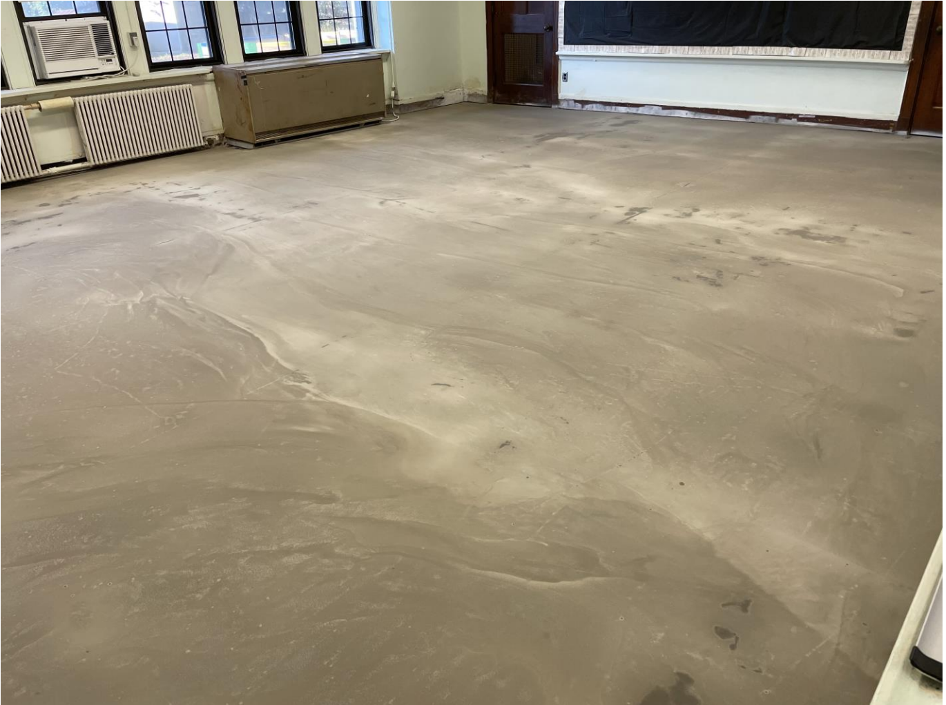
Ardex self leveling for floor in room 8 at SME
