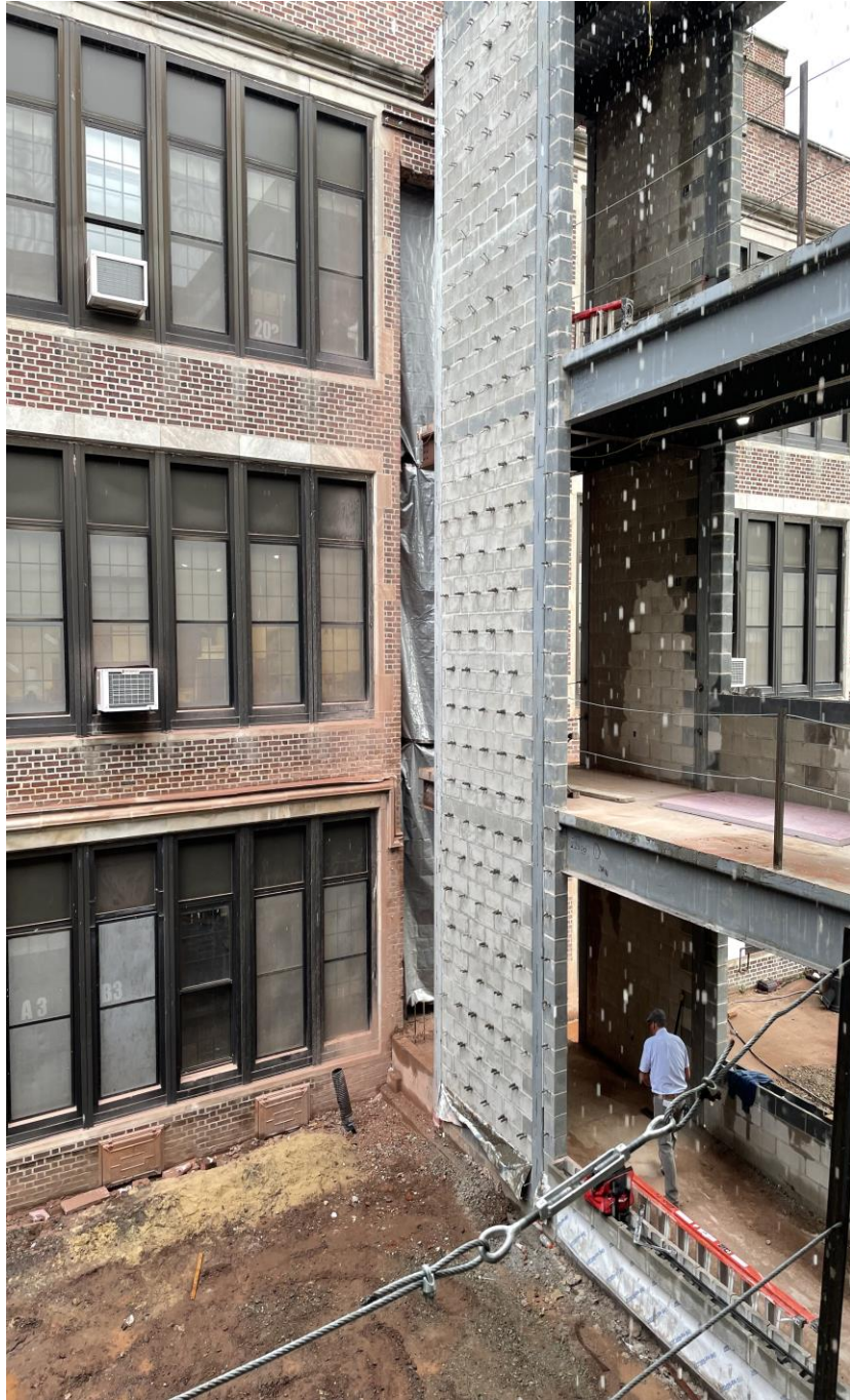
Demo of existing brick wall for proposed corridor at SME
