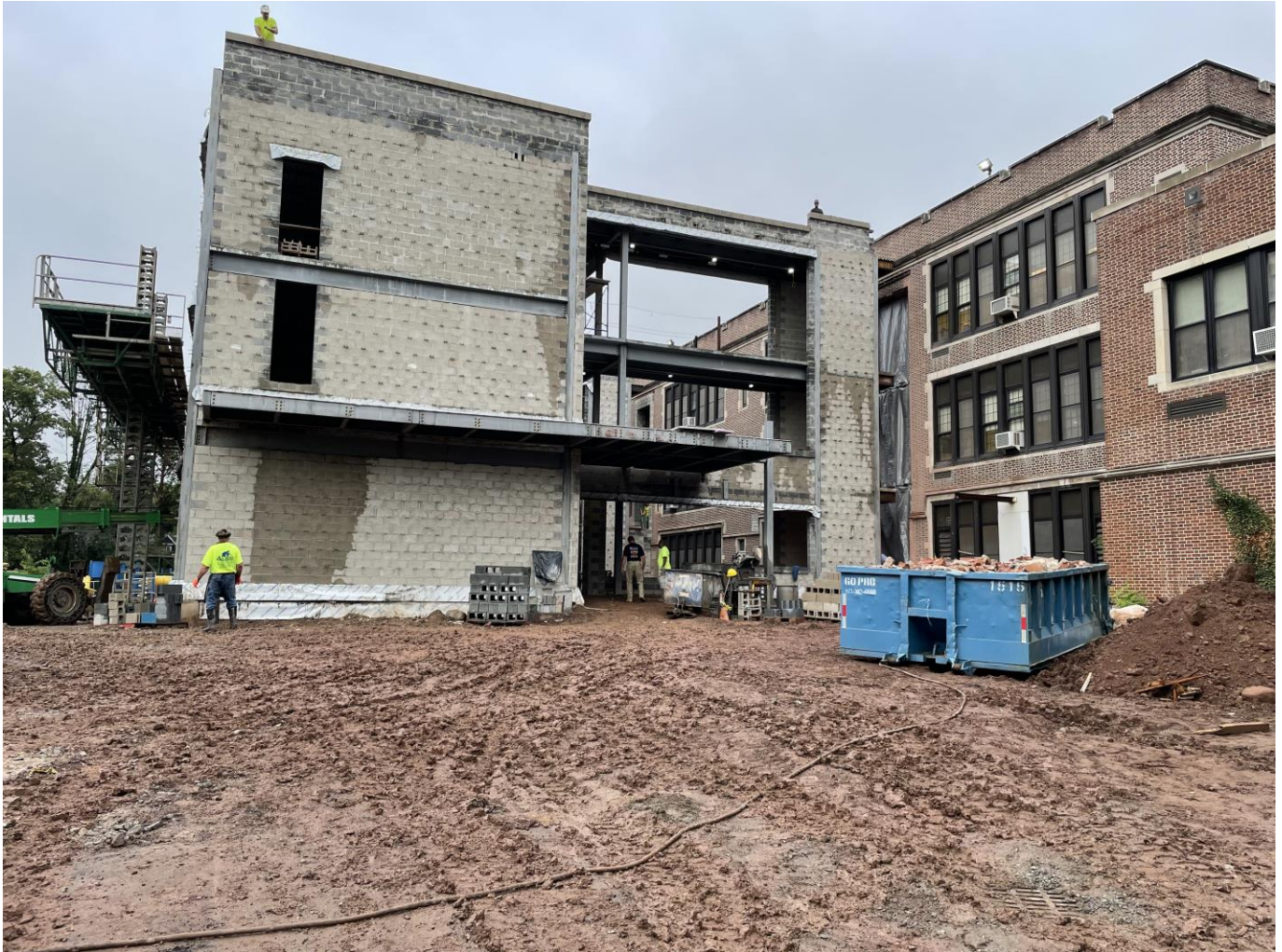
Exterior block work at SME
