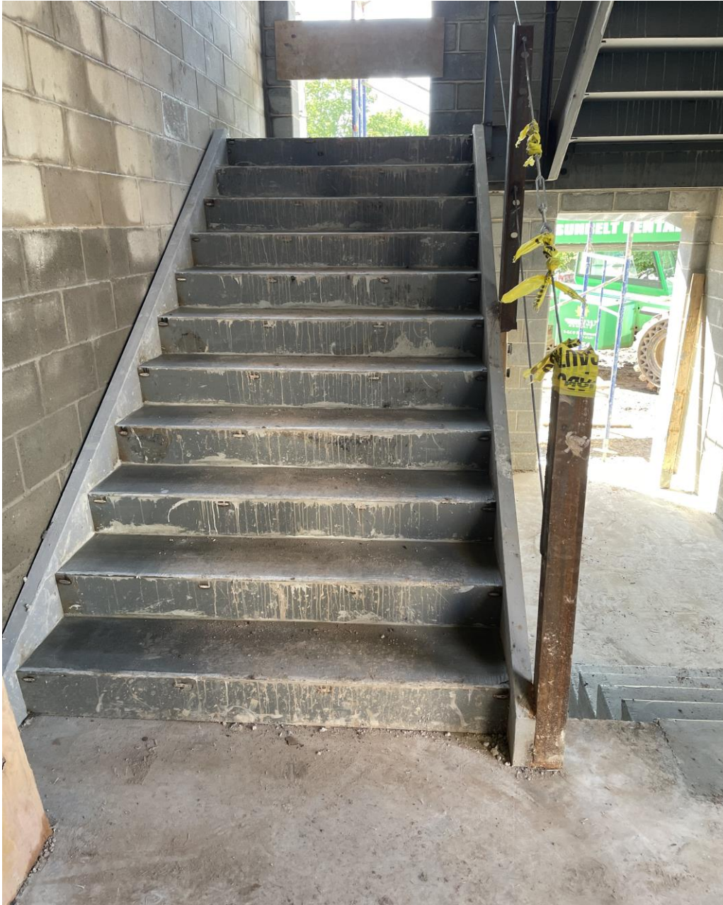
Poured concrete for stairs at SME
