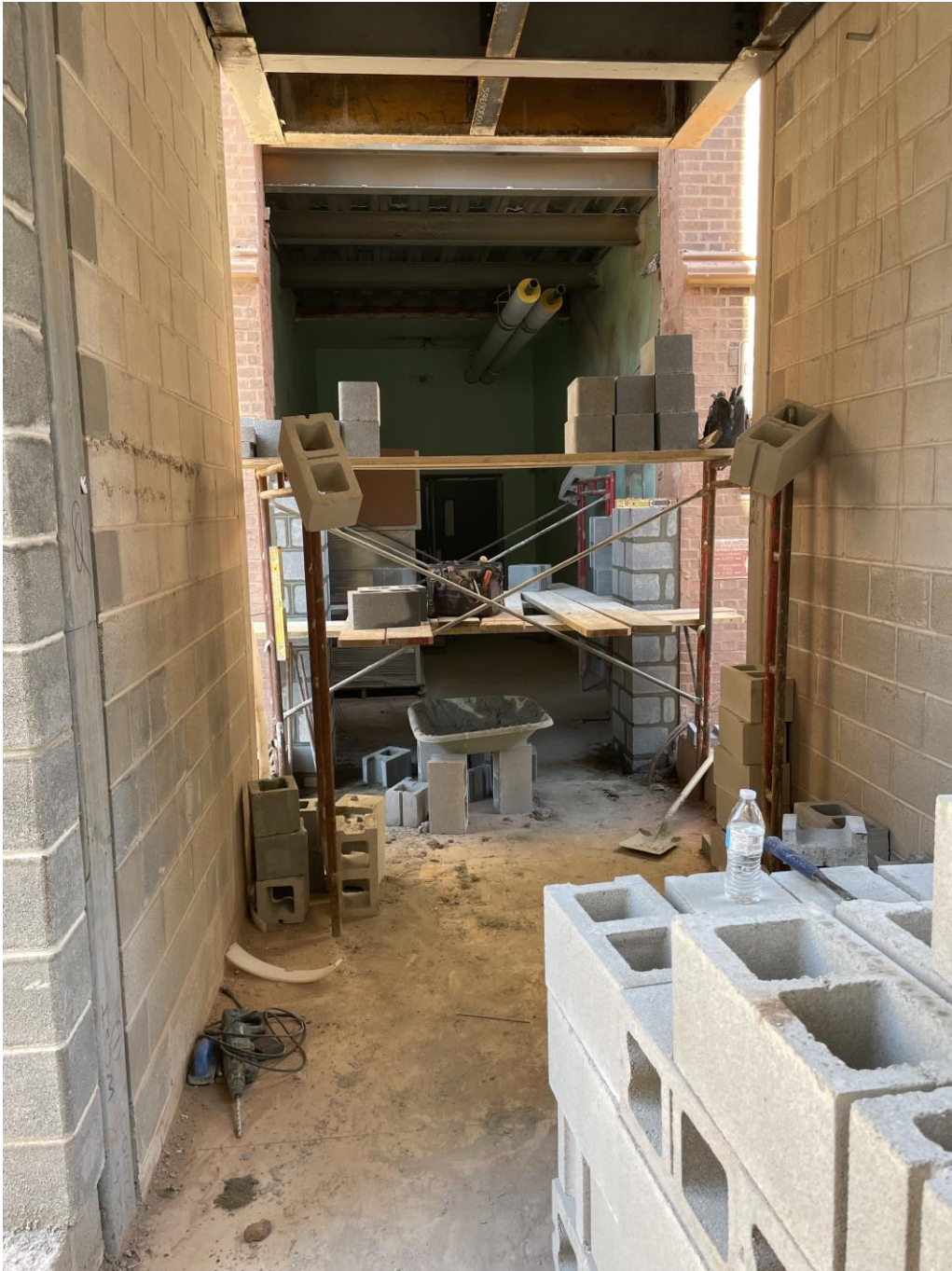
Construction of Fire wall at SME
