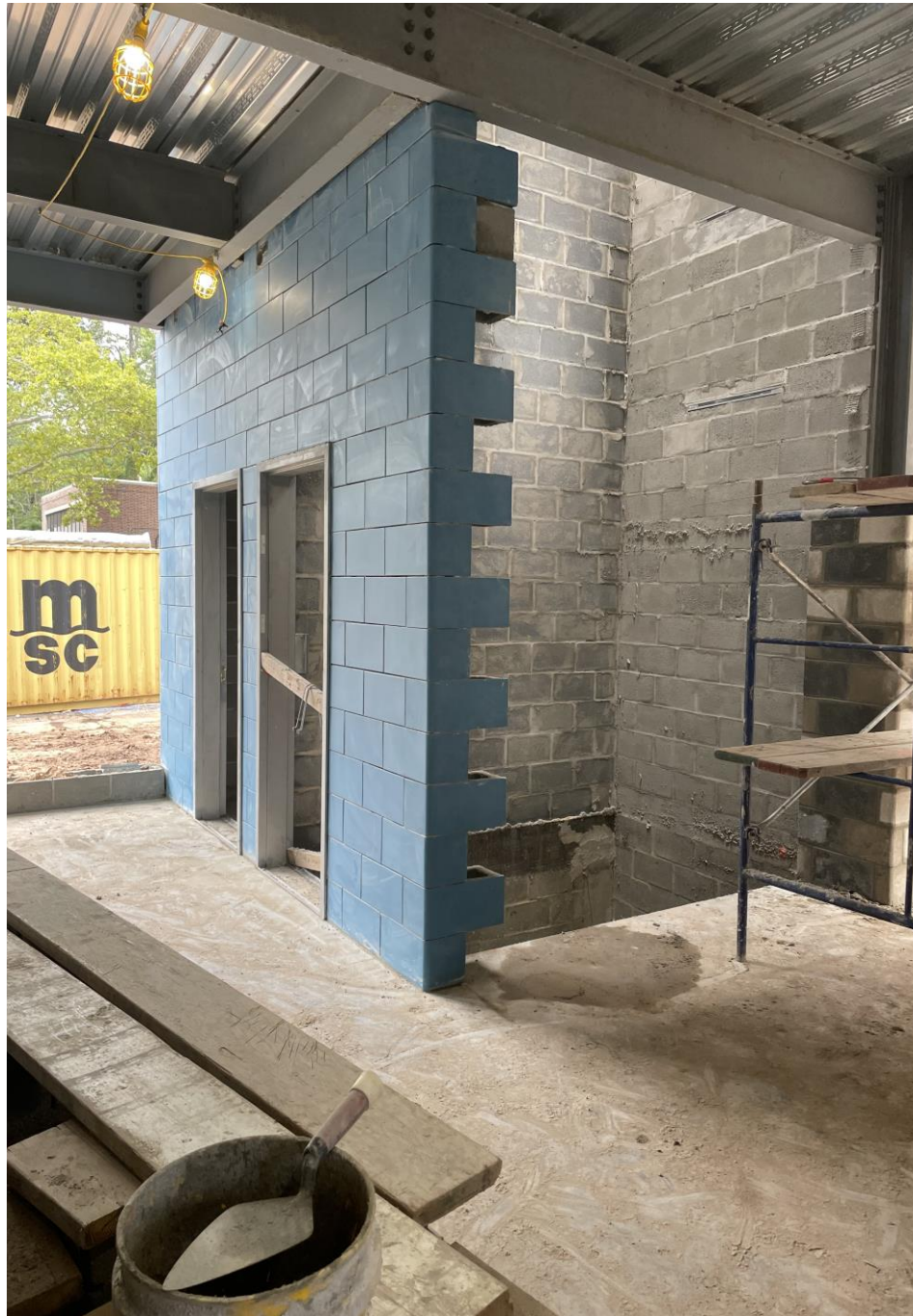
Glazed block at proposed elevator shaft at SME
