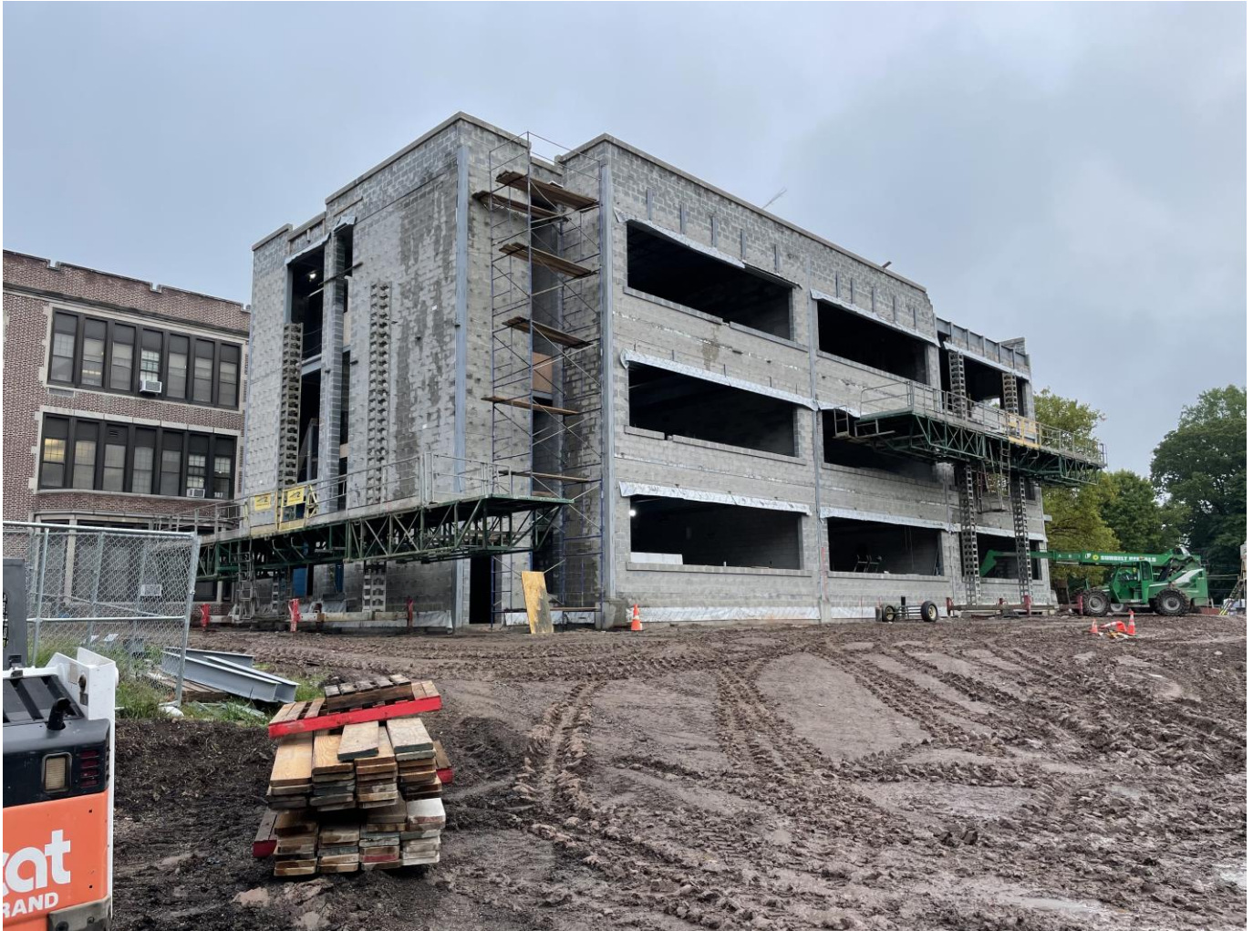
Exterior block work at SME
