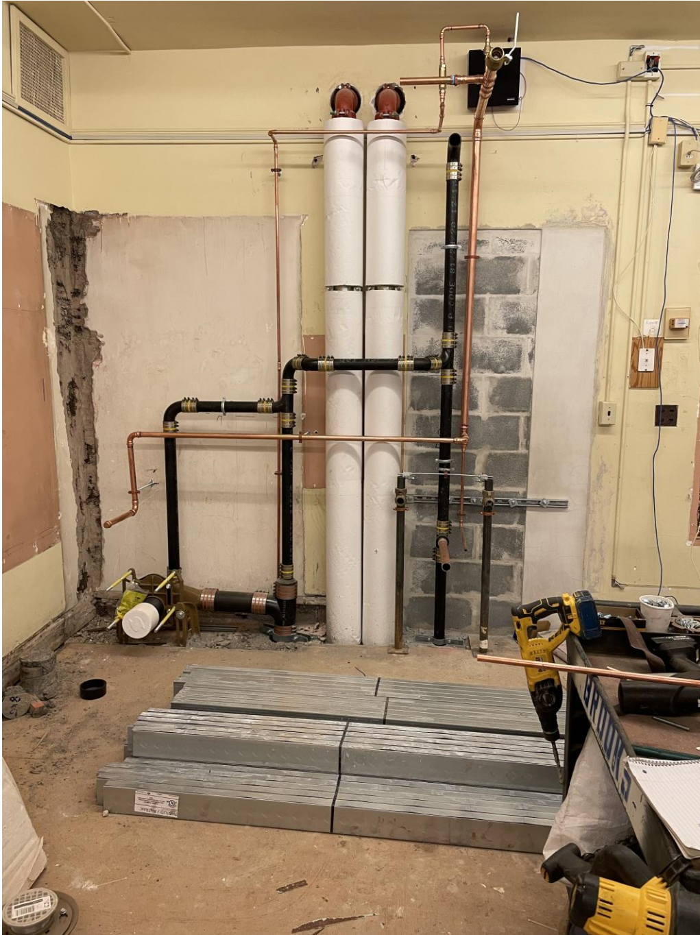
Plumbing rough for proposed office at SME
