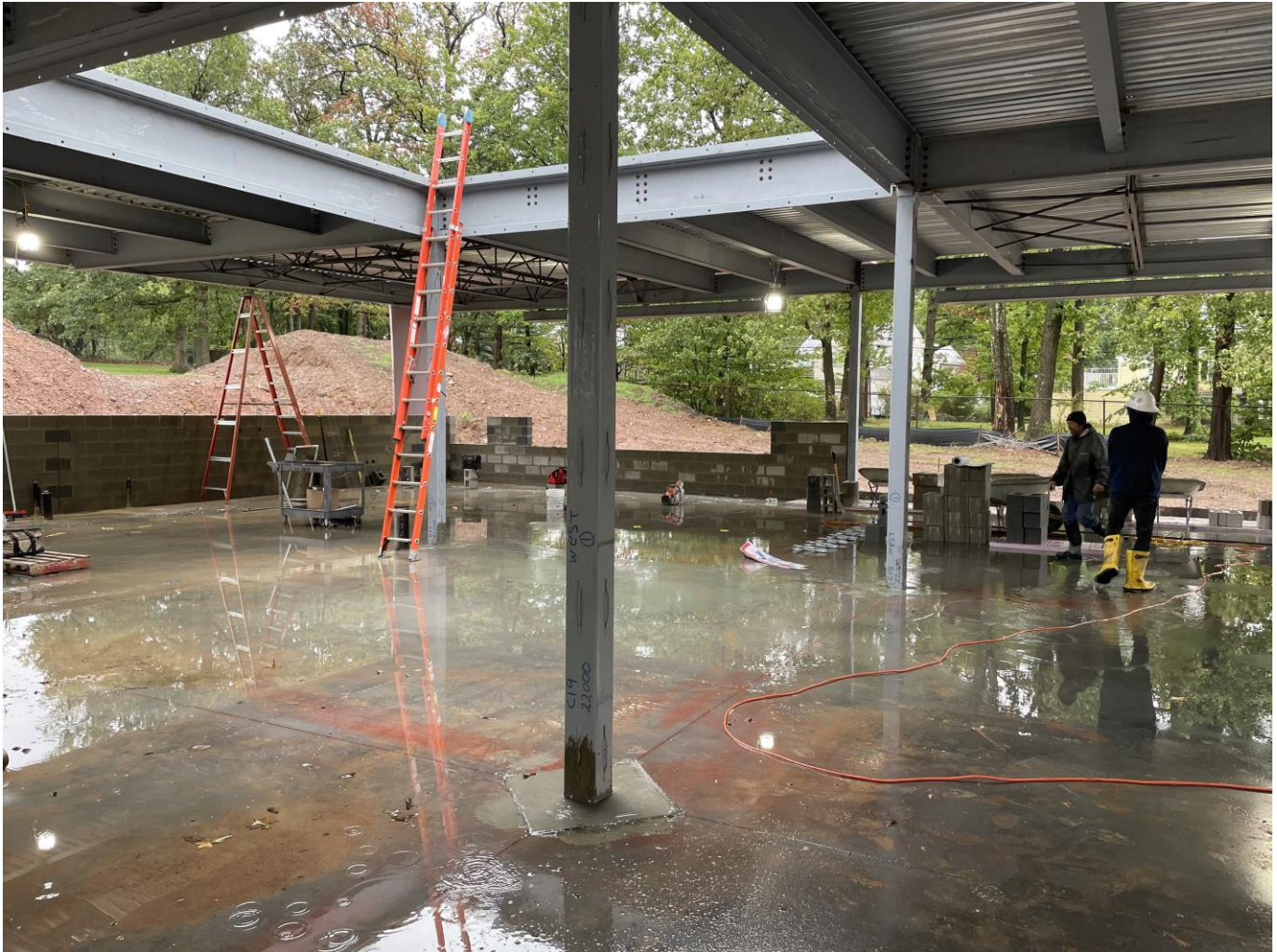
CMU block at SMA for addition
