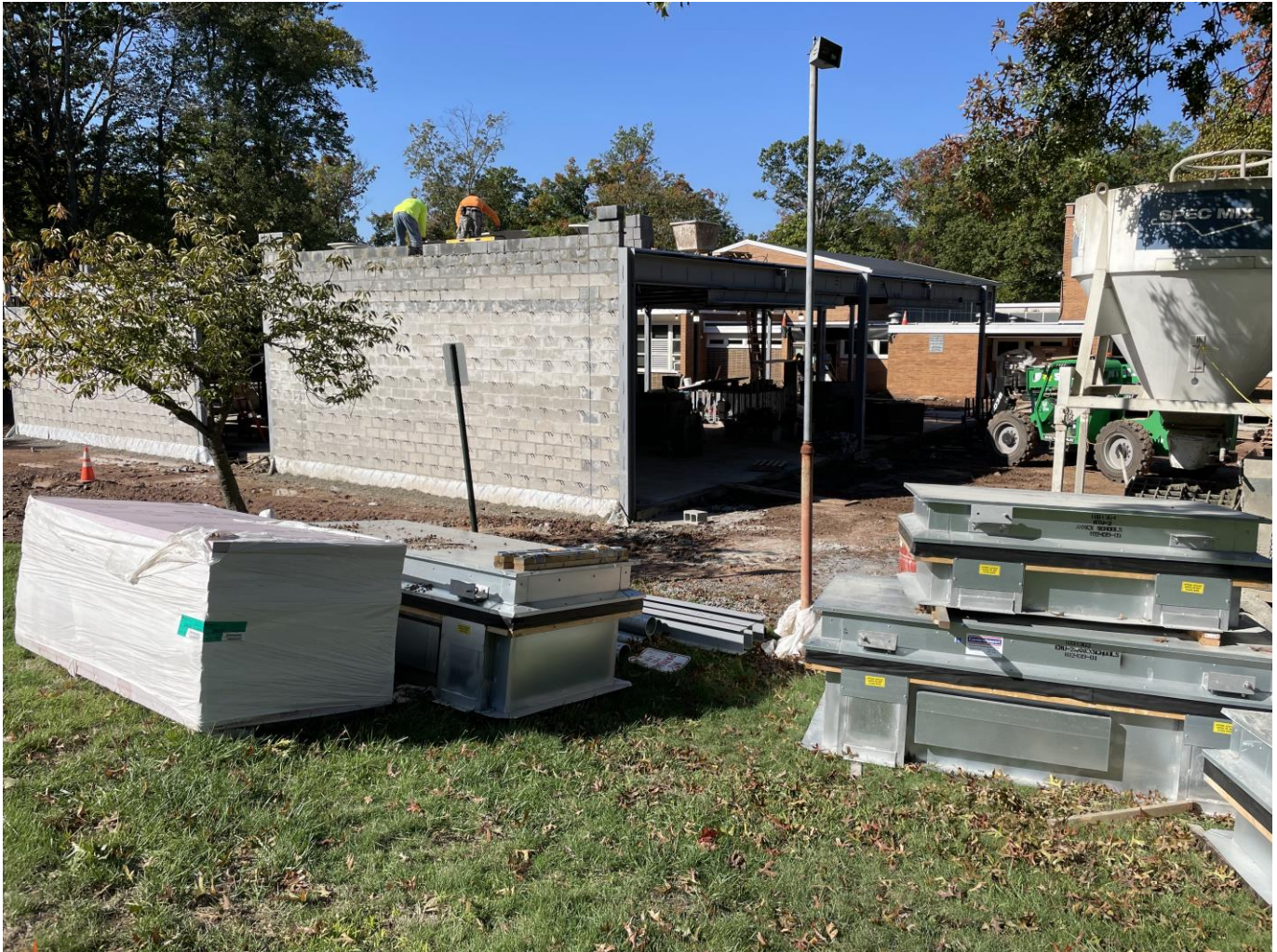
CMU block at SMA for addition
