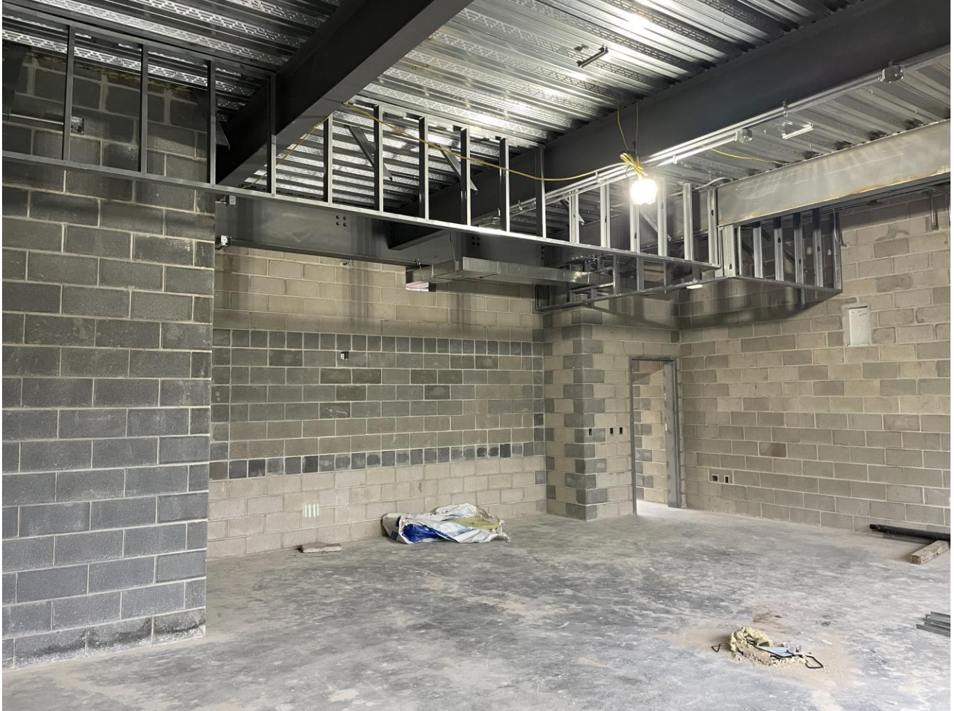
Soffit framing and ductwork at SME
