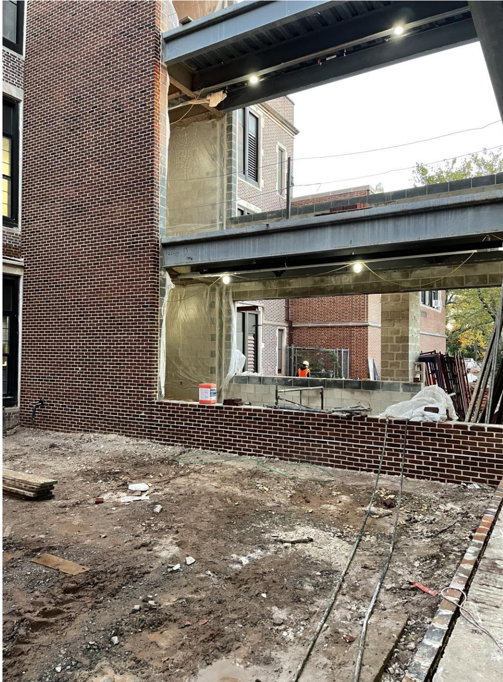
Exterior brickwork at SME
