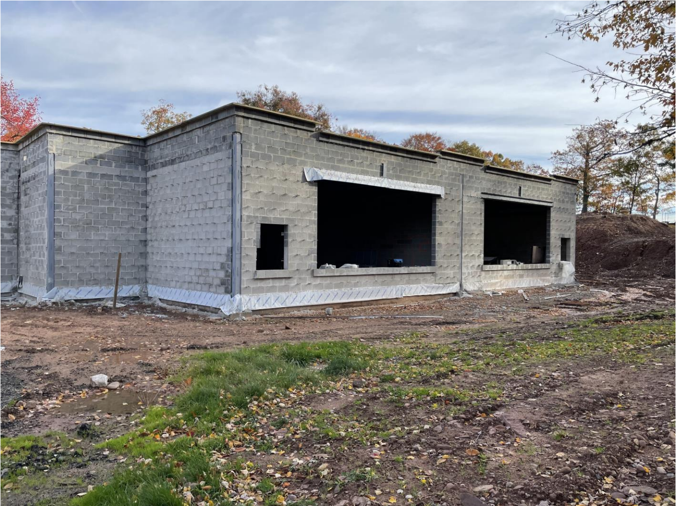
Exterior CMU block at SMA
