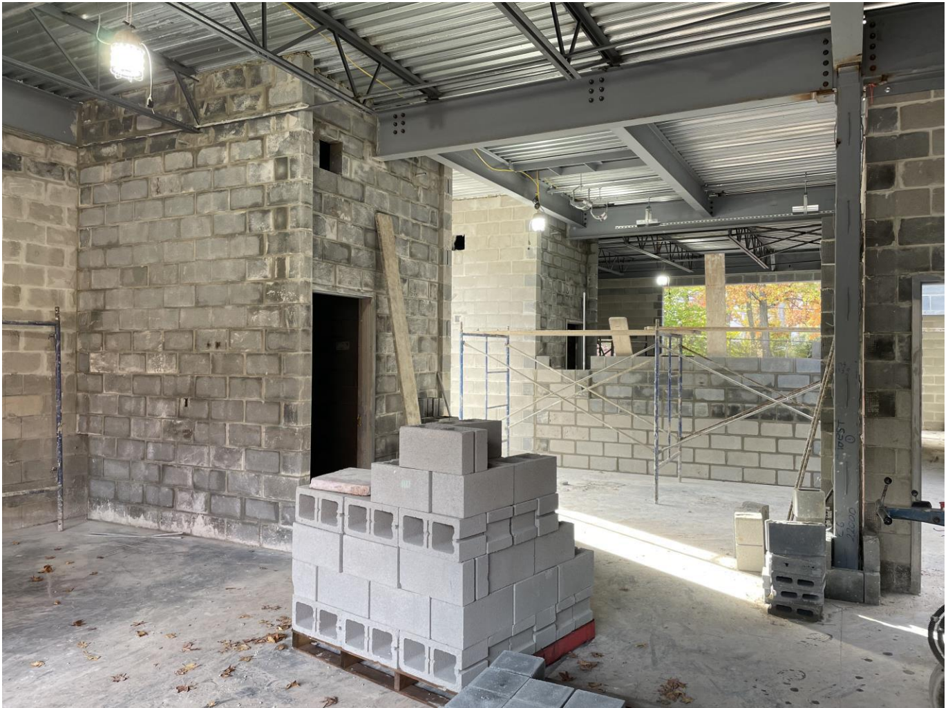
CMU interior block at SMA
