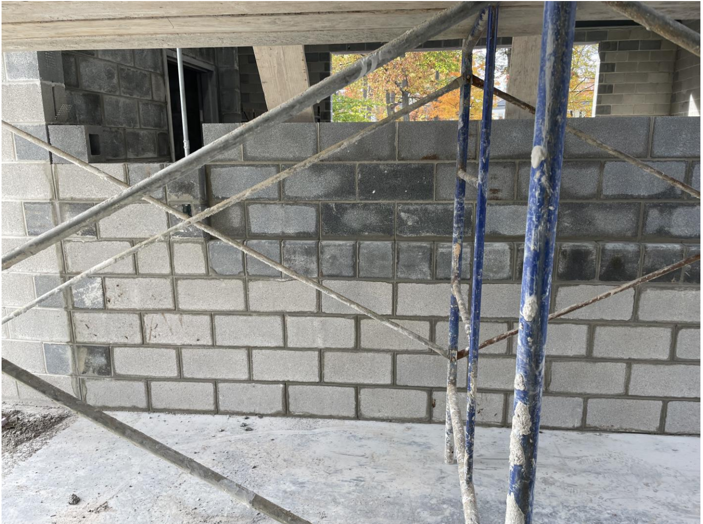
CMU interior block at SMA
