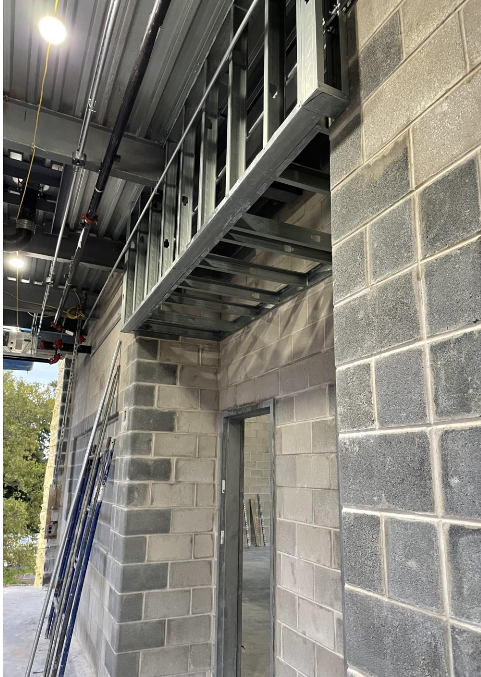
Metal framing for corridor soffits at SME
