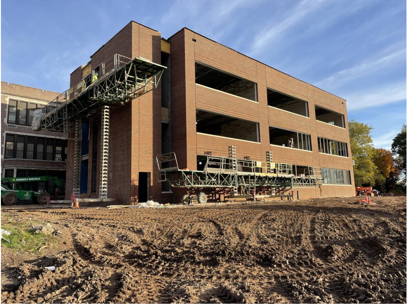
Exterior of addition brickwork at SME
