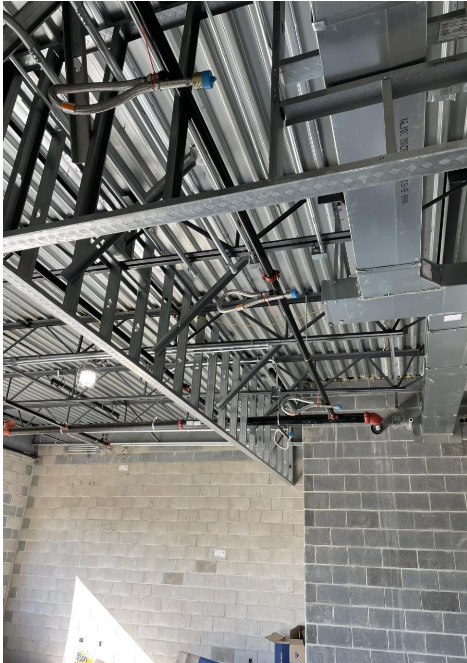
Metal framing for soffits in classrooms at SME
