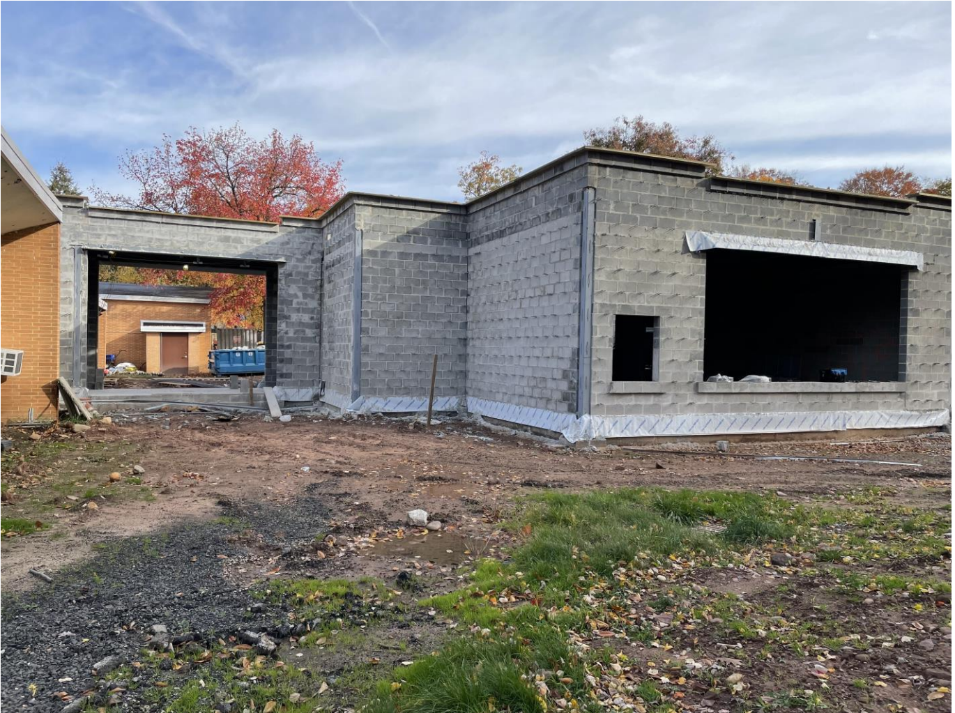
Exterior CMU block at SMA
