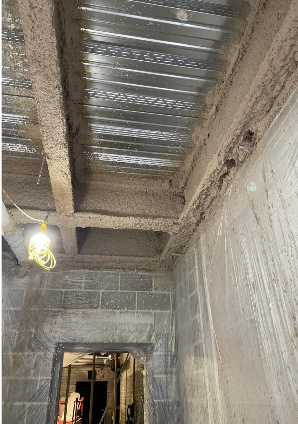
Fireproofing at SME
