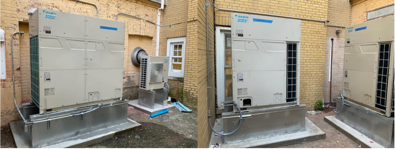
Courtyard Heat Pumps: Conduit runs for wiring underway (not all shown).
