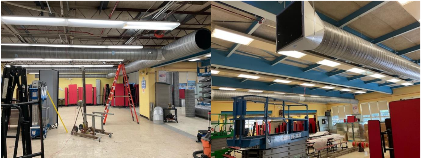
Cafeteria ductwork underway.
