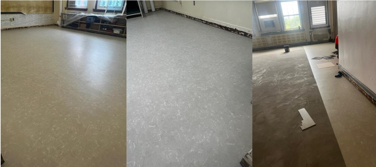
New Floor Tiles- 2 nd Floor Installation Classrooms 288, 287 & underway 295
