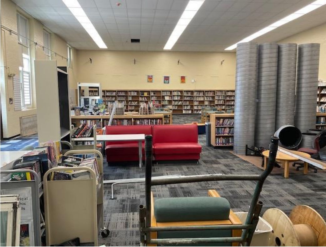
Library: Conduit runs, Duct hangers & Duct staged in space.
