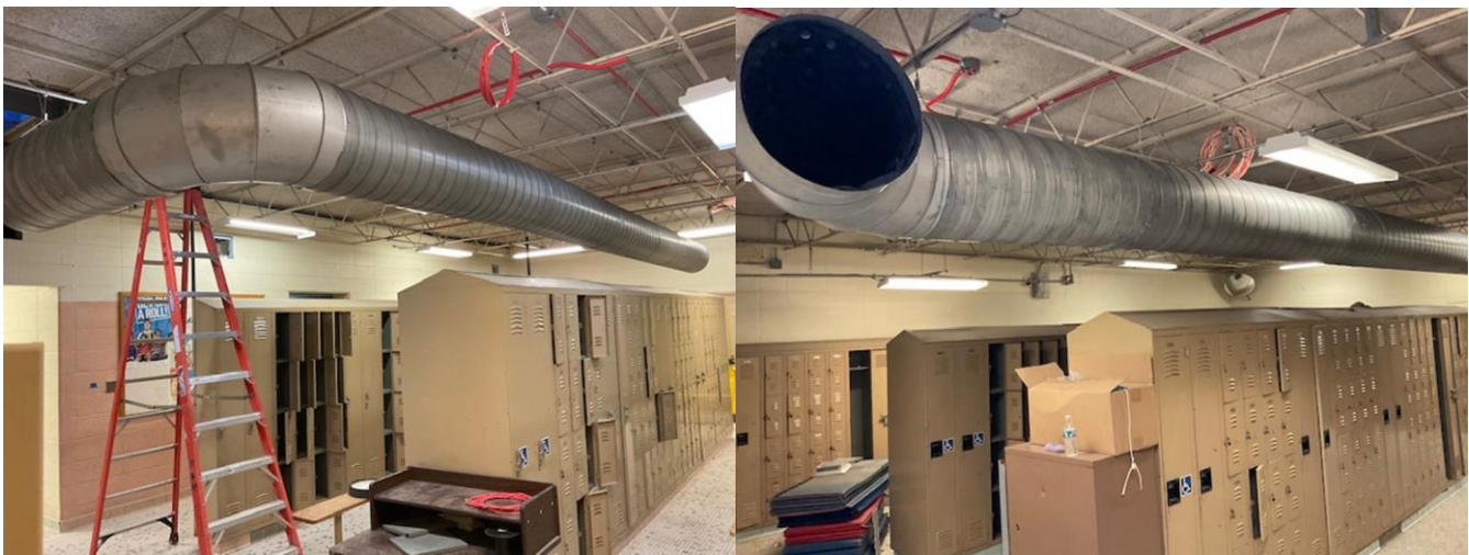
Girls & Boys Locker Rooms- Ductwork underway
