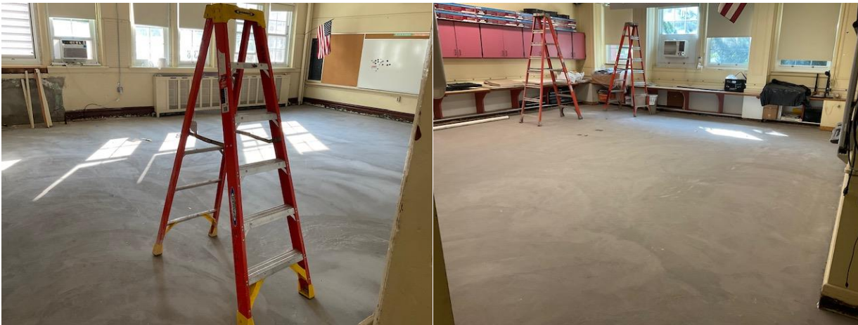
Floors almost ready for tiles- Left CR 138 & Right : CR 20
