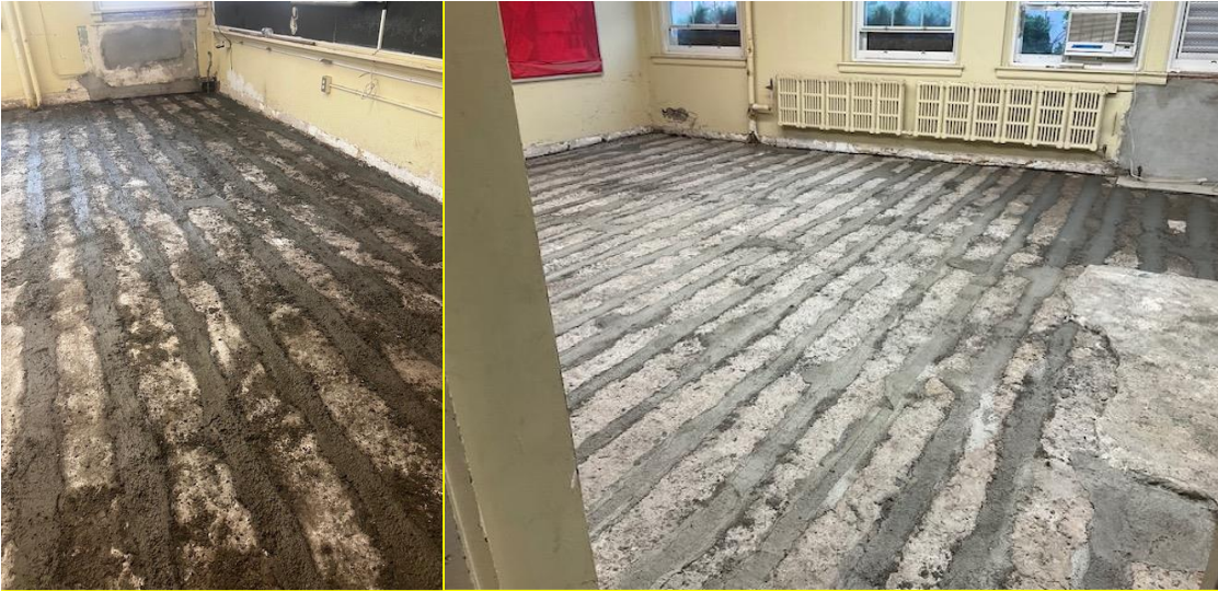
Floors Underway- Left: CR 156 & Right: CR 157
