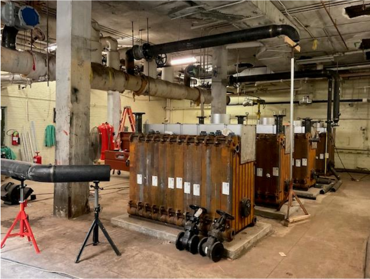
Boiler Room piping & valving installation continues. Estimated @ 35% Complete.
