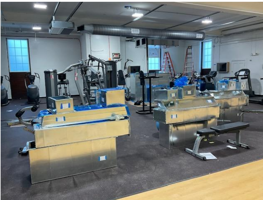
Aux Gym: Connecting ductwork staged.
